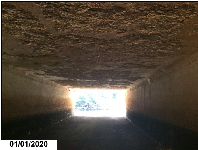
Box Culvert barrel 1 spalls in the Soffit of the top.
