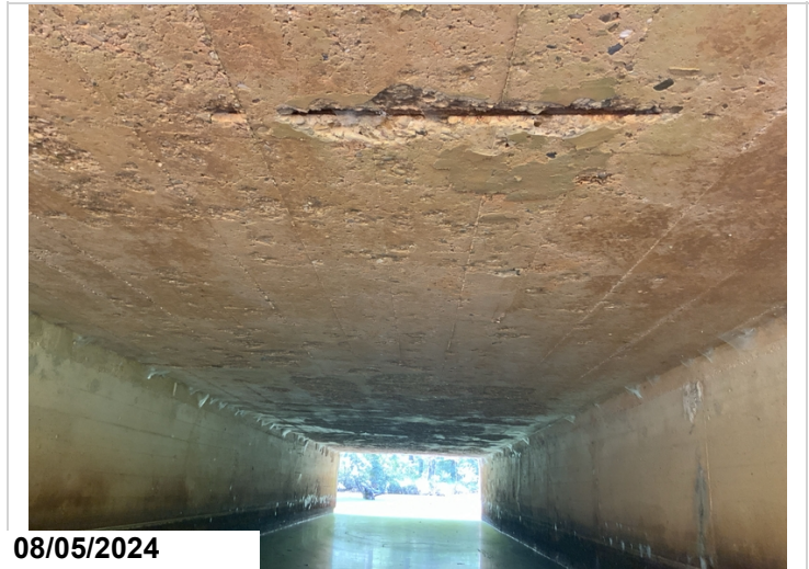
Barrel 1 soffit exposed rebar.
