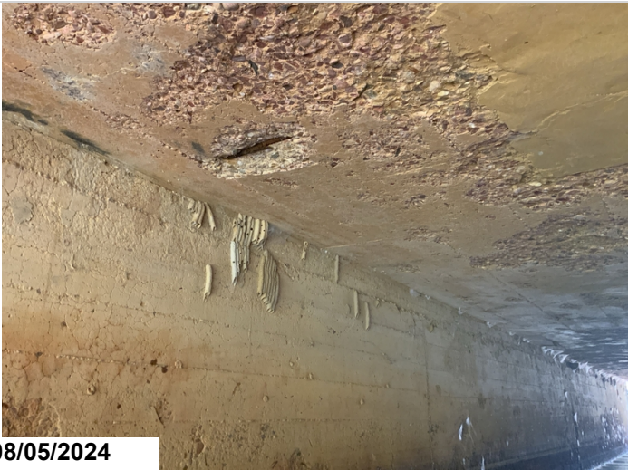
Barrel 2 soffit has exposed rebar.
