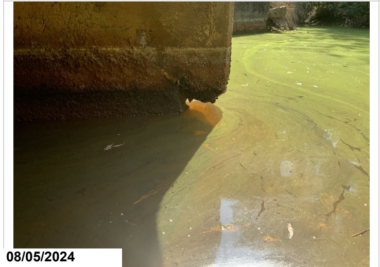
Divider wall outlet end 6" section of severe abrasion.
