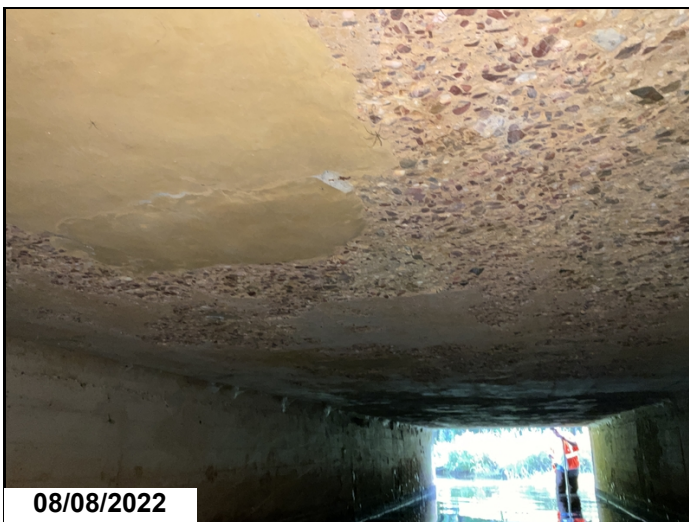
Spalling on the top of the box in barrel 2.
