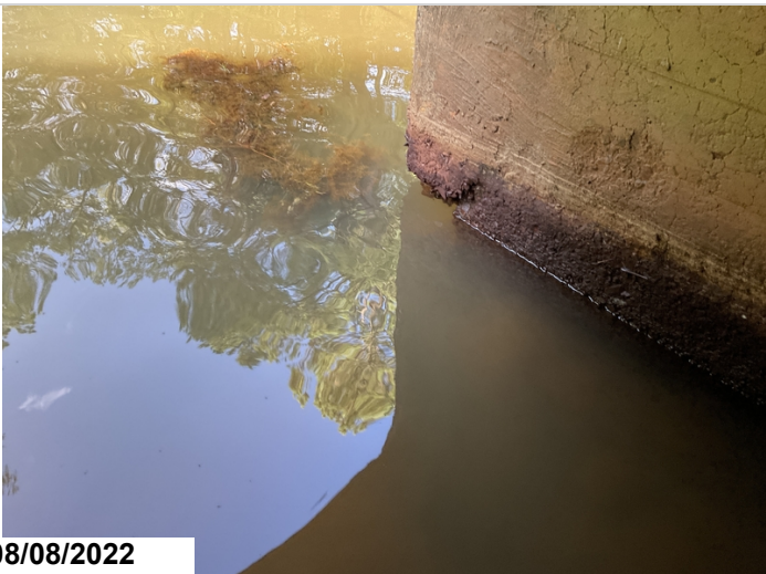
Right end of the center wall, large spall.
