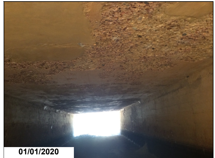
Box Culvert barrel 2, looking from Rt. @ Soffit of box Culvert top has spalls over most of the top. P
