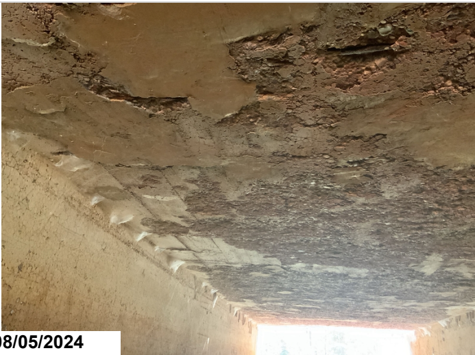
Barrel 1 exposed rebar in soffit
