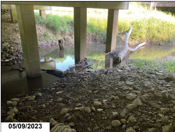
Drift at bent 3
