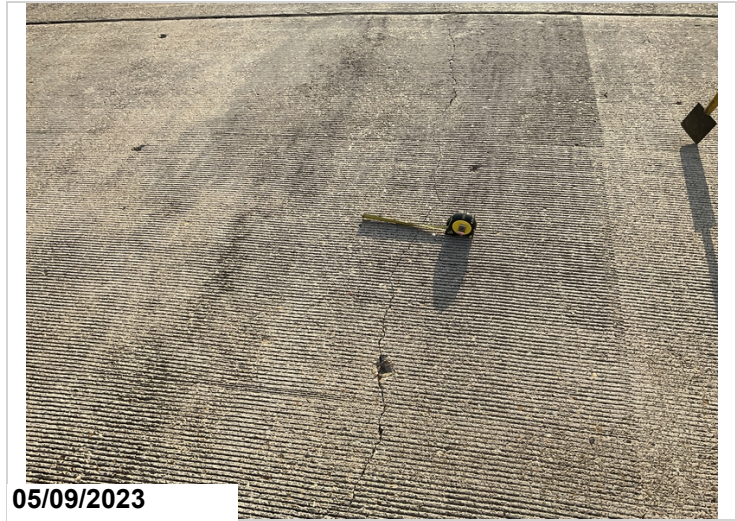
Typical deck cracks upto 0.030".
