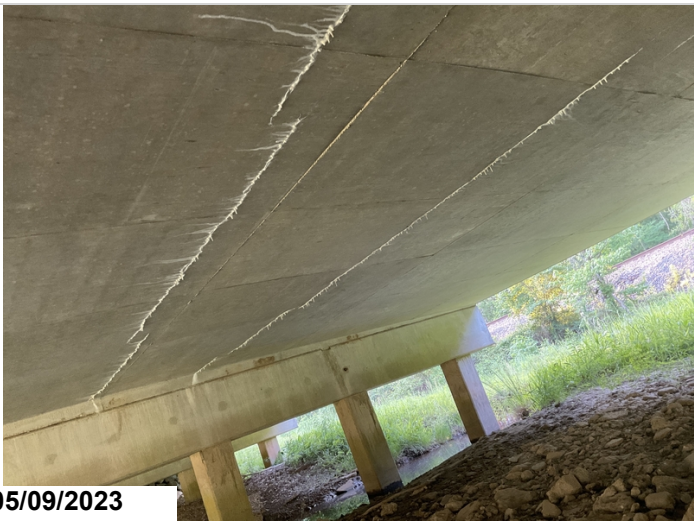
Span 4 efflorescence
