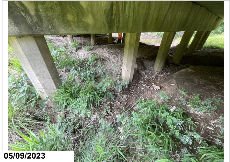
Bent 5, local scour at piles 2- 6.
