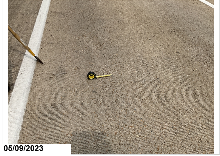
Span 1, map cracking upto 0.025" wide.
