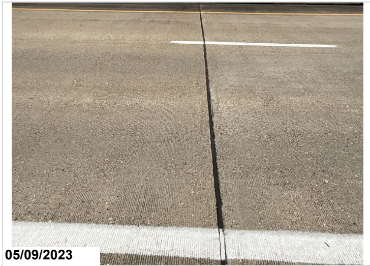
Bent 2, joint seal, debris impaction
