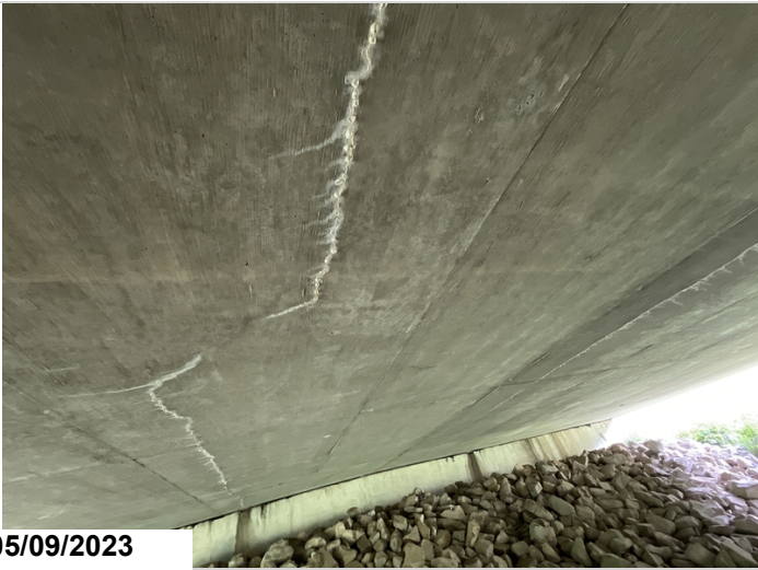
Span 6 efflorescence
