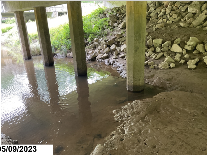
Bent 2, local scour @ piles 3-6
