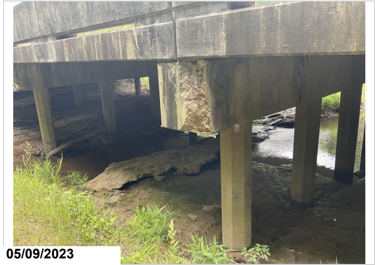
Bent 2, left end of the cap has a spill.
