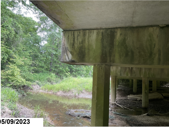
Bent 3, cap left end, vertical cracks 1/4" wide.
