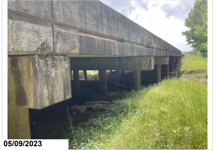
Bent 4, 5, & 6, left end of caps have spalls.
