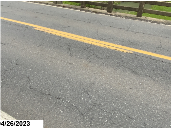
Deck all spans cracks in wearing surface.
