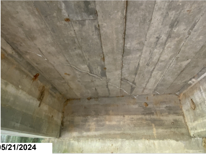
Cracks with efflorescence bay 1.
