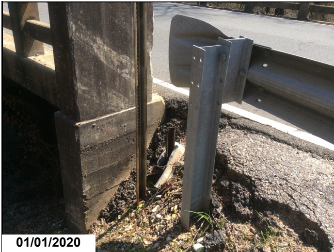
Abutment 1 left side slope erosion.
