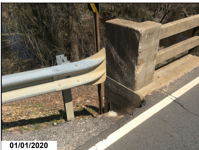
Abutment 1 left showing hole @ edge of traffic path.
