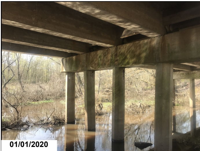
Bent 4 piles 3-5 spalls with exposed rebar
