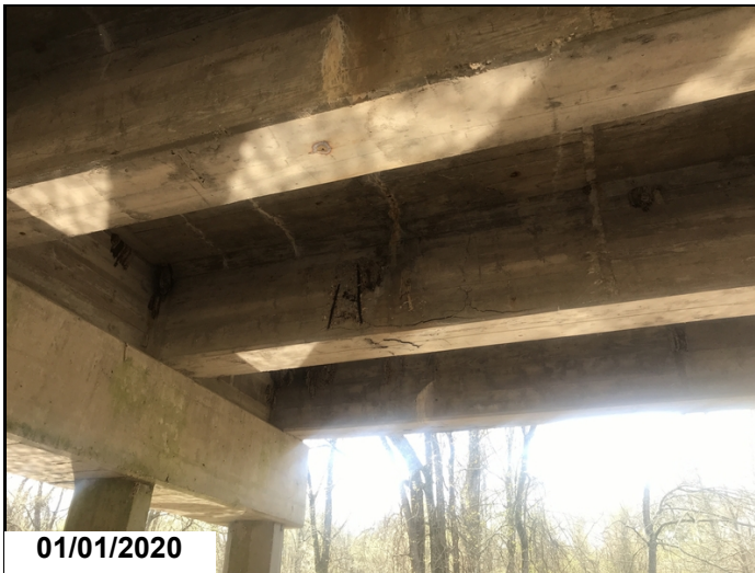
Span 4 girder 4 cracking and spall with exposed rebar
