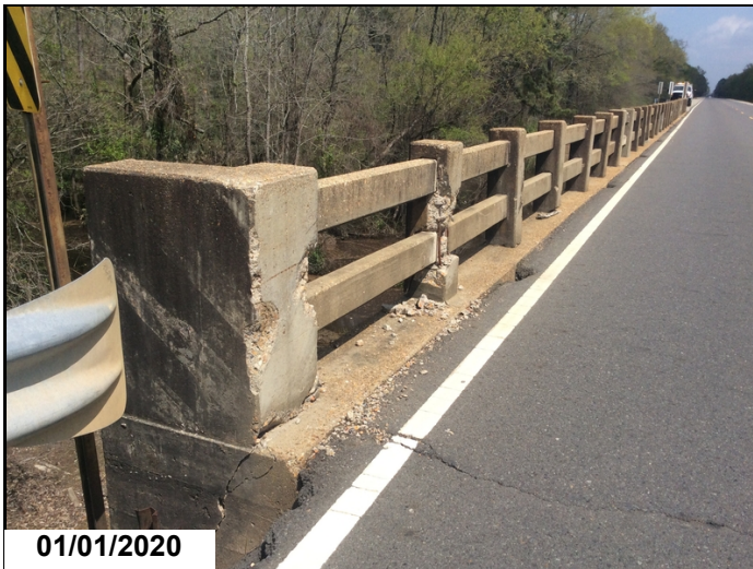
Abutment 1 Lt., BR. end post & 1st 3 guardrail posts have collision damage
