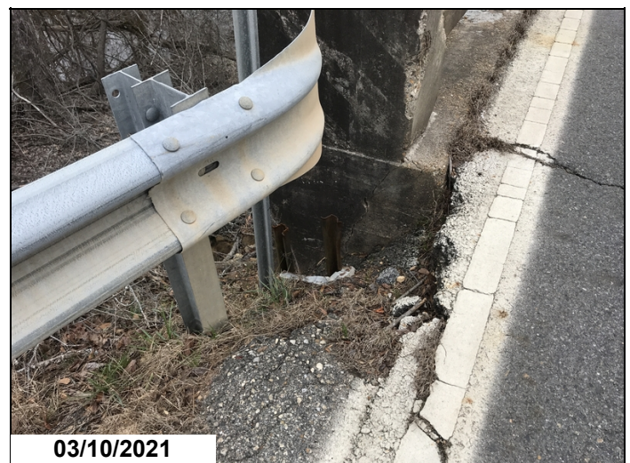
Erosion left side abutment 1
