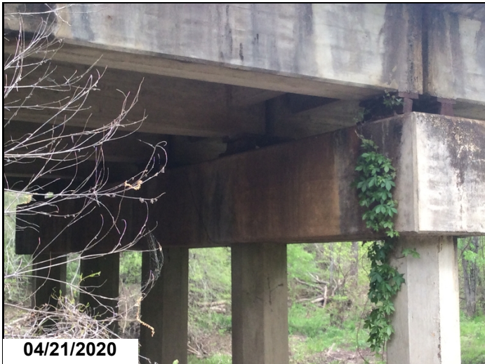
Bt. 2 looking Rt., bearings are rocked ahead & have rust on them.
