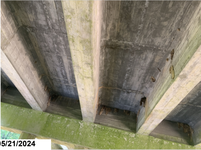
Span 4 has efflorescence.
