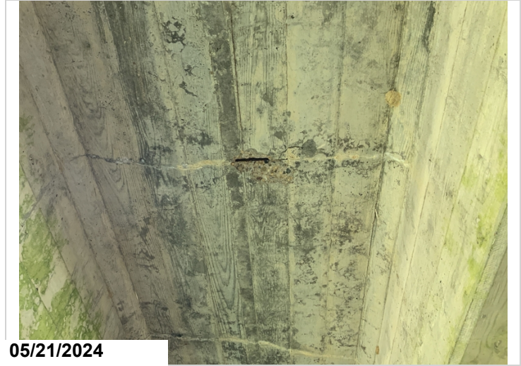
Span 13 bay 1 exposed rebar
