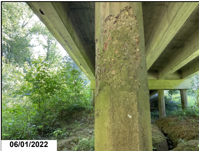
Bent 13 pile 2 spalled
