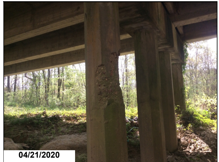
Bent 13 Pile 2 spalled
