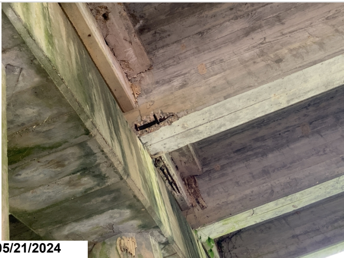
Bent 13 span 12 girder 3 exposed steel.
