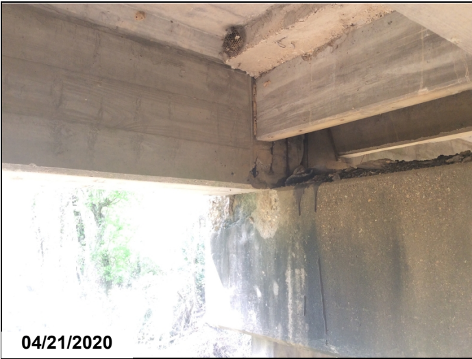
Bent 7, girder 1 ahead, has spall on girder end at bearing area. Also cap Rt. End ahead side has spall with exposed steel.
