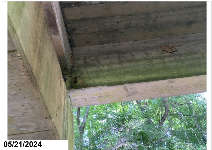
Span 5 girder 1 has exposed rebar.
