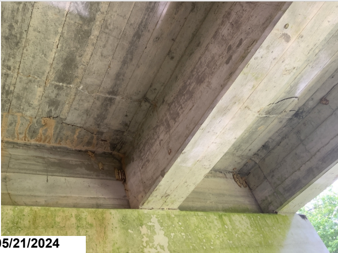
Span 11 under surface has delams.
