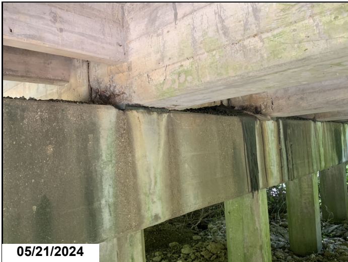
Girders 2&3 at bent 7 spall with exposed steel at bearing areas.
