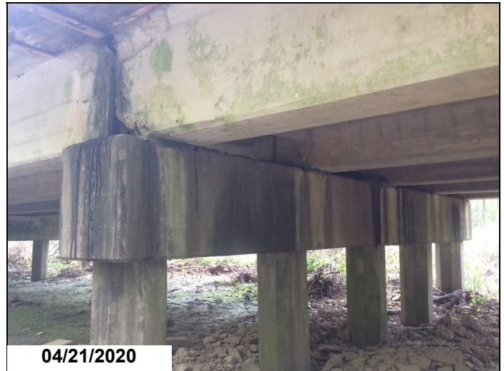
Bent 7 back, girder 1 @ bearing area has spall with exposed steel. Section loss to girder end. Also girder 2 has delamn. on Lt. side & girder 3 has spall over bearing area.
