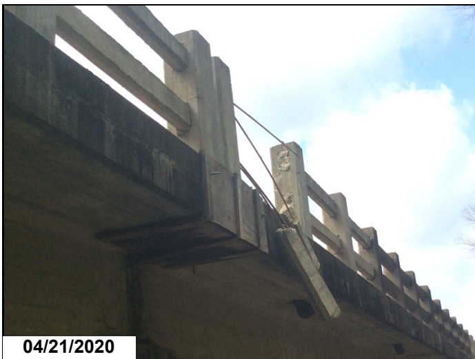
Span 9, Lt. side concrete rail @ Bt. 10 have collision damage.
