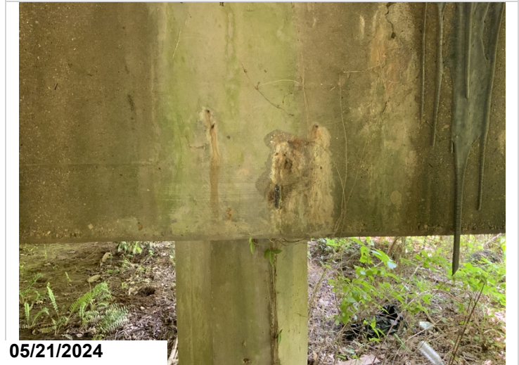
Bent 10 cap back has spall.
