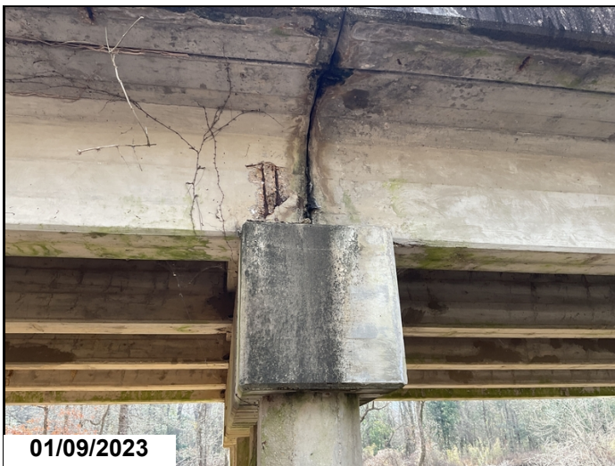
Span 5 girder 1, spall with exposed rebar.
