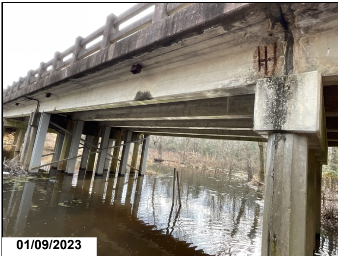
Span 2, girder 1, exposed rebar on both ends.
