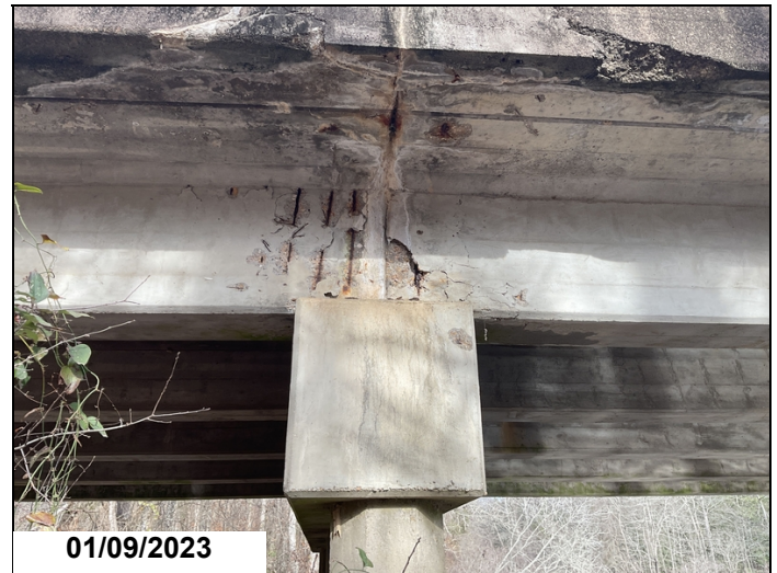
Span 1 & 2, girder 5, @ Bt. 2, spalls with exposed rebar.
