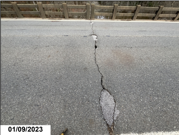
Bent 3, joint between spans 2 & 3 there are holes in the overlay and joint.
