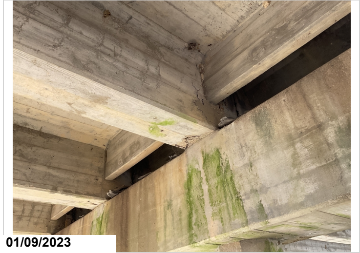
Span 5 girder 2. Spall with exposed rebar.
