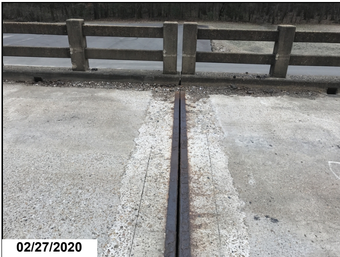
Joint @ bent 3 looking from Lt. to Rt. Concrete on Rt. side from curb back Lt. Both sides of joint has spalled out for about 5' & approx. 2" deep.
