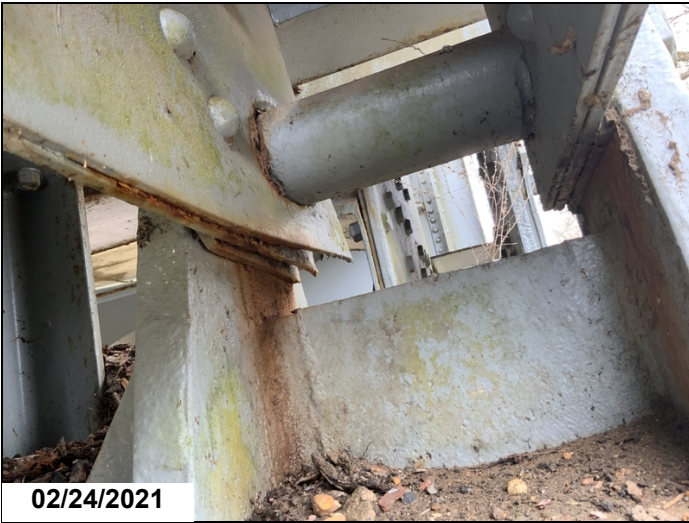
Left side truss 2, L0 pin has section loss
