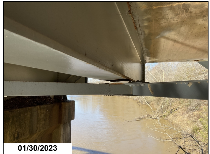
T3, FB 2, lateral brace, bolt missing in connection.
