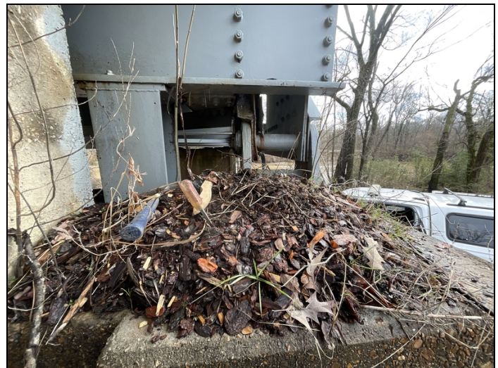
Bent 11, debris built up around the bearings.
