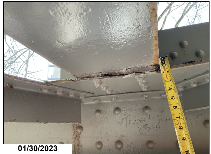
T1 L4 Rt. 3/8" section loss lower flange of floor beam.
