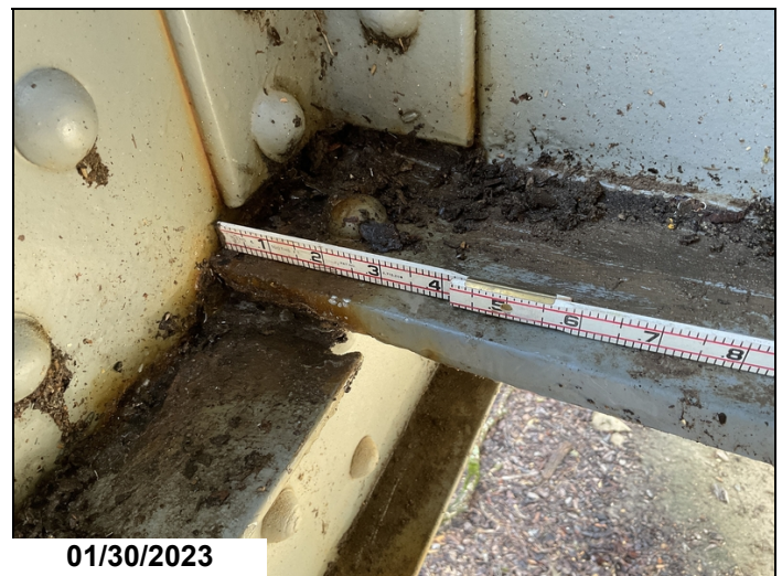
T1 L2 Lt., back side. 0.5" hole in top flange of lower cord.
