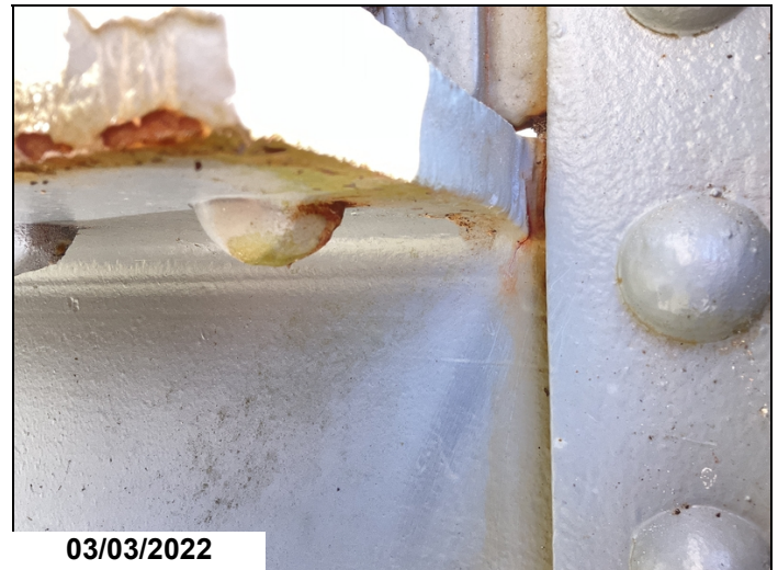
Truss 2 at L10 crack in FB
