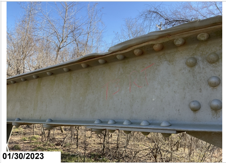
Top flange damage between U7 & U8.
