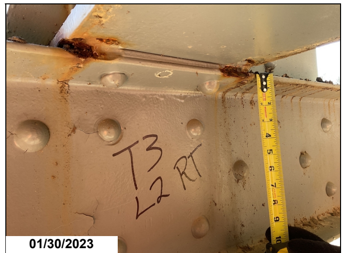
T3 L2 Rt. Pitting upto 1/4" deep, bottom flange of FB, Top flange of chord.
