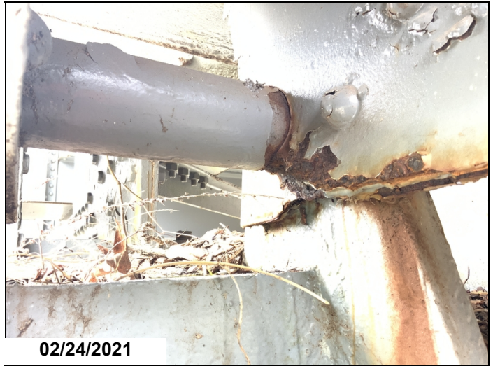
Truss 3 right side, RL0 at pin connection plate with section loss
