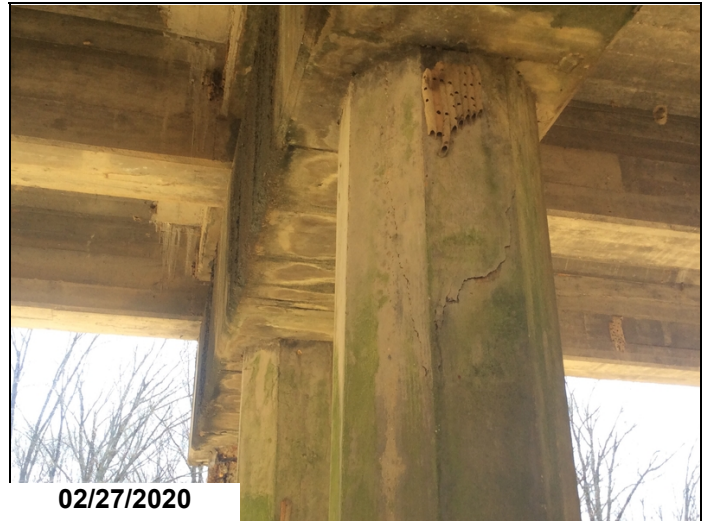
Bent 3, Pile 3 has 1 1/2' of delamination @ top of pile & bottom of cap.
