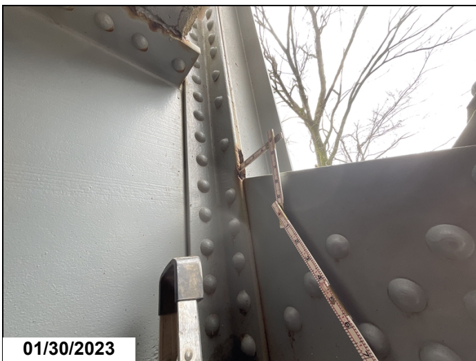
T1 L3 Rt. Pack rust at connection plates.
