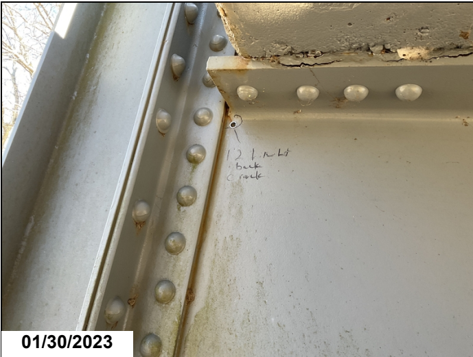
T2 L10 Lt. Crack repaired, hole drilled & arrester installed.
