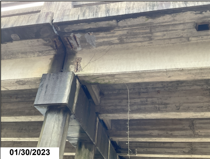
Span 6 @ Bent 7, spall with exposed rebar.
