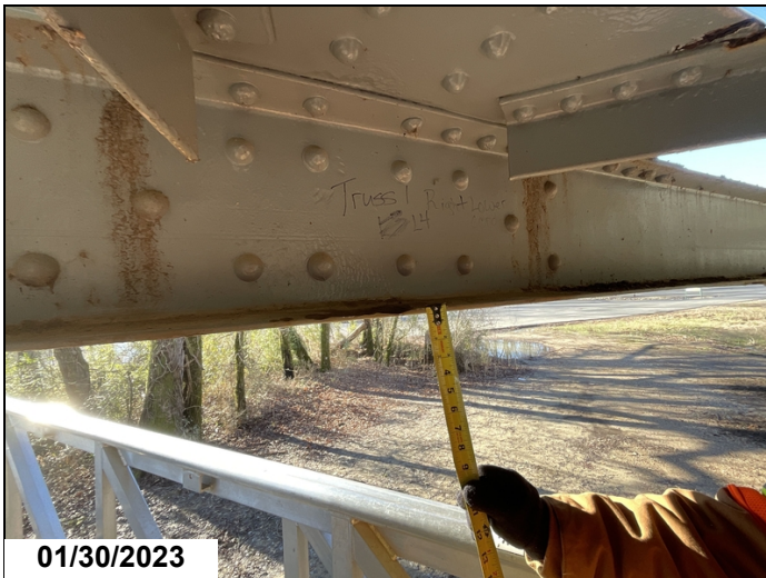
T1 L4 Rt. Inside C-channel of lower chord. Bottom flange of inside cord down to knife edge.
