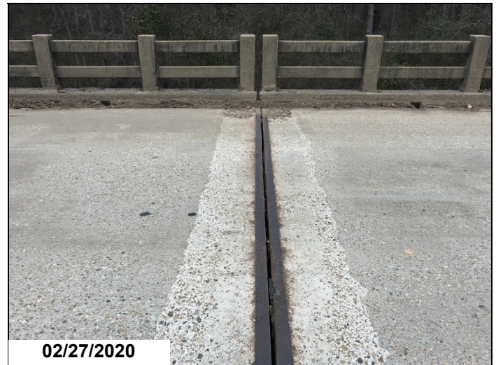
Bent 9 looking from Rt. to Lt. @ joint. Concrete on Lt. Side of the bridge, both sides of the joint have spalled out for about 2' & approx. 1 1/2" deep.
