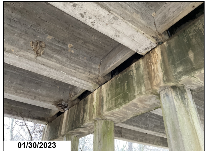
Span 24, @ Bent 24, Girders 2- 4 have spalls with exposed rebar.
