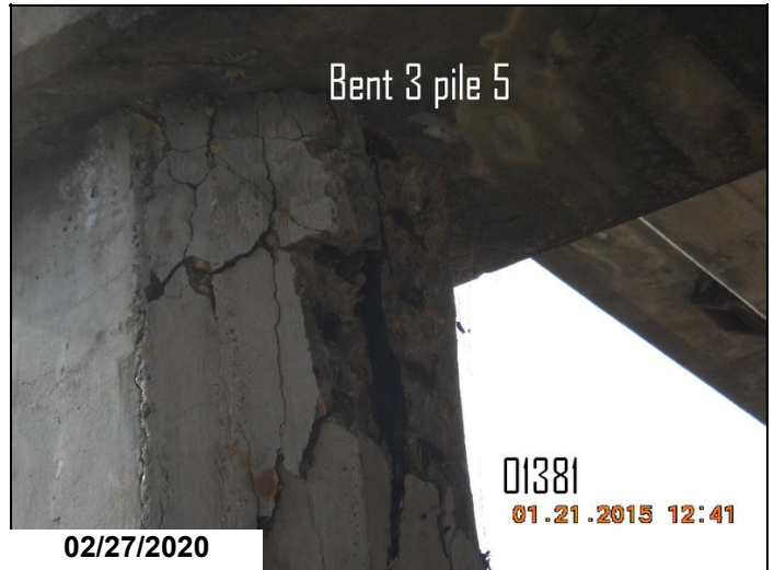
Bent 3 pile 5 has spall and delamination with exposed steel.
