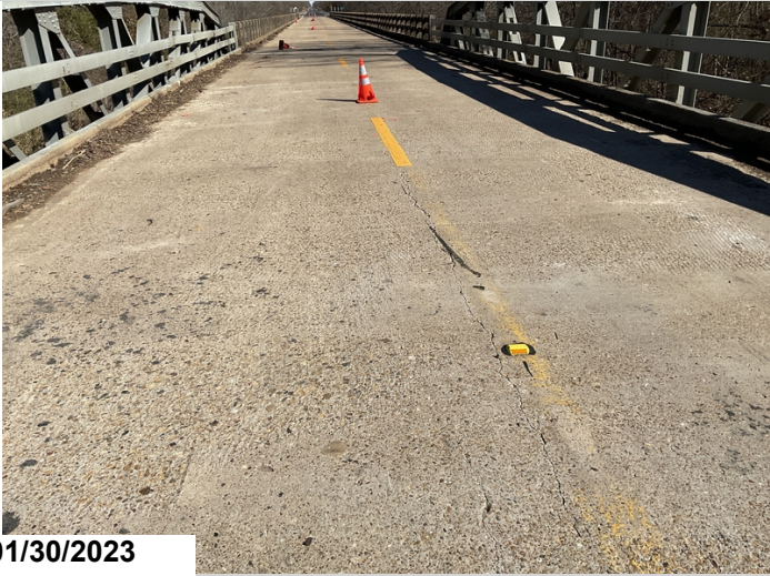
Deck cracks span 13
