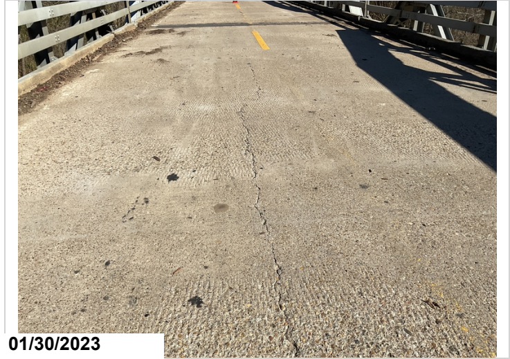
Cracks in deck span 12
