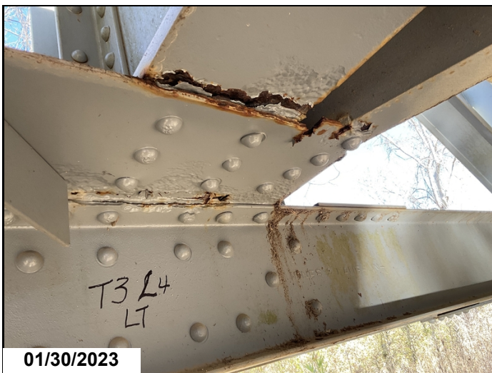
T3 L4 Lt., Corrosion hole in gusset plate, pitting in the bottom web of the FB upto, 3/8" deep.
