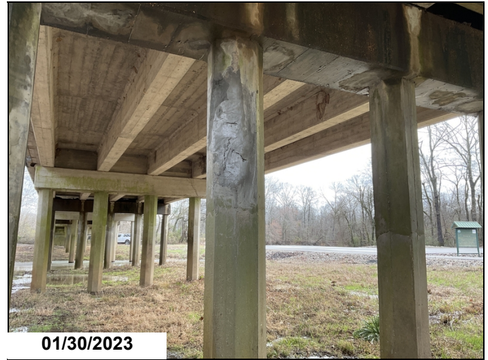
Bent 5, pile 2 has been repaired.
