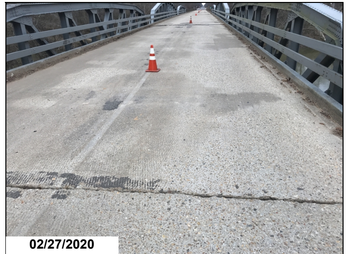
Truss #1 deck, joint is rough.
