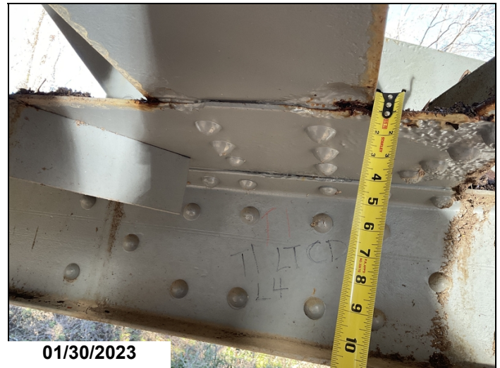
T1 L4 Lt. 3/8" section loss lower flange of floor beam.
