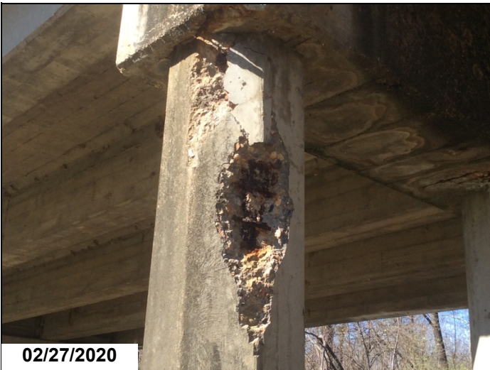
Bent 5, pile 5 has 2 1/2' of spall & delam with exposed steel.
