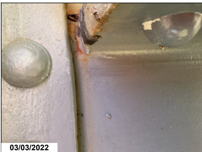
Truss 3 at L1 crack in FB
