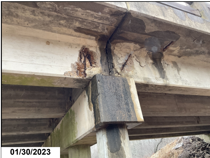
Span 26 & 27, Girder 5, exposed rebar.
