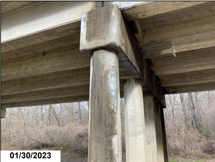
Bent 5, pile 5 has been repaired.
