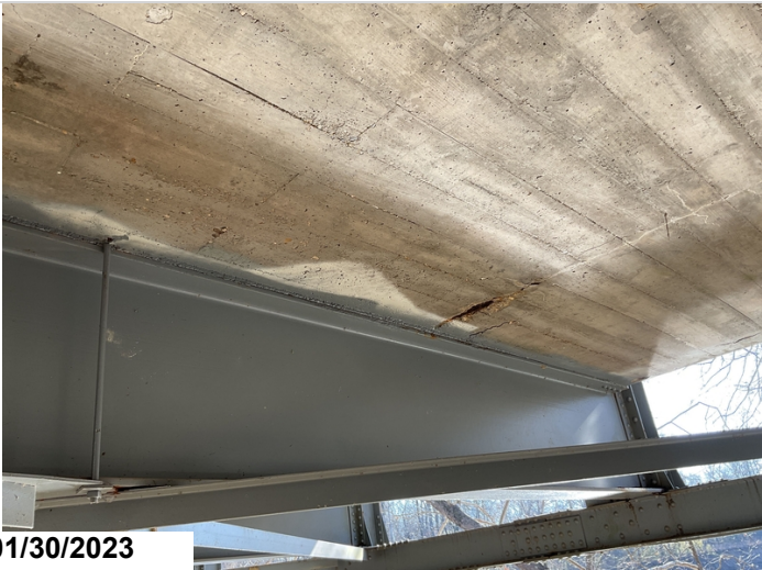
Truss 1, exposed rebar in deck.
