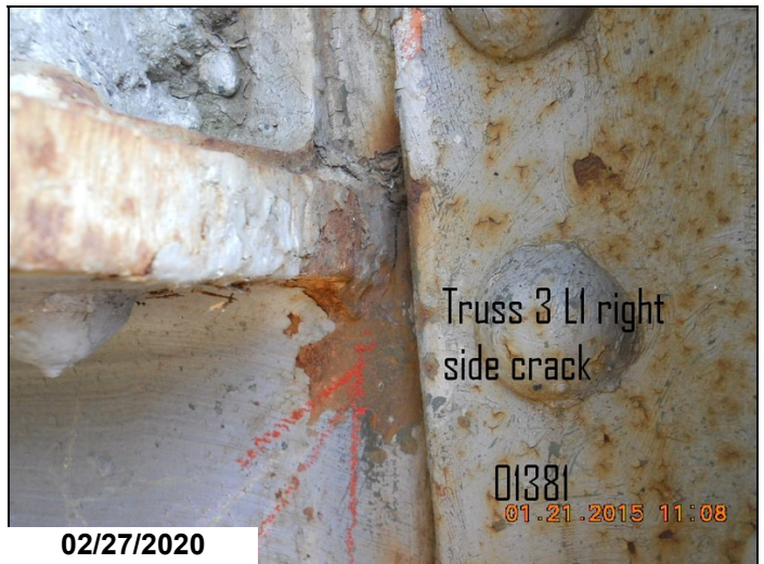
Truss 3, L1 Rt., crack in web of FB.
