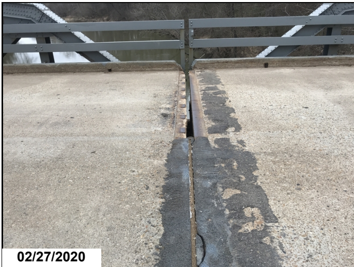
Joint between T2 & T3 Lt. side looking from Rt. to Lt., gap is 3 1/2" wide between road irons.
