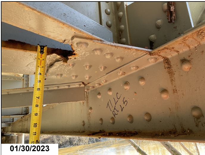
T1 L5 Rt. 3/8" section loss lower flange of floor beam.
