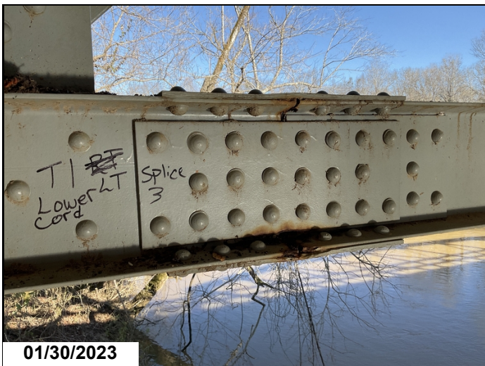
T1 Lower chord, splice 3. All splice plates have pack rust.
