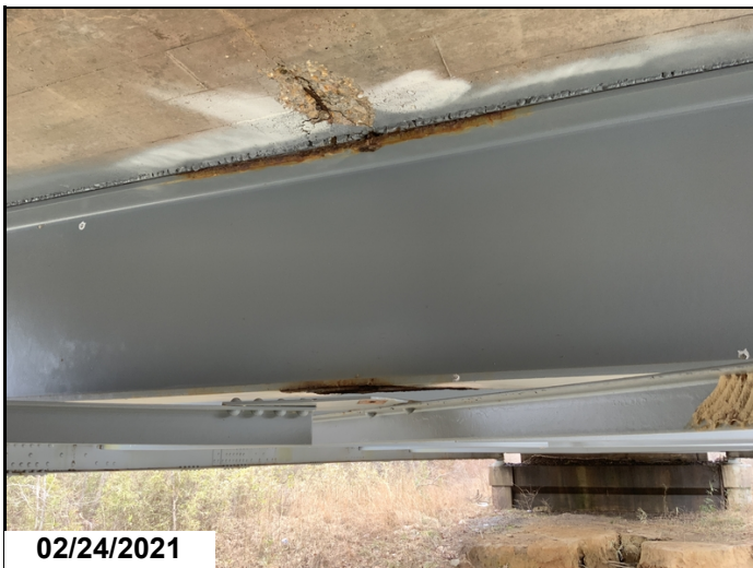
Truss 3 fb 2, cross bracing connection bolts missing
