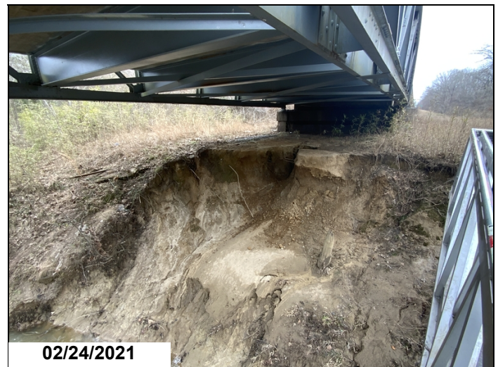
Bank erosion span 13
