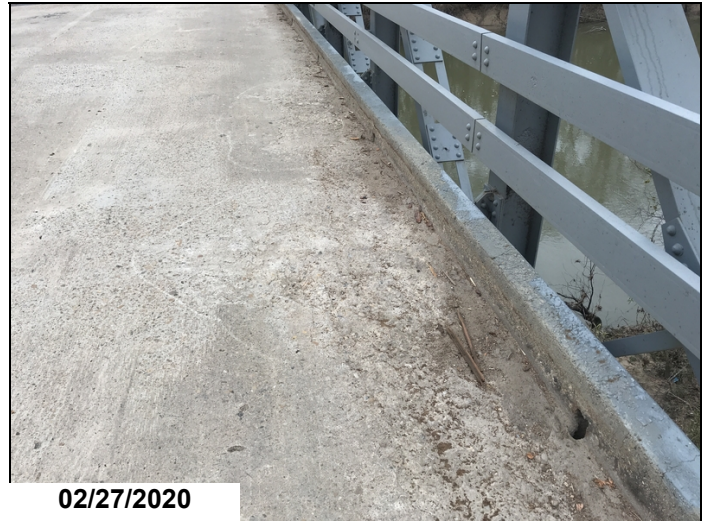
T3 @ midspan from L3 - L5 Lt. in the gutter line is spalled approx. 1" deep.
