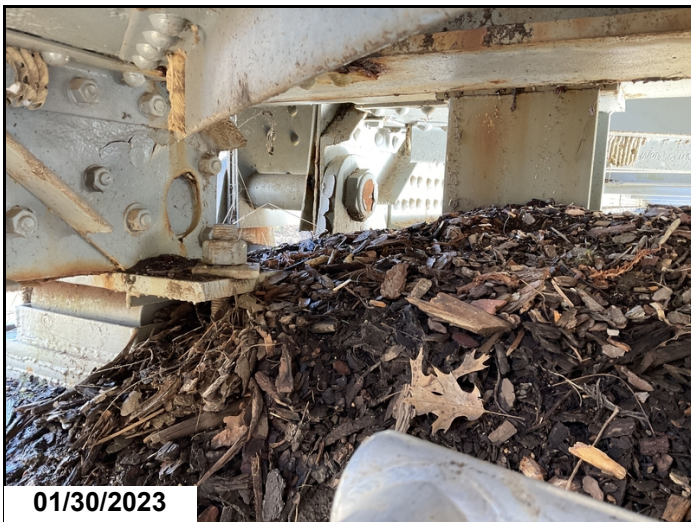
T2, L0, Left, pack rust at gusset plates.
