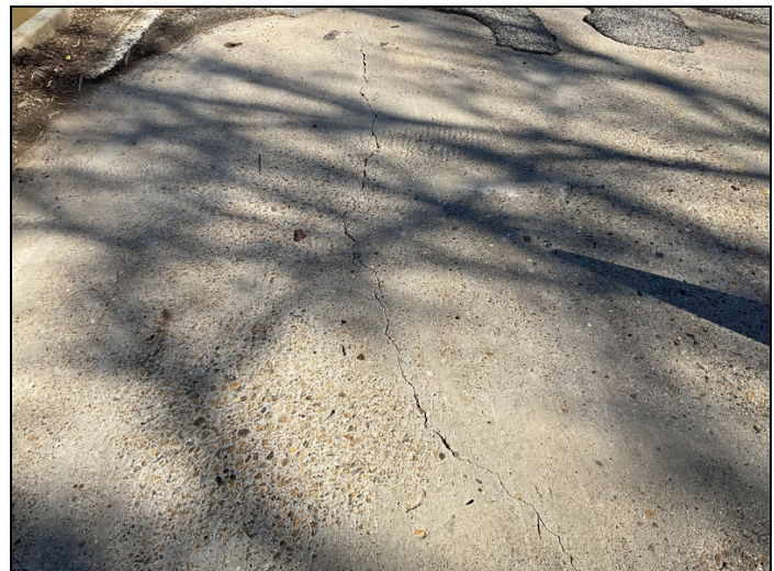
Crack in deck span 11
