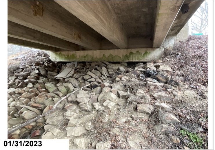
Bent 28 abutment, embankment has settled below the cap.
