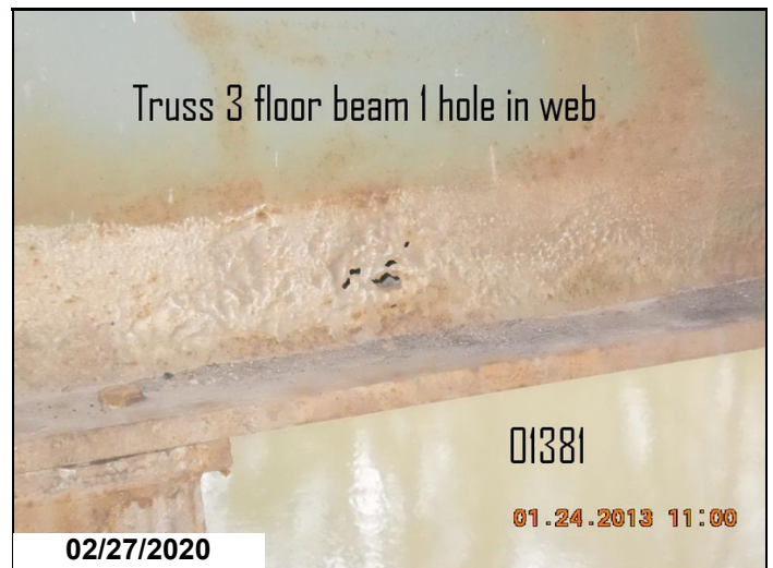
Truss 3, hole in FB.
