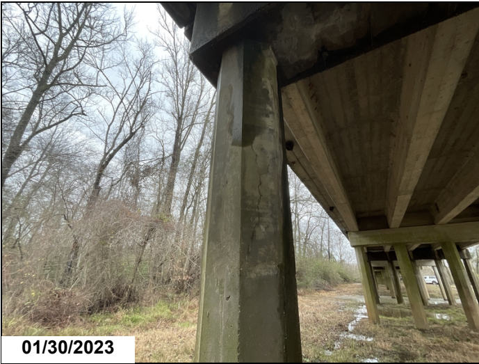
Bent 5 pile 1, vertical crack upto .030"
