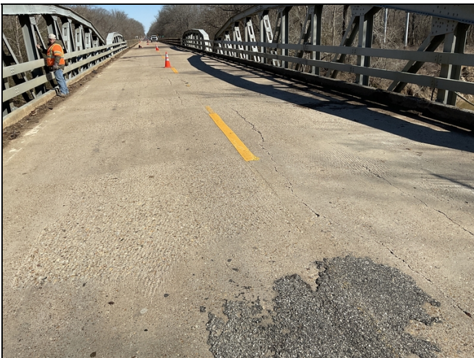
Deck cracks span 12
