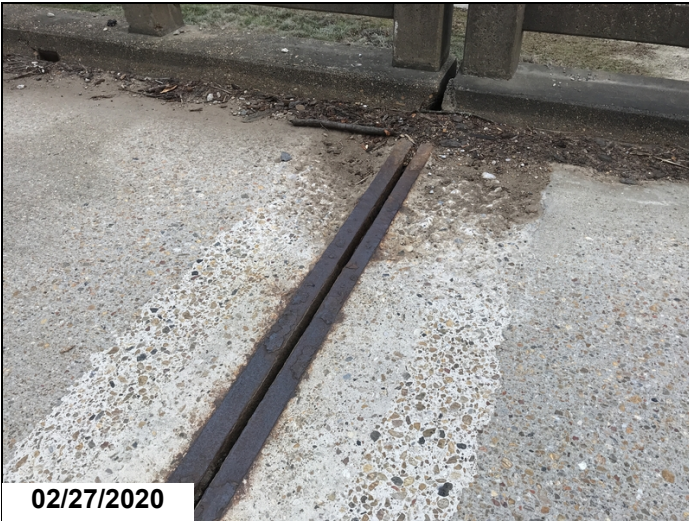
Bent 9 Rt. Side of bridge deck @ joint has spalled out about 3' away from curb into travel lane approx. 2" deep.
