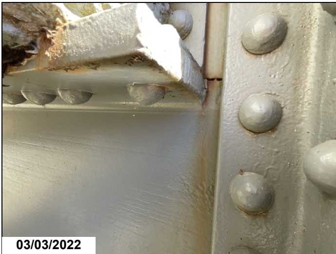
Truss 2 at L9 crack in FB
