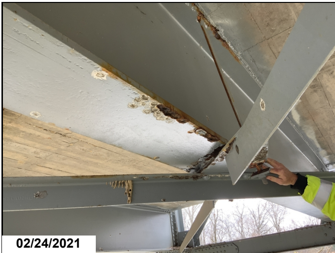
Truss 2, fb 4, cross bracing hanger bolt broke
