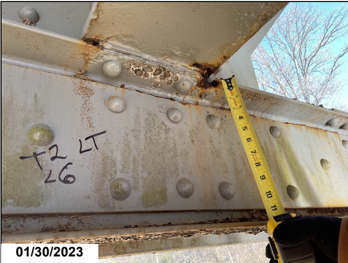
01/30/2023 T2 L6 Lt. Inside C-channel of lower chord. Top flange 1/2" hole in the outside of the top flange.
