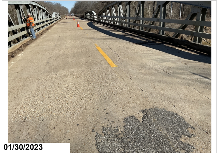
Deck cracks span 12
