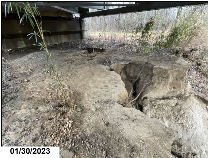
Erosion below span 13
