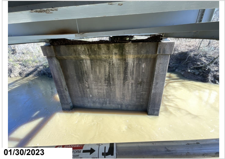
Bent 13, columns and pier wall have abrasion.
