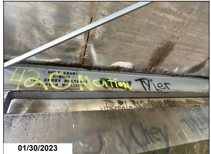
Truss 1, FB 1, corrosion along the flanges.
