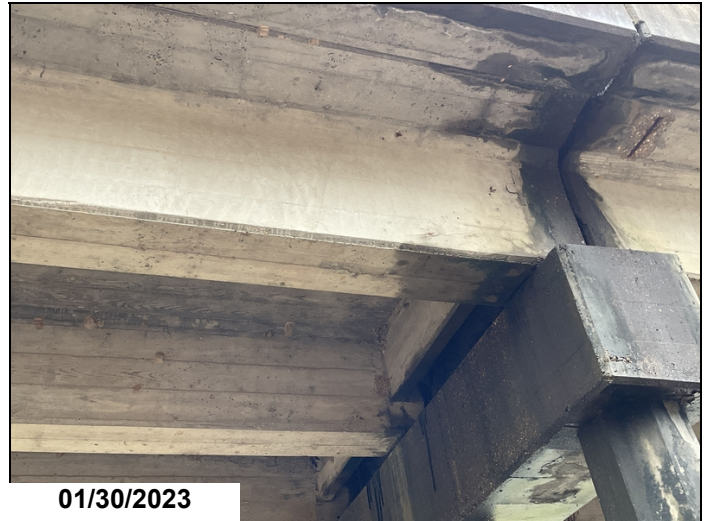
Span 5 @ Bent 5, Girder 1 has a small delam & crack 2' long horizontal crack that is 0.025".
