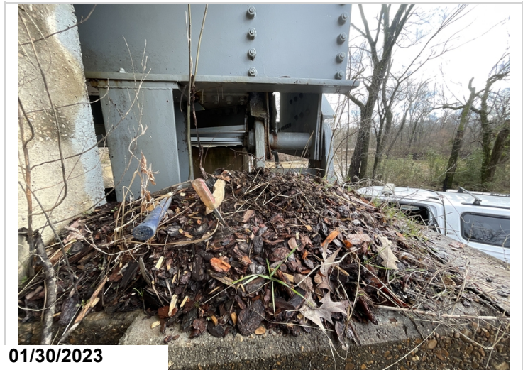
Bent 11, debris built up around the bearings.
