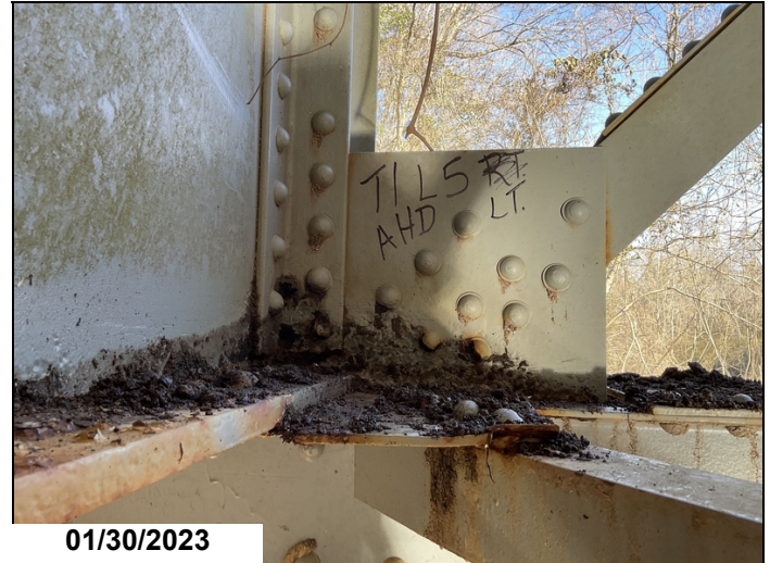
01/30/2023 T2 L6 Rt. Inside C-channel of lower chord. Top flange pitting upto 1/4".
