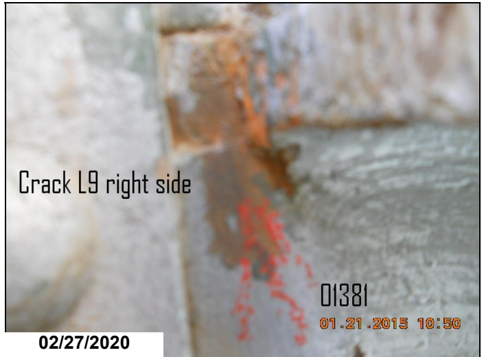
Truss 2, L9 Rt., crack in web of FB.
