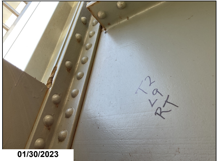
T2 L9 Rt. Crack repaired, hole drilled & arrester installed.
