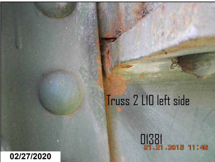
Truss 2, L10 Lt. crack in web of FB.
