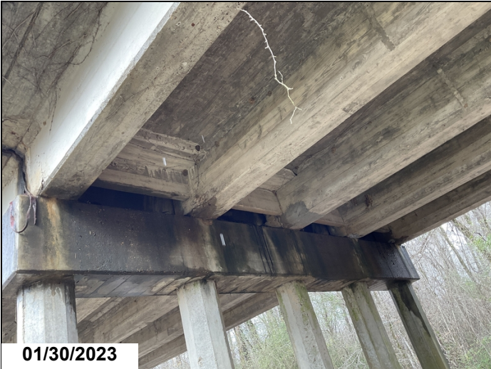
Span 9 @ Bent 9, Girder 1 has 2' long horizontal crack 0.025, Girder 3- 5 have small spalls with exposed rebar.
