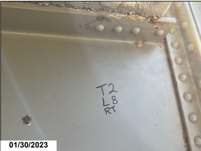
T2 L8 Rt. Crack repaired, hole drilled & arrester installed.
