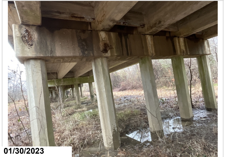
Bent 18 cap, ahead side, spalls with exposed rebar.
