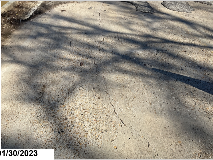
Crack in deck span 11
