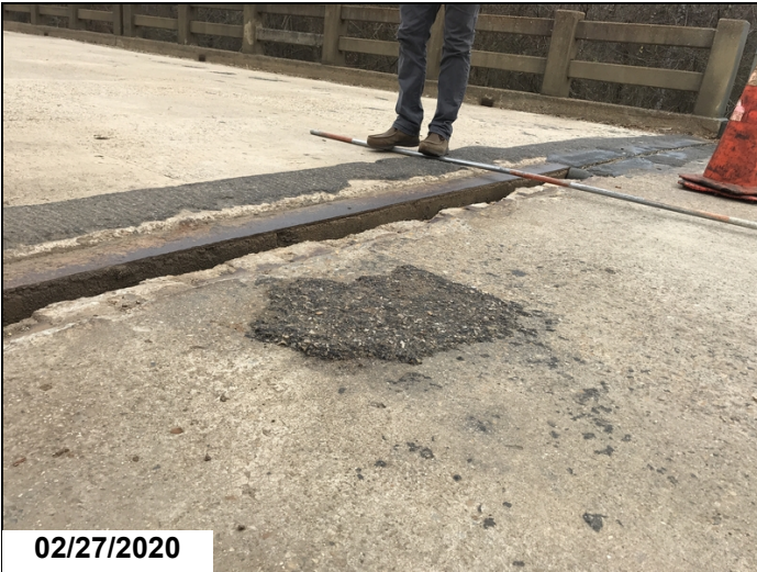
Joint between T3 & approach span, the gap is 4" & there is about a 2" drop from approach span to T3. Road iron on T3 Lt. from C/L Lt.
