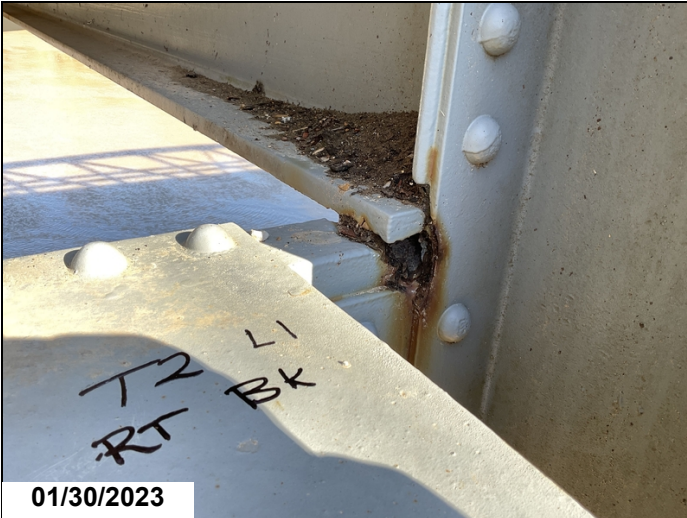
01/30/2023 T2 L1 Rt. Inside C-channel of lower chord. Pitting to top flange & web 3/8" deep.
