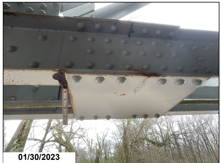
Truss 1, right, splice just ahead of L3. Pack rust at connection plates & bottom flange has section loss upto 1/8" deep.
