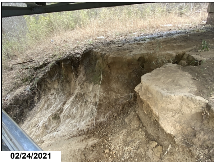
Bank erosion under truss 3
