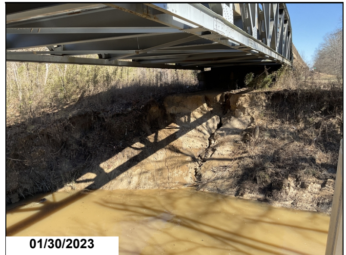
Span 13, Erosion of embankment towards Bent 14.
