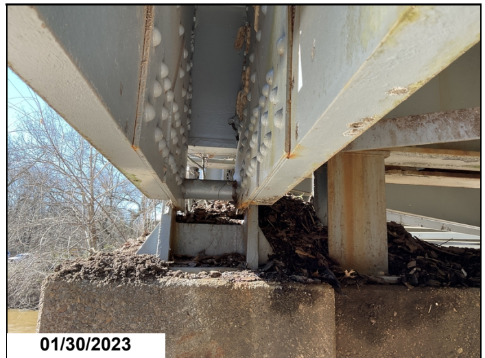
T3, LO, Rt, gusset connection has pack rust.
