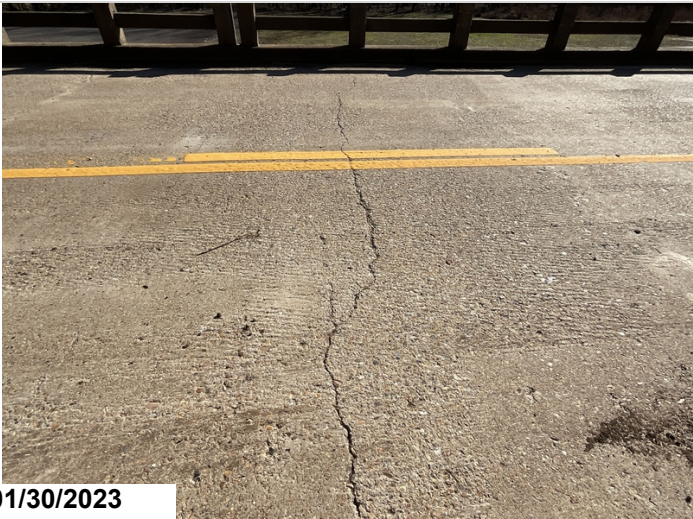
Span 1 transverse crack
