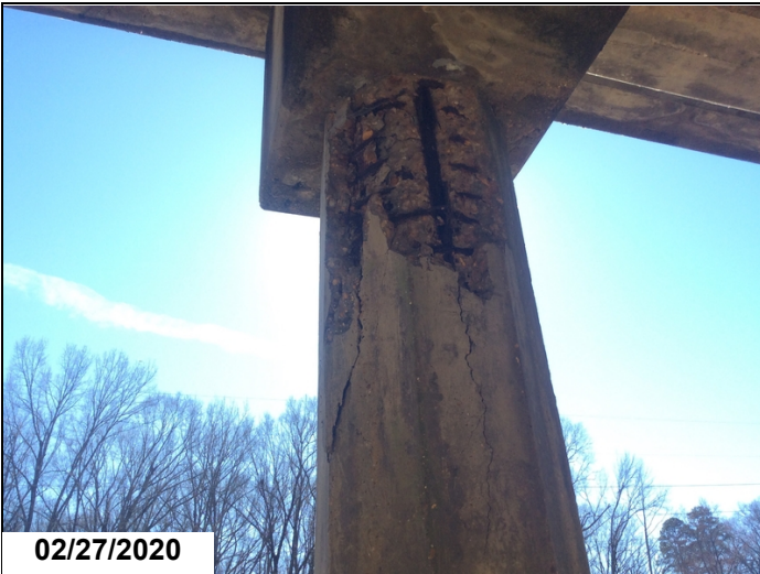
Bent 3, pile 5 has a large spall at top of pile, with exposed steel, with about 2' of cracks coming down the face of the pile below the bottom of the spall.
