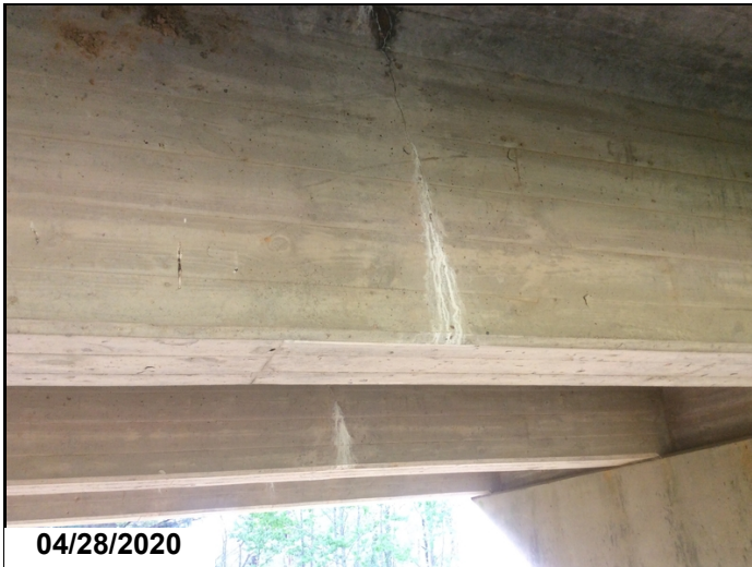
Span 10 girder 2, crack with efflorescences.
