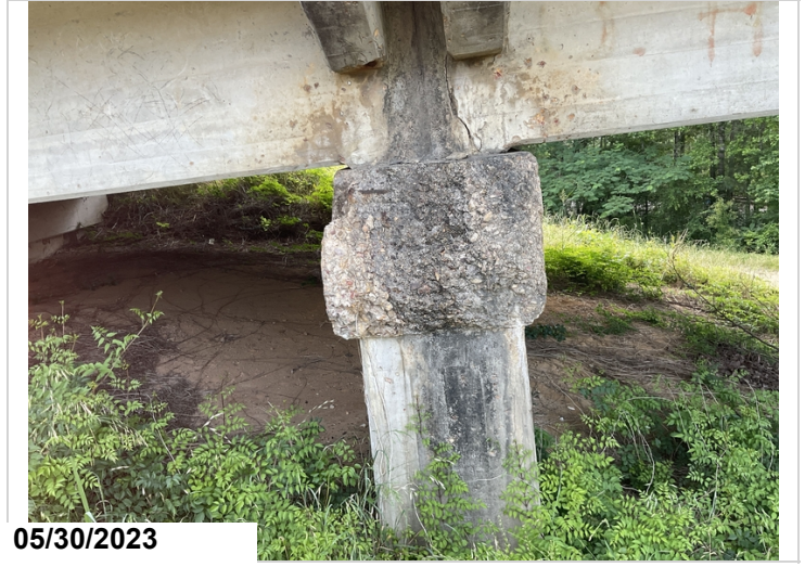
Bent 11 right end of cap spalled
