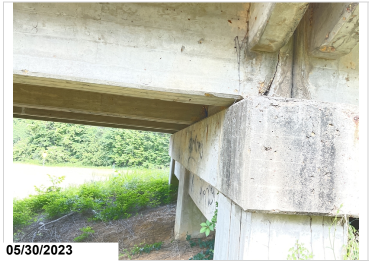
Span 10 bent 11 cracks in girders 3 and 4
