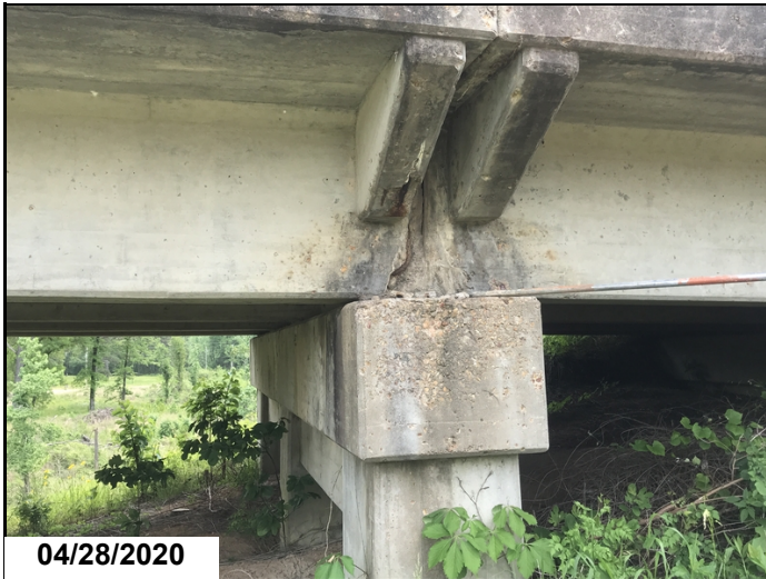
Span 2 girder 1 spalled
