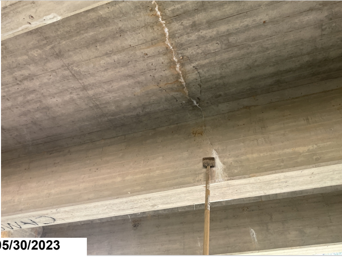
Span 10 girder 3 vertical crack 0.050" with efflorescence
