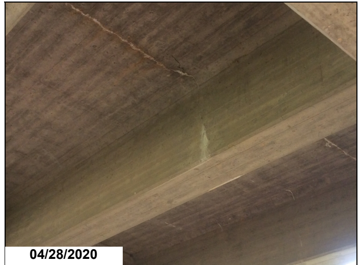
Span 10 cracks in girders
