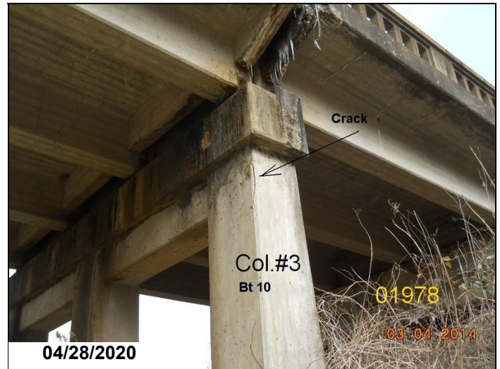
Bent 10, column 3 has a large crack on back side below bottom of the cap.
