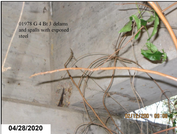
Bent 3 girder 4 with delamns and spalls with exposed rebar.
