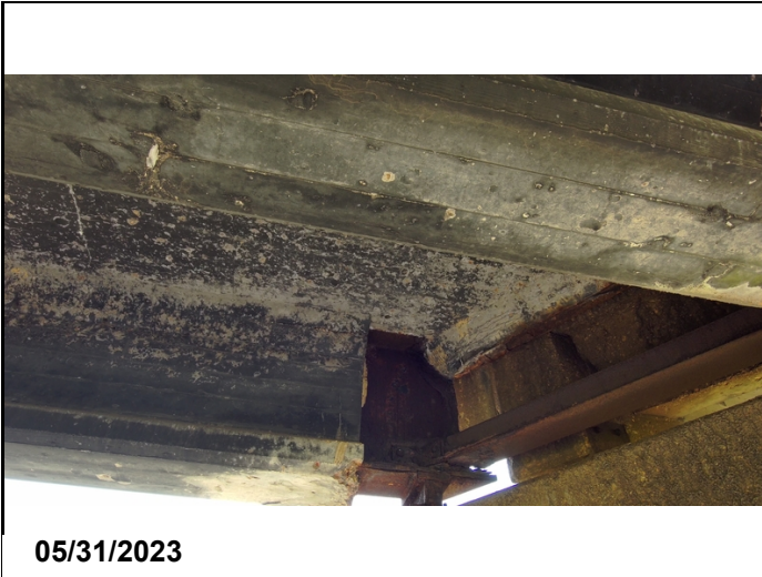
Span 6, Beam 5 @ Bent 6, flange and bottom web have upto 1/8" pitting at the beam end.
