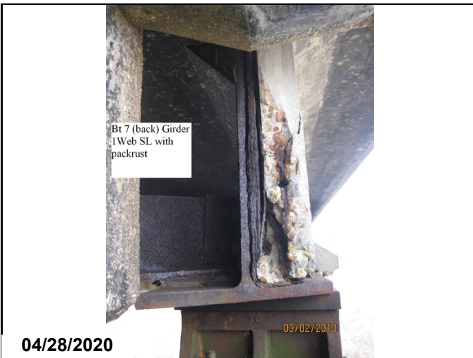
Span 6 @ bent 7, girder 1 web has heavy pack rust that is causing the encasement to shell off the girder.
