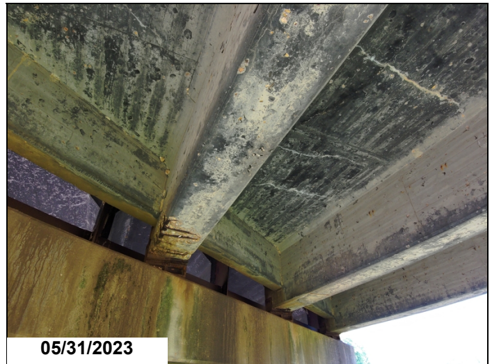
Span 7 @ Bent 7, Girder 3 exposed rebar.
