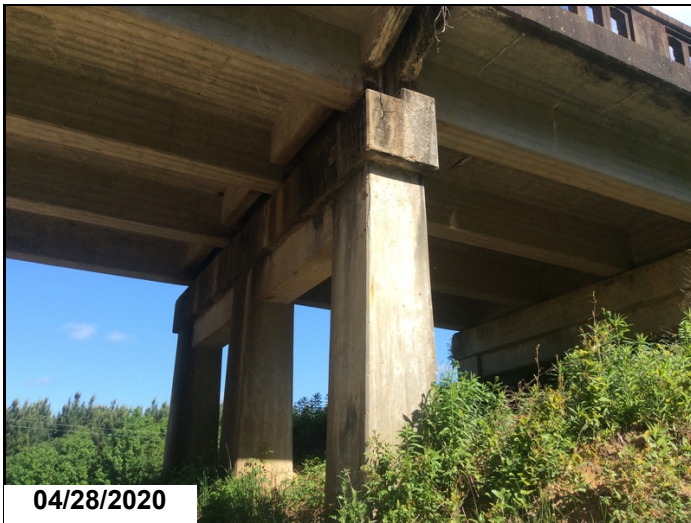
01978 column 3 BT. 10 vertical crack.
