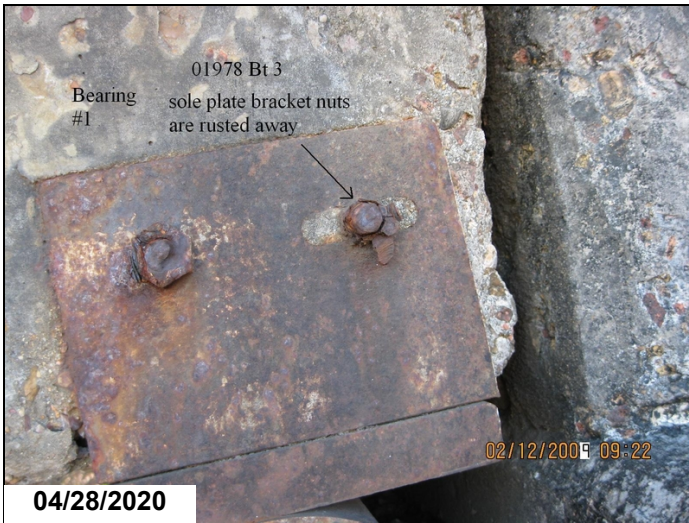
Bent 3 (ahead), girder #1 nuts connecting sole plate bracket to girder is rusted with 100% sec. loss.
