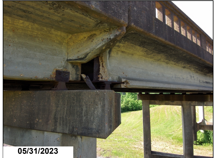
Span 6, Beam 1 @ Bent 7, flange and bottom web have upto 1/8" pitting at the beam end.
