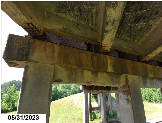
Span 7 @ Bent 7, Girder 2 - 4 have spalls with exposed rebar in the bearing area.
