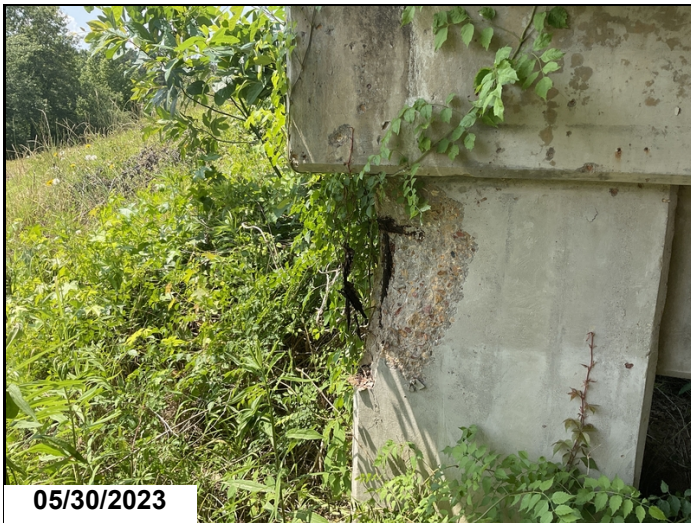
Bent 2 column 3 spalled with exposed rebar
