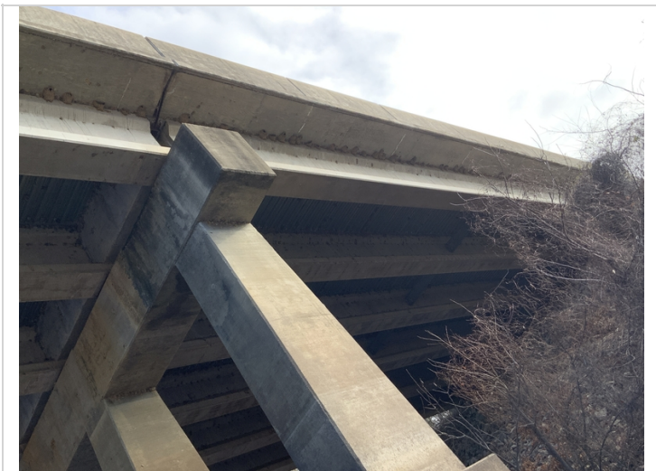
Span 5 right side soffit overhang has cracks with efflorescence.
