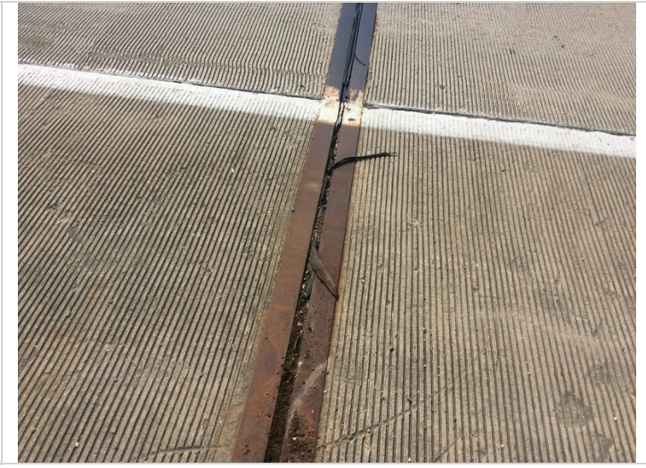
Joint 2, torn and filled with debris.
