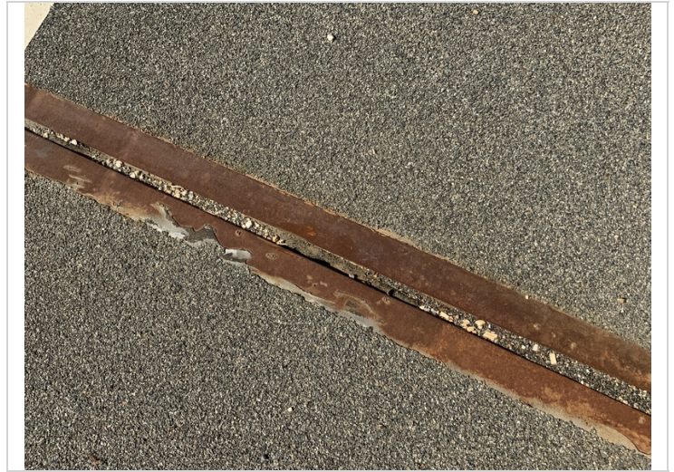
Bent 4 joint seal on left shoulder is torn.
