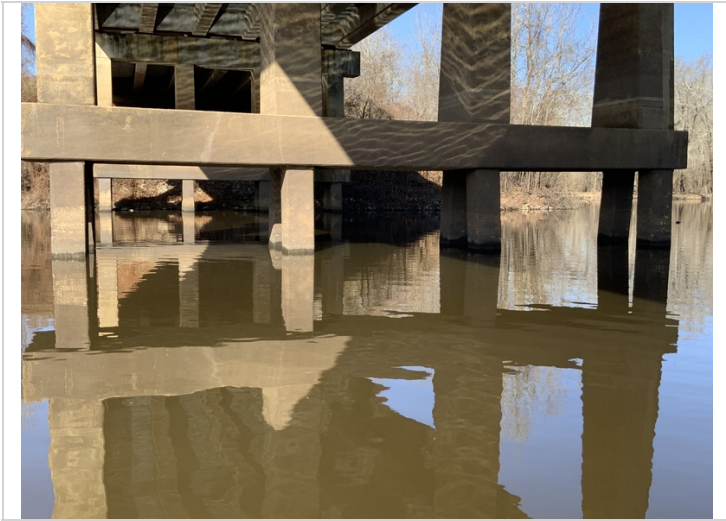
Bents 2&3 piles have abrasion, common bents 4,5,&6.
