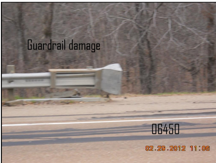
Terminal end post, collision damage.
