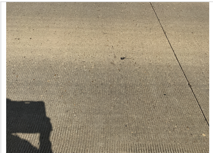
East end approach slab has transverse cracks, common west end.
