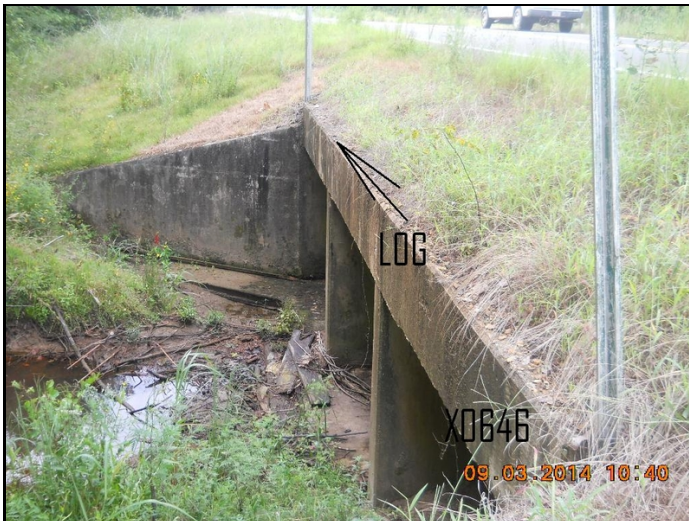
Inlet and ends of box culvert @ barrel #1 is silted in 1/4 of the barrel.
