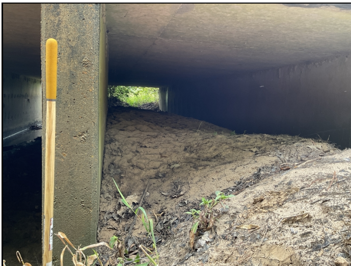
Barrel 1 is half full of sediment.
