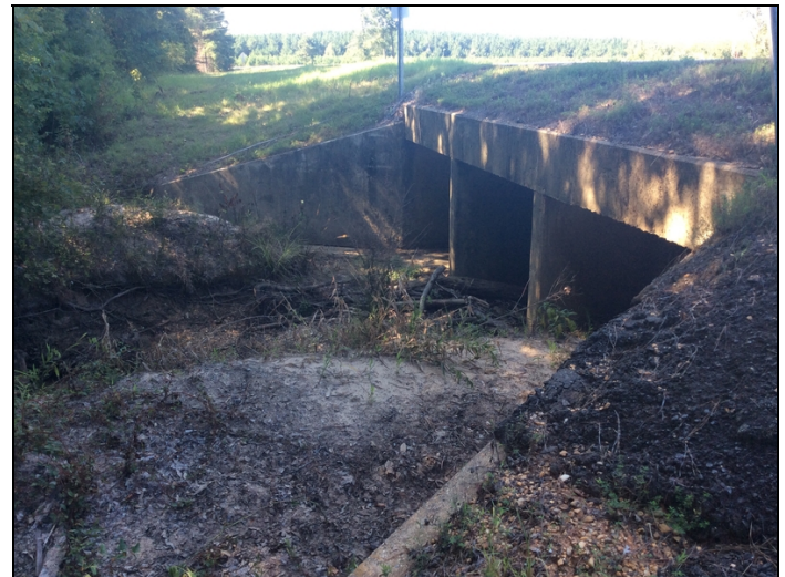
Lt. side of box has significant silt built up just outside the openings.
