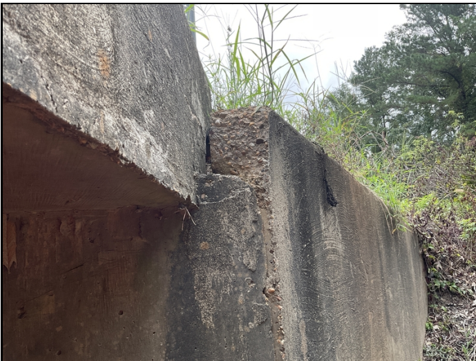
Barrel 4, right wing wall has separated.
