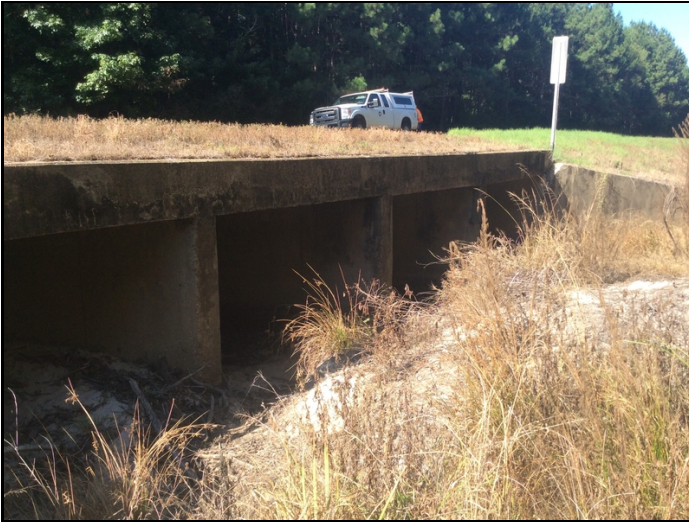
Outlet end, Lt. side has silt built up @ outlet end of all barrels for 3/4 of the openings.
