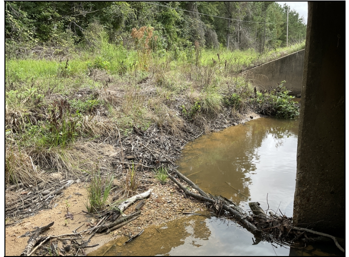
Left of the culvert side has silt built up @ outlet end of all barrels for 3/4 of the openings.
