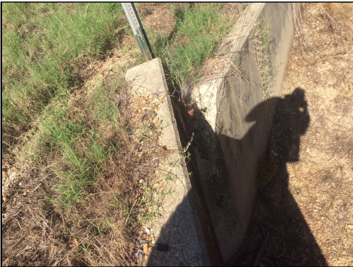
Wingwall left side broke at barrel 1
