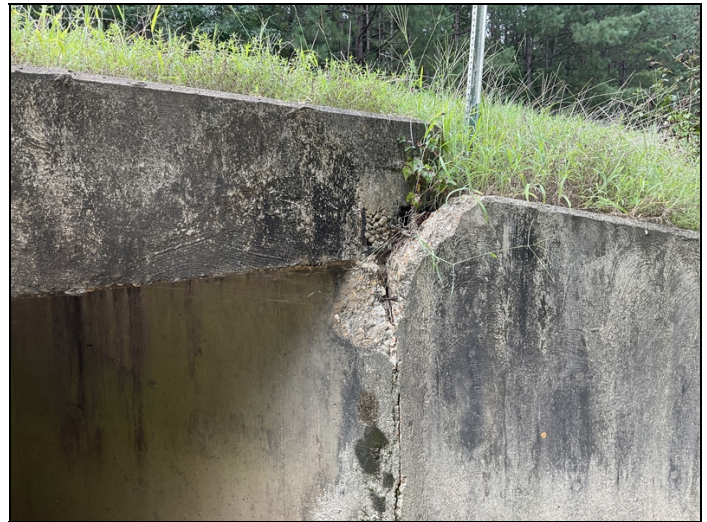
Barrel 1, left side, the wing wall has broken.
