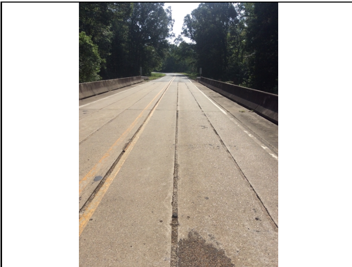
06148 grout missing from key ways
