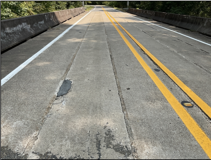
Spalls along the keyways and missing grout.
