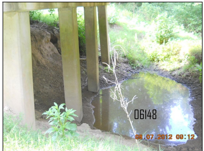
Large hole scoured under span 2 @ Bt. 2.
