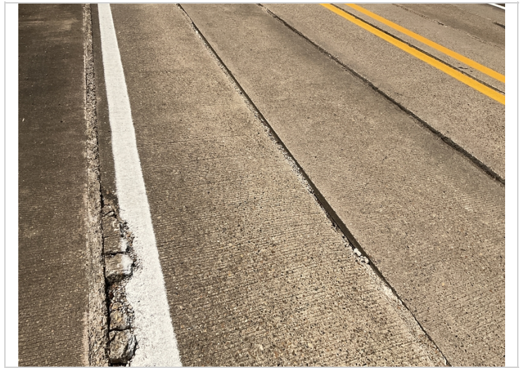
Spalls in the keyways and keyway grout.
