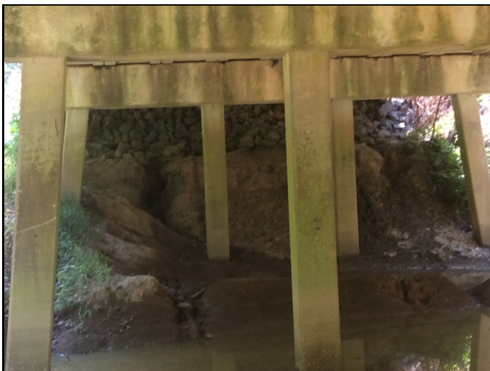
Abutment 2 slope erosion, this is caused by the missing keyway grout.
