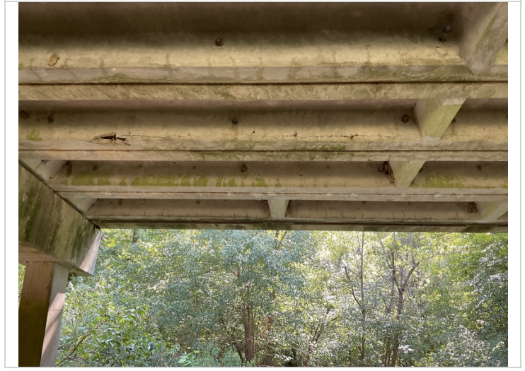
Span 3, girder 7, cracks & spalls with exposed rebar.
