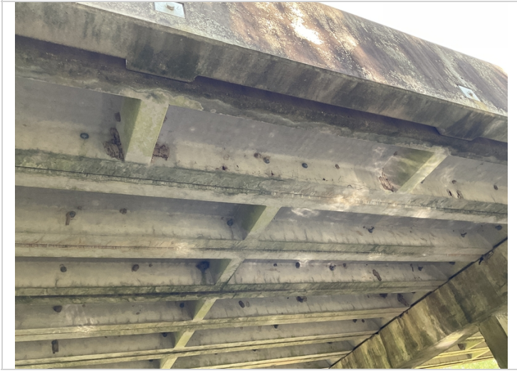
Span 2 girder 8, cracks & exposed rebar.
