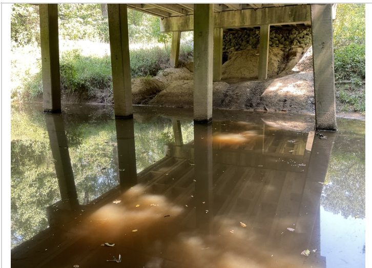
Bt. 3 pile have abrasion
