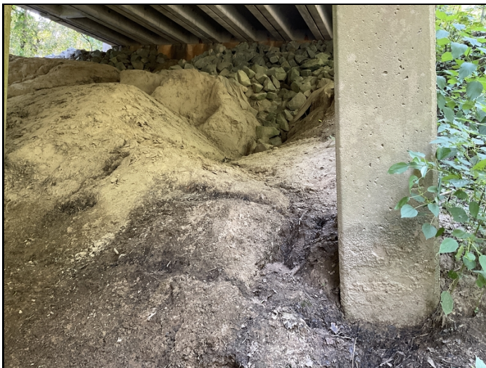
Span 1, embankment has been scoured.
