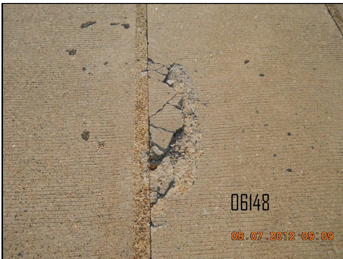
06148 grout missing from key ways
