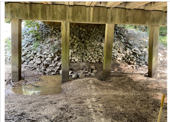
Bt. 3 pile have abrasion
