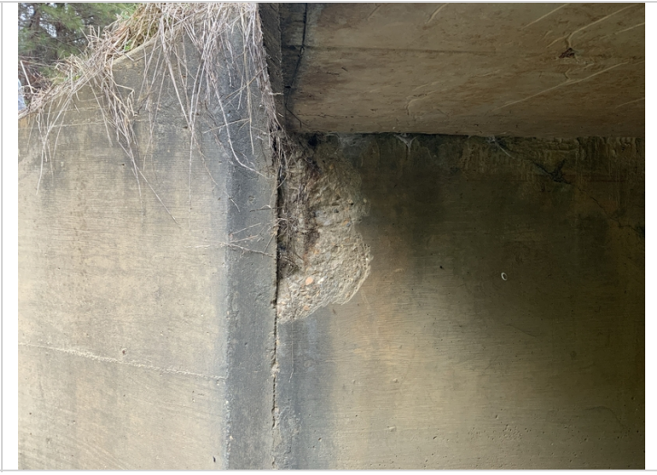
Barrel 4 left end, exposed rebar
