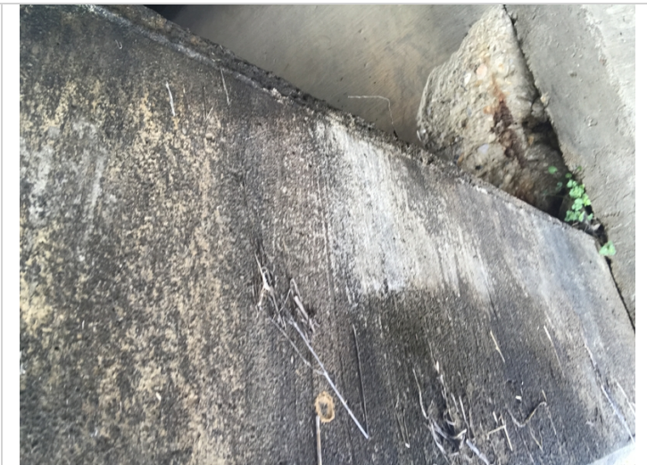
Barrel 4 left side, outside wall, spall with exposed rebar.
