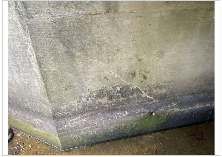
Barrel 1 crack with efflorescence outer wall
