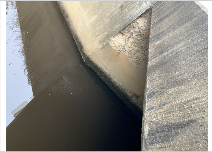
Barrel 4 spall with exposed rebar.
