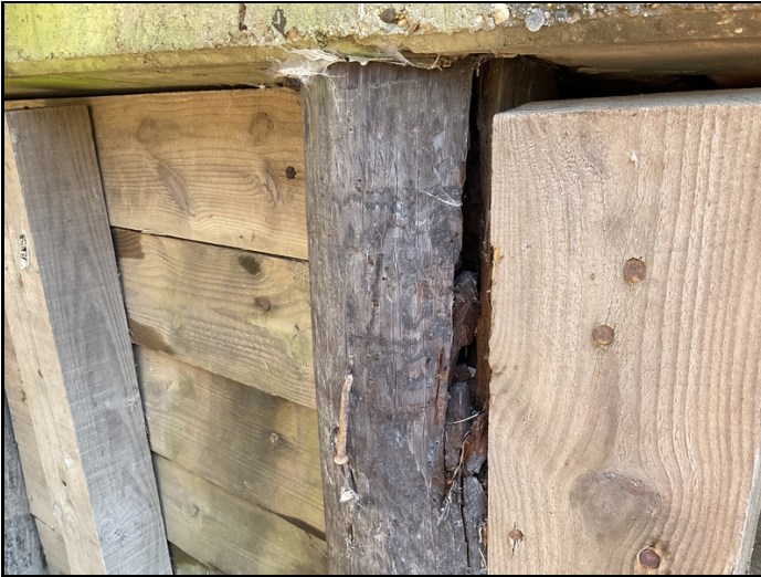
Bent 1 pile 1 is hollow.
