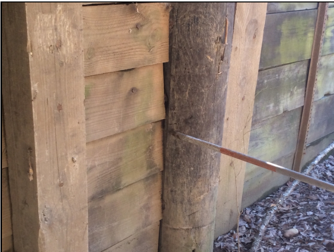
Bent 1 Pile 1 hollow & outer shell has split vertically @ the backwall.
