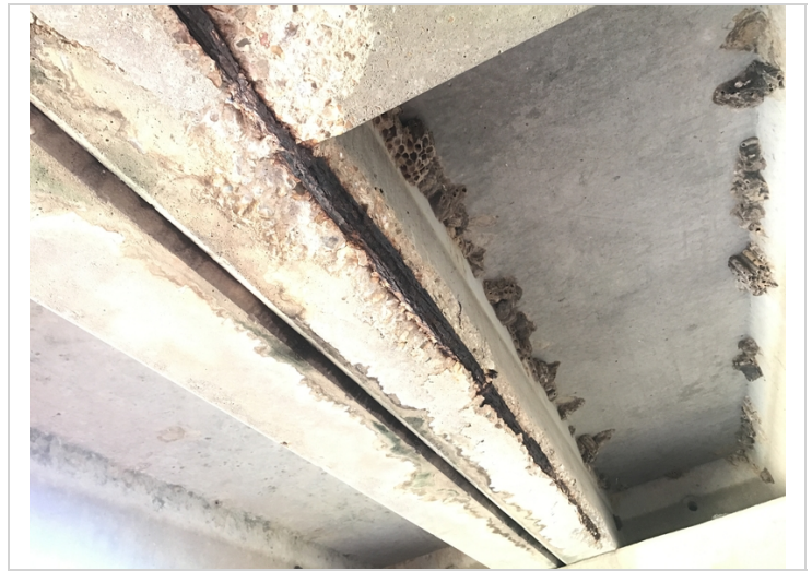
Span 1, unit 6, left leg, section loss to rebar.
