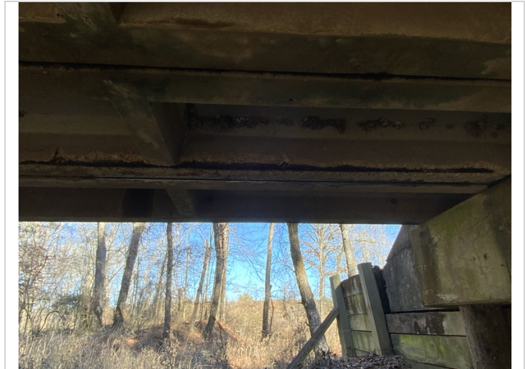
Span 1 unit 6 exposed rebar right leg.
