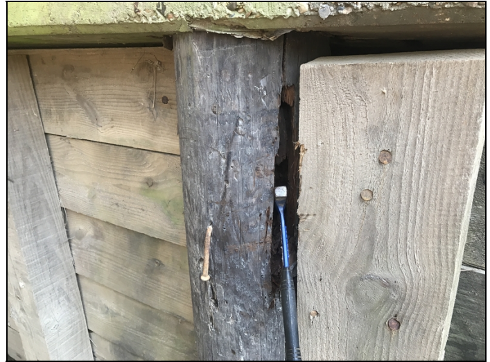
Abutment 1 pile 1 inside decay
