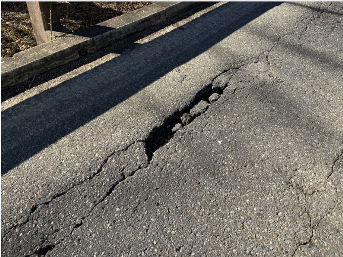
Spall in asphalt wearing surface
