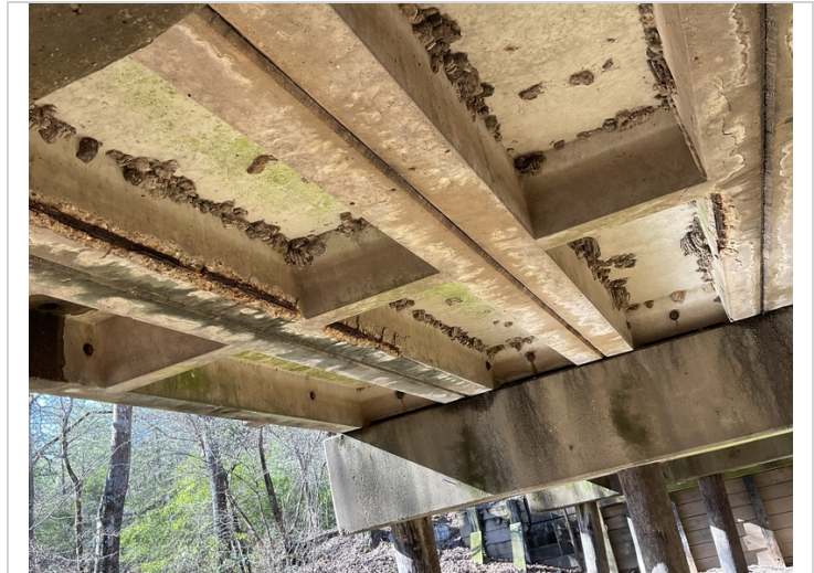
Span 3 units 2 and 3 legs have spalls with exposed rebar.
