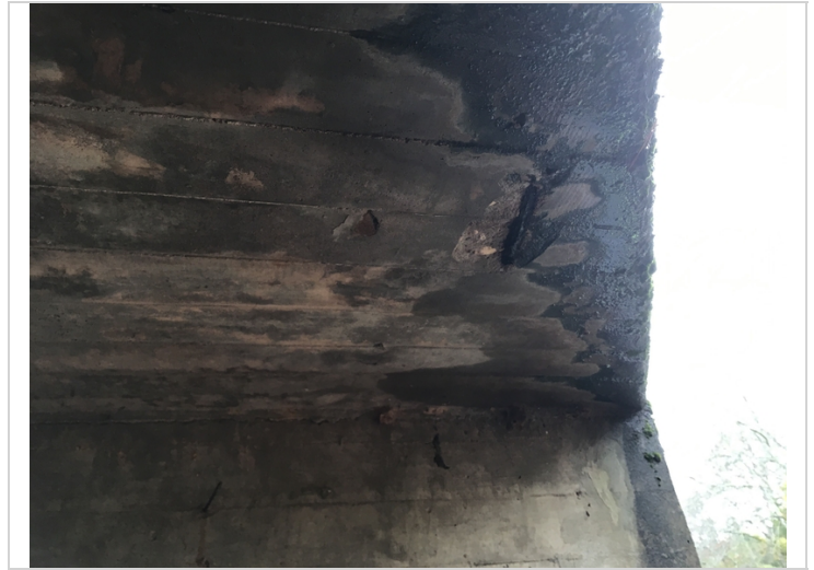
Right end of barrel #1 has exposed rebar in the top of the barrel.
