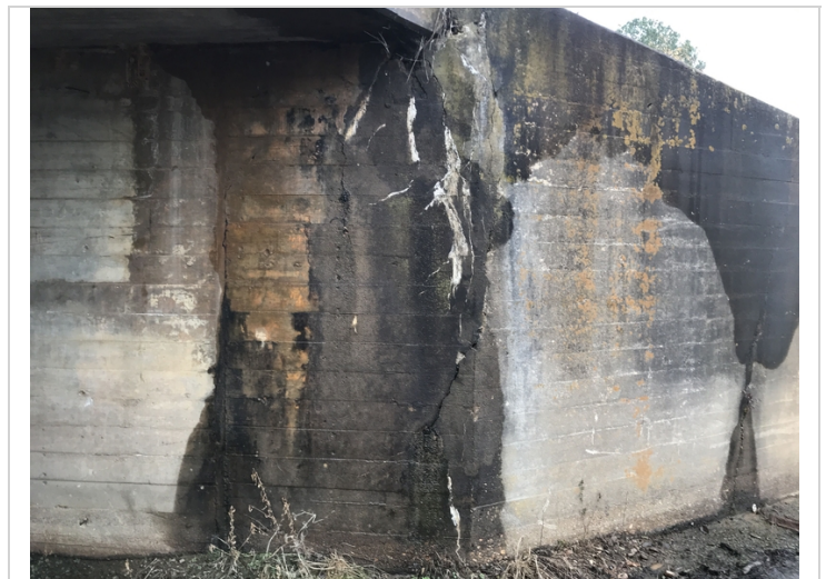
Barrel #1 left end has moderate vertical cracks with minor efflorescence at the connection.
