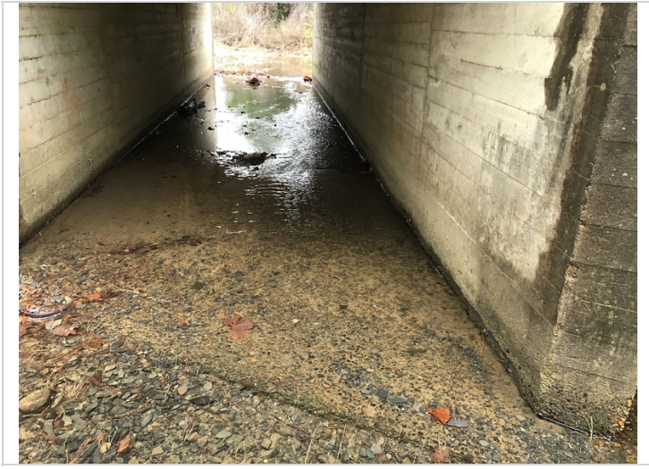
Barrels 2 & 3 have minor abrasion throughout the full length of the floor.
