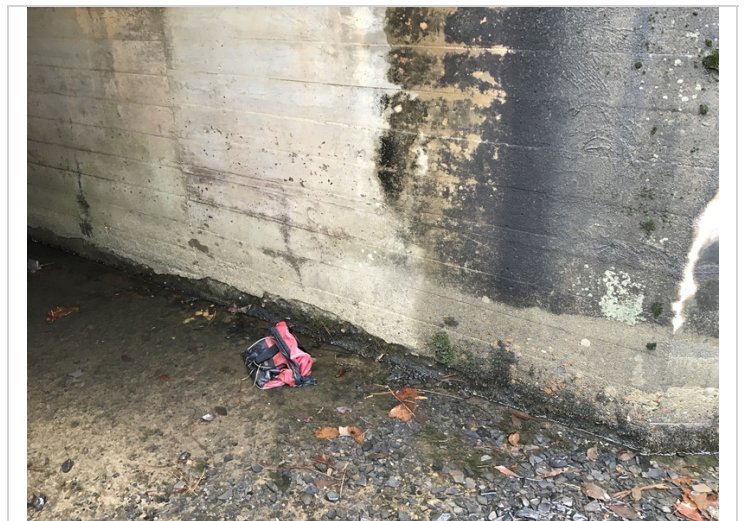
Bottom of the walls in barrels 2 & 3 near the right end have minor abrasion.
