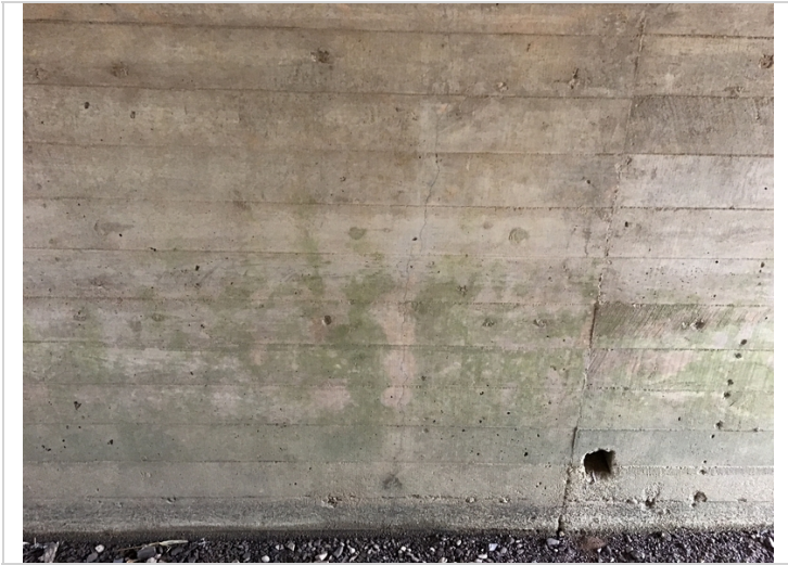
Few minor vertical cracks in the walls of barrels.
