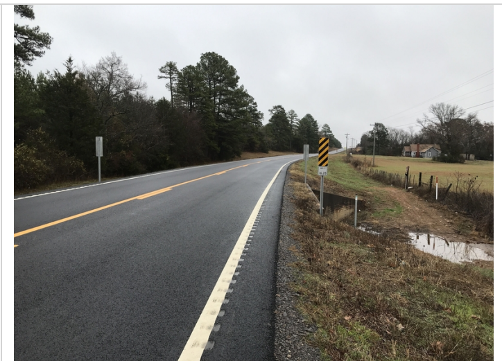
East bound log mile marker sign is incorrect, the west bound log mile marker sign is missing.
