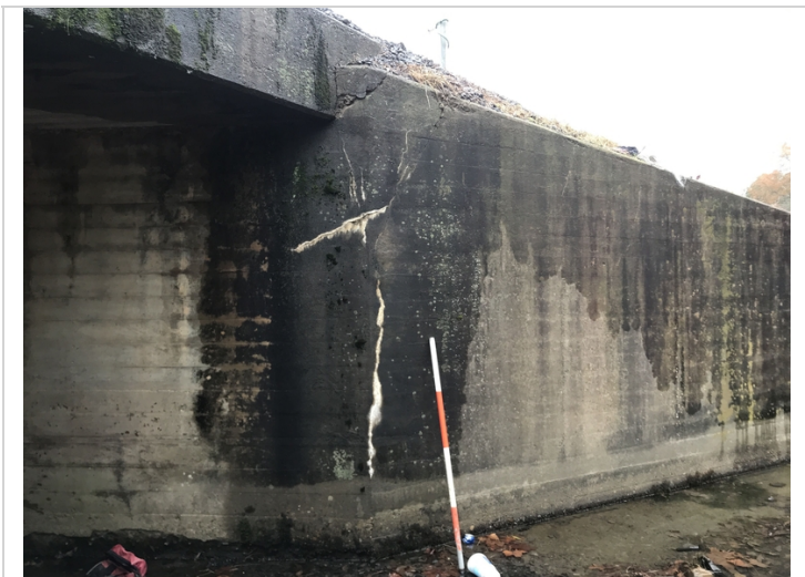
Right end of barrel #1 has minor to moderate vertical cracks with moderate efflorescence.
