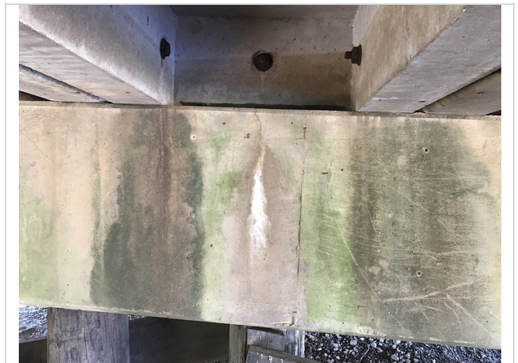
Bent 6 crack in cap over pile 5
