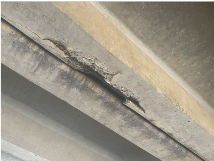
Span 8 unit 5 left leg 5' from bent 8 has exposed rebar.
