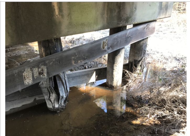
Bent 8 piles 7 and 9 typical of old rotten piles.
