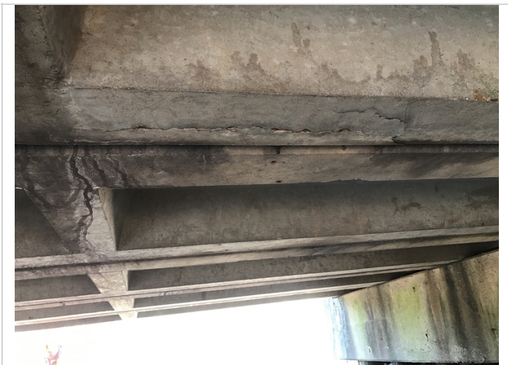
Span 10, unit 5, crack in bottom left leg.
