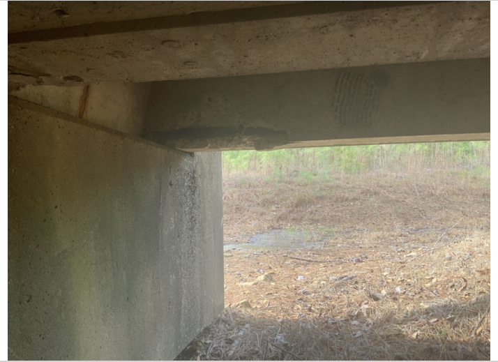
Span 11 unit 1, left leg, exposed rebar at bent 11 bearing area.
