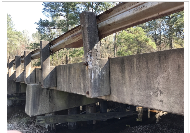
Span 5 left side post and rail damage
