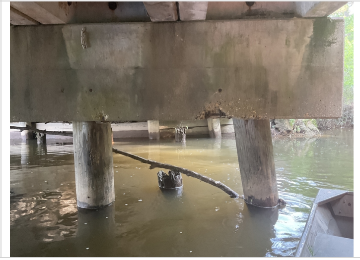
Bent 2, exposed rebar in the bottom of the cap.
