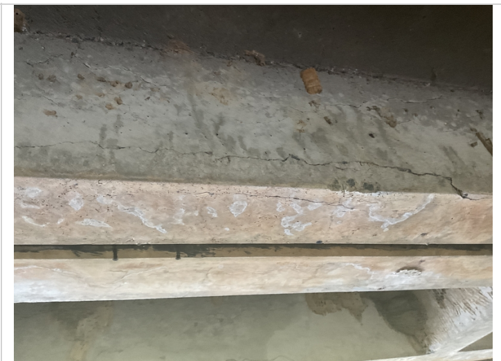
Unit 4 span 2, large cracks on the bottom of the unit leg.
