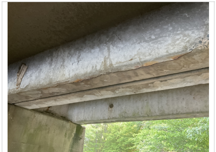
Span 1 unit 6, large crack in the leg of the channel unit.
