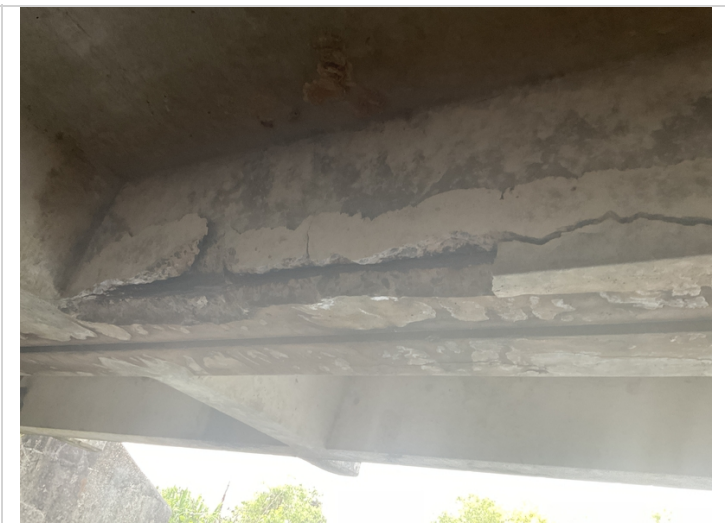
Span 1, unit 2, exposed rebar and large delaminated area in the unit leg.
