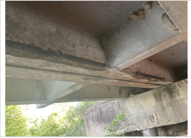
Span 2 unit 2, exposed rebar in the channel leg.
