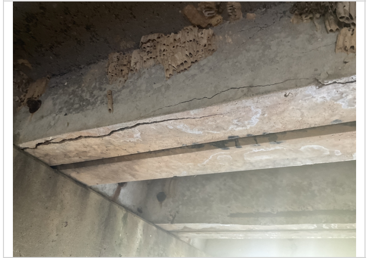
Unit 3 span 2, large longitudinal cracks on the bottom of the unit leg.
