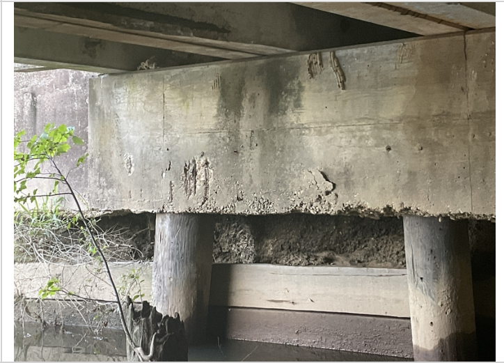
Bent 3 left side, exposed rebar in the face of the cap.
