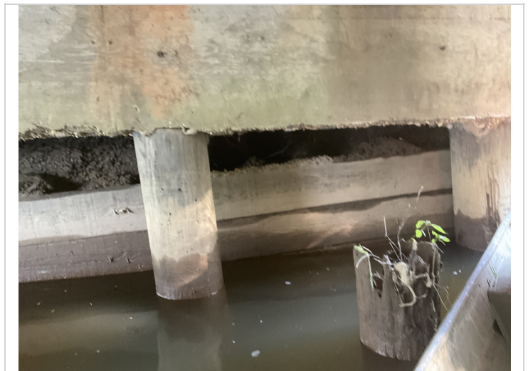
Bent 3, large void behind the timber cribbing.
