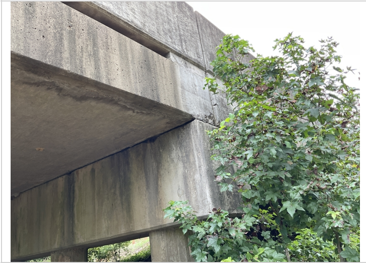
Span 2 & 3, right side at Bt. 3, spalls in the end of the slab.
