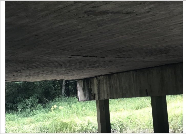
Span 2 @ C/L of bridge @ middle of span there is a 3' - 4' delamn on soffit of deck.
