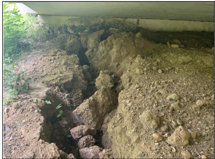
Abutment 1 erosion goes back under the abutment cap.
