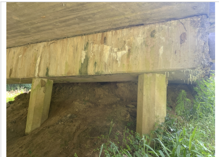
Bent 4 cap back cracks with efflorescence.
