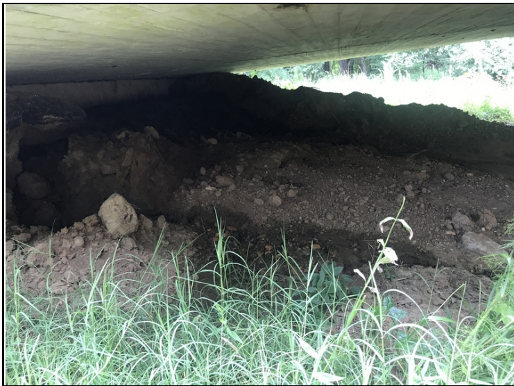
Abutment 1 erosion
