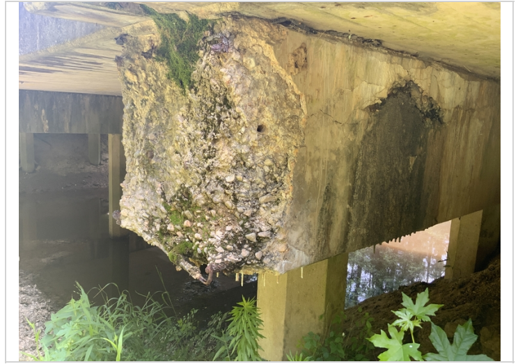
Bent 4 cap right end exposed rebar.
