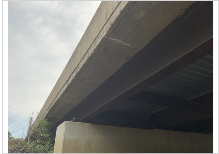
Soffit efflorescences
