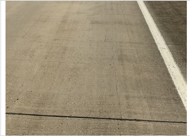
Transverse and longitudinal deck cracks 0.040 max
