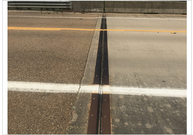
Joint material abutment 1
