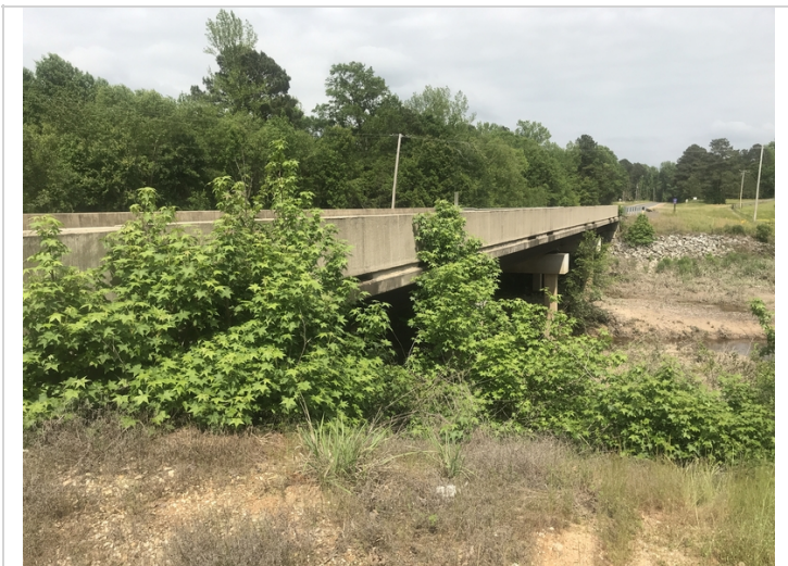
Span 1 looking ahead @ vegetation growing up beside & back under the bridge, this is typical of both sides of the bridge.
