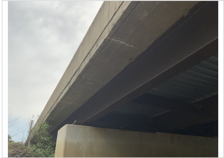
Soffit efflorescences
