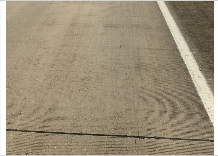
Transverse and longitudinal deck cracks 0.040 max
