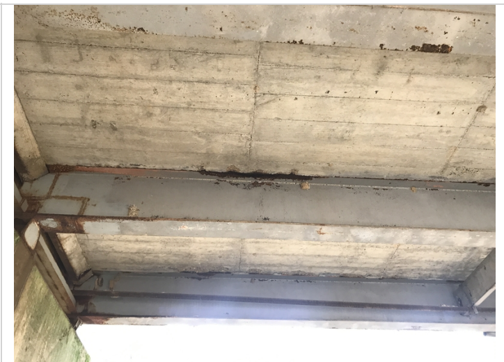
Span 3 girder 2 corrosion to top flange.corrosion
