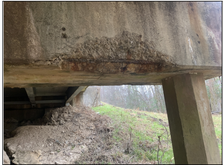
Bent 5 cap large spall with exposed rebar.
