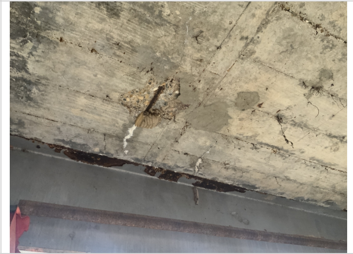
Span 1 soffit has spall with exposed rebar.
