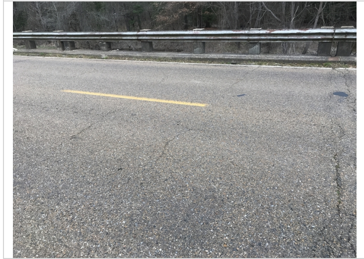
Wearing surface 481' of cracks.26xlength.
