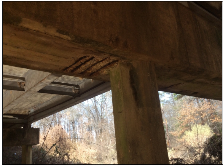
Bent 3 cap, spall between piles 2 & 3 with exposed steel & section loss.
