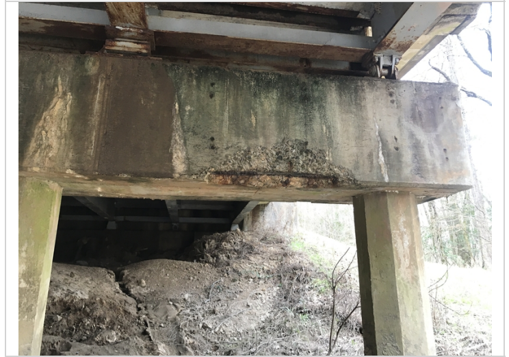
Bent 5 back side between piles 3 and 4 large spall with exposed reinforcing steel.
