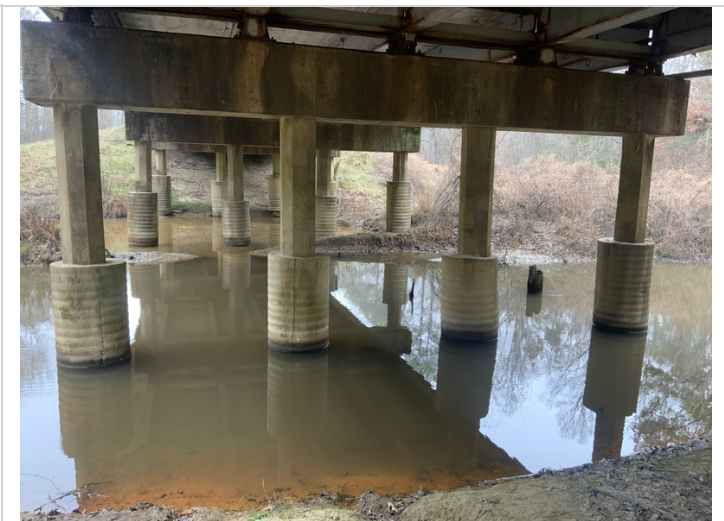
Bents 2-4 piles with cracks or spalls have been repaired with collars.
