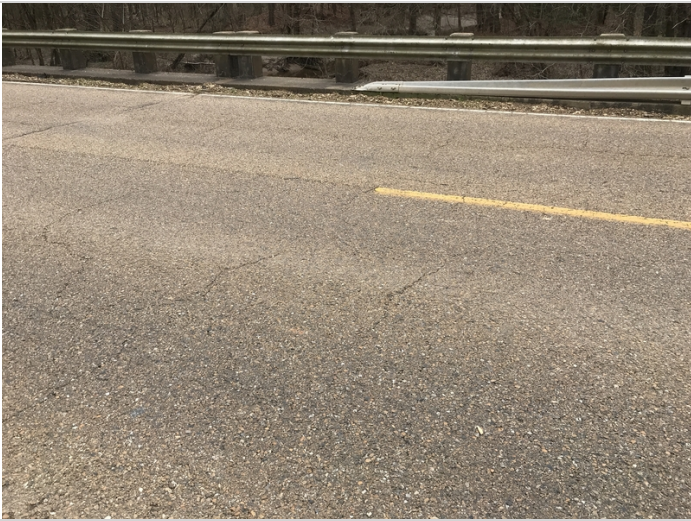
Typical cracking in wearing surface.
