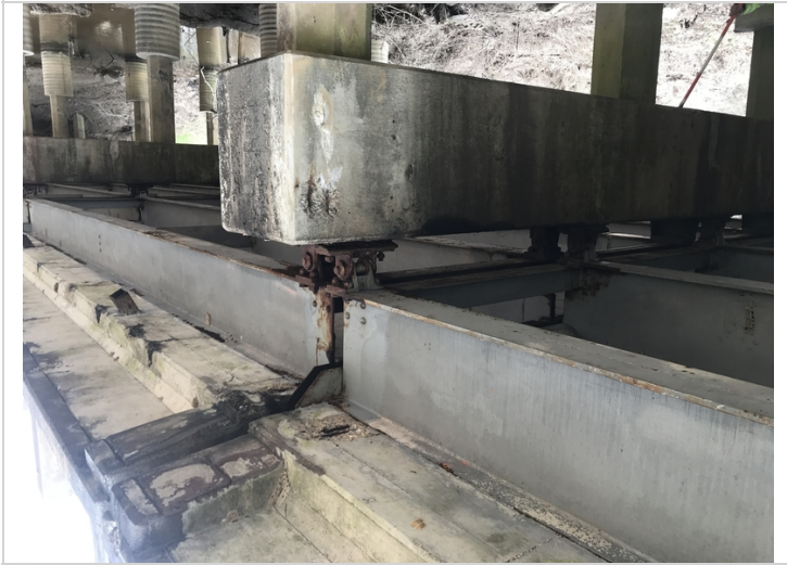
Bent 2 corrosion to moveable bearings.
