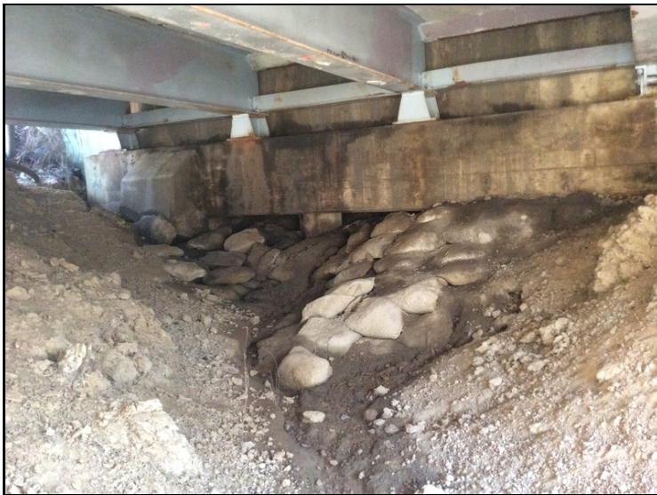
Abutment 2 cap has scour between piles 2 & 3, with pile 3 exposed (1').
