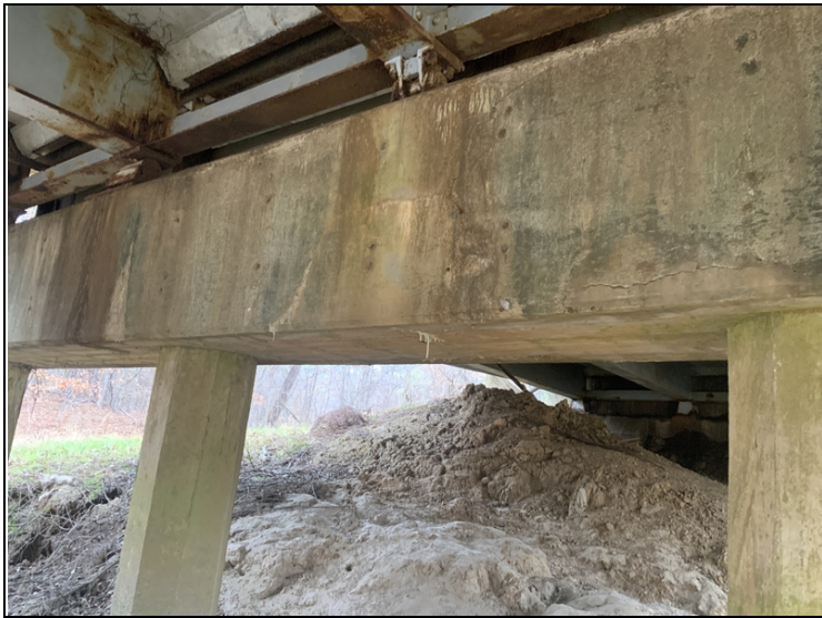
Bent 5 cap cracks with efflorescence.
