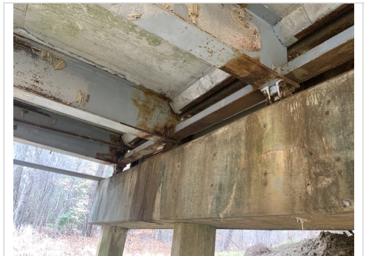
Span 4 bent 5 beam ends have corrosion.
