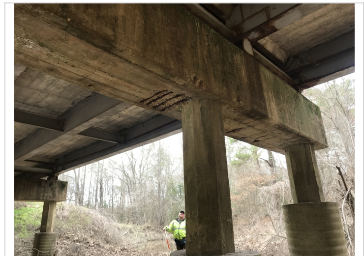
Bent 3 under side of cap has exposed reinforcing steel.
