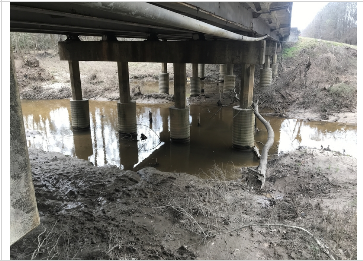
Repairs on piles at bents 2 thru 4.
