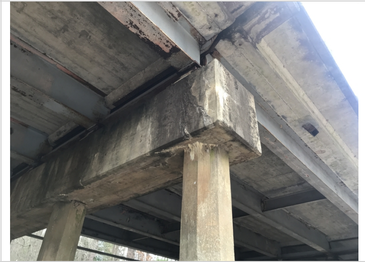
Bent 4 right side has efflorescence cracking.
