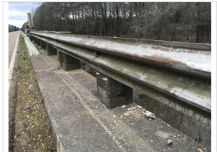
Loose connection span 2 left side.
