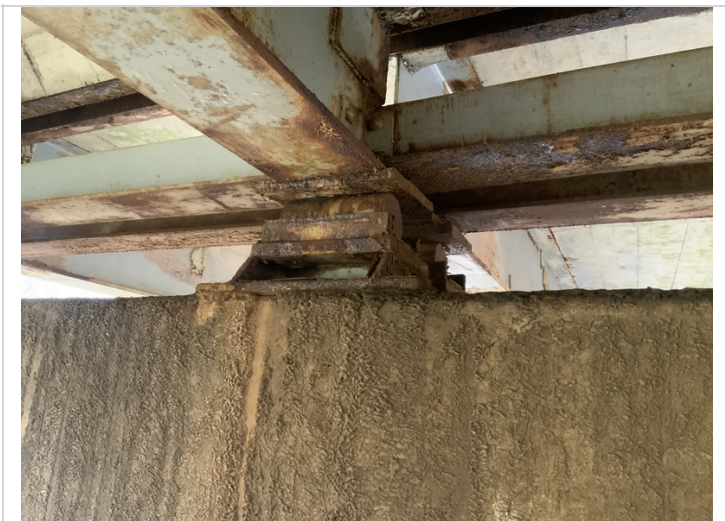
Bent 5 span 5 bearings have active corrosion.
