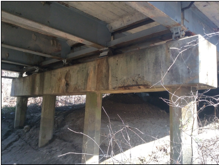
Bent 5 cap with large spall with exposed steel & section loss, between piles 3 & 4. Also cracking & delamination to bottom of cap between piles 2 & 3.
