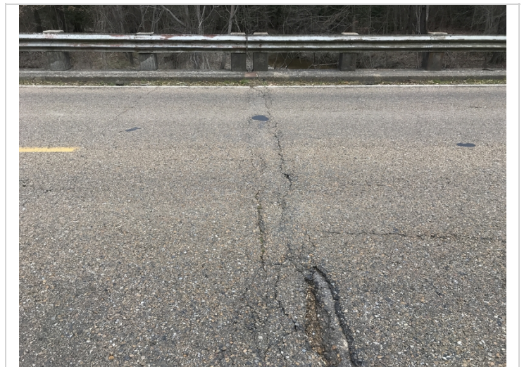
Typical condition of joints.
