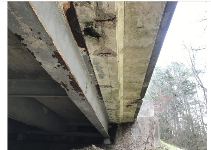
Span 5 right side spalls in the soffits with exposed reinforcing steel.
