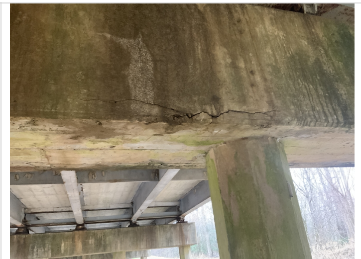
Bent 2 cap back has crack.
