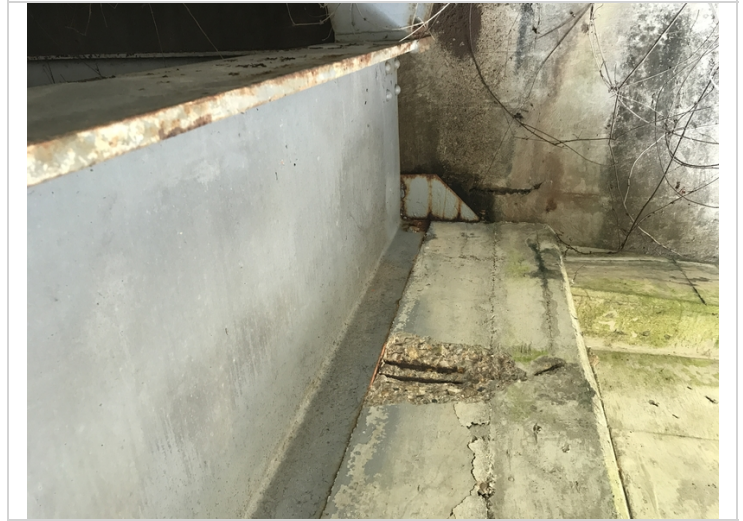
Span 1 right side spall with exposed reinforcing steel.
