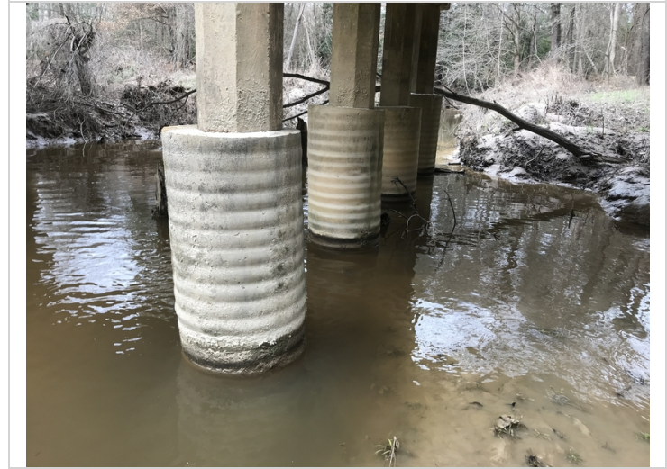
Bent 4 all 4 piles have local scour.
