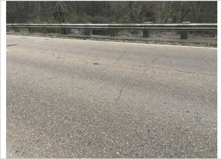
Typical cracking in wearing surface.
