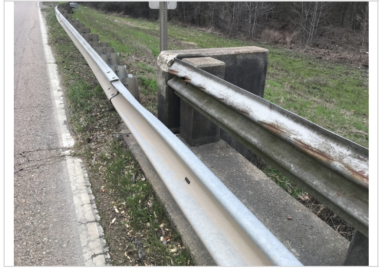
Collision damage to metal rail left side.
