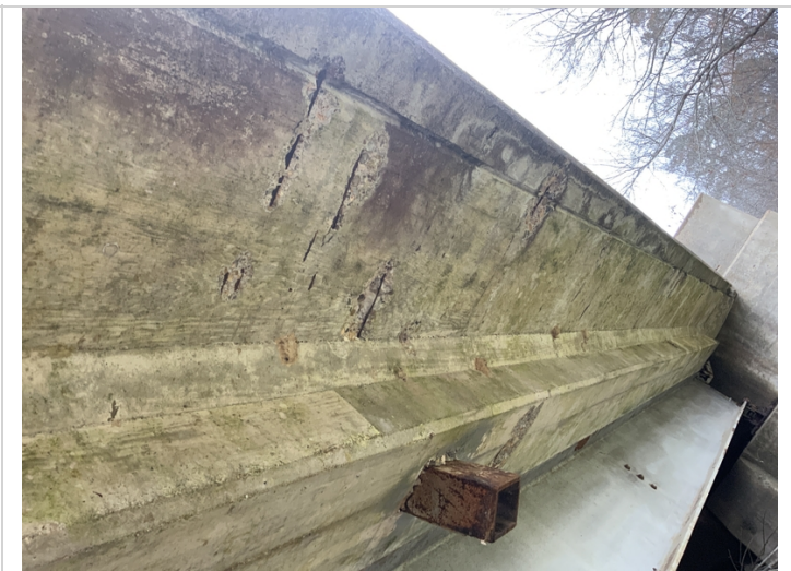
Deck soffit span 4 right side has spalls with exposed rebar.
