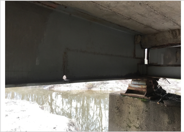
Bent girder5 has a tee splice repair.
