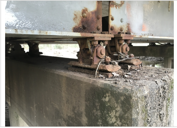
Typical condition of bearings.
