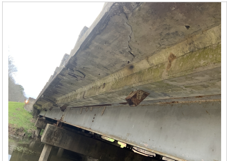
Deck span 3 right side soffit overhang has delams.
