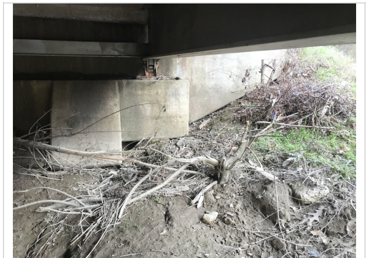
East abutment has erosion under wing wall on right side approximately 10' in length
