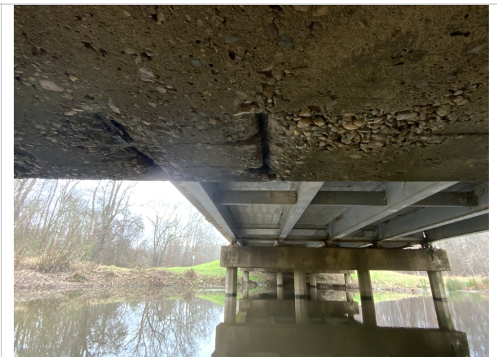
Bent 4 cap has spalls with exposed rebar on bottom of cap between columns 3&4.
