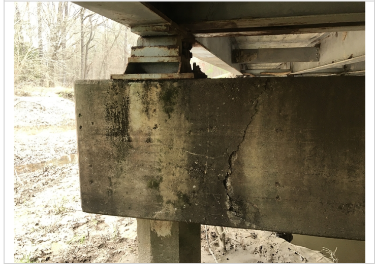
Back side bent 1 left side 2' delam this is typical on bents 3 and 4.
