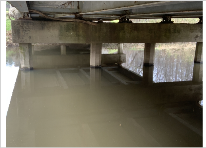
Bent 3 columns have abrasion at waterline.
