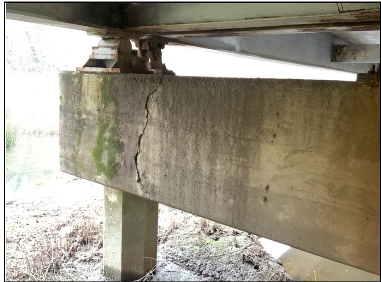
Bent 2 cap cracked between columns 1&2.
