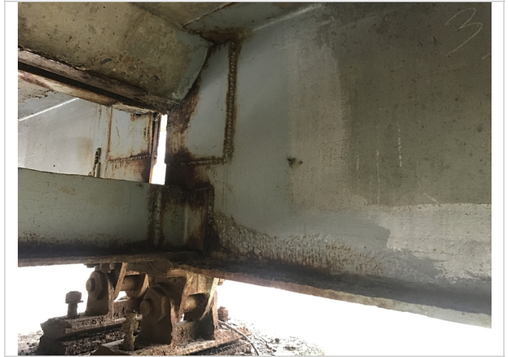
Bent 4 girder 1 has been painted in past, this area has section in lower part of web.
