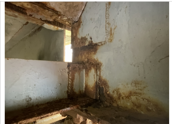
Bent 2 span 3 beam 1 beam end has corrosion.
