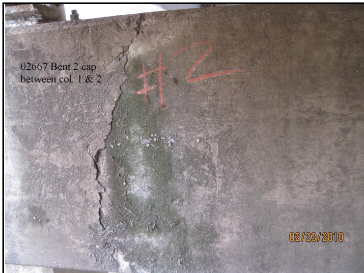
Bent 2 cap is cracked.
