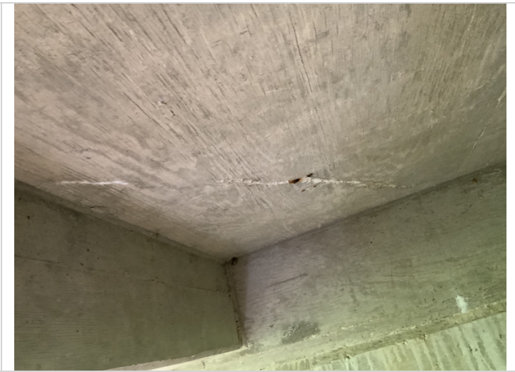
Span 1 soffit cracks with efflorescence, common all spans.
