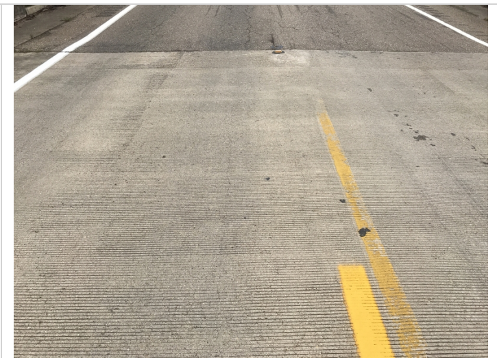
Span 1, longitudinal cracks, max 0.035.
