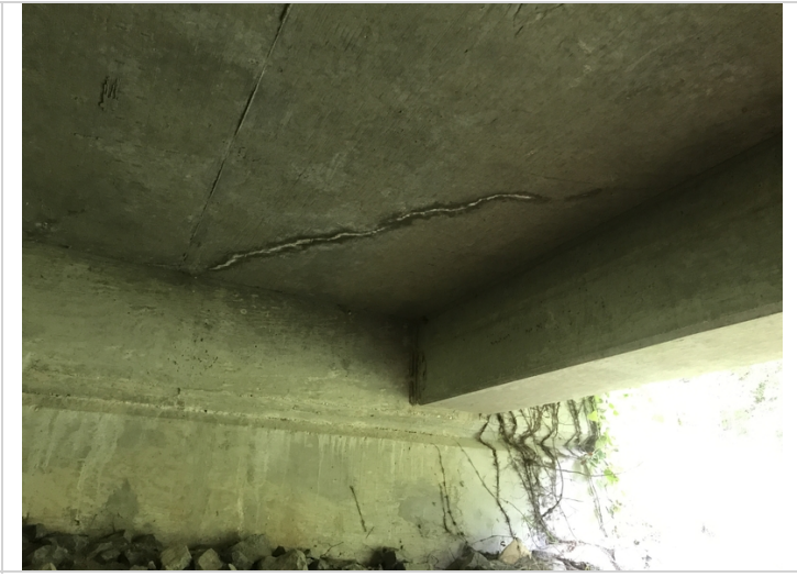
Soffit, span 3 bay 4, diagonal crack with efflorescence.
