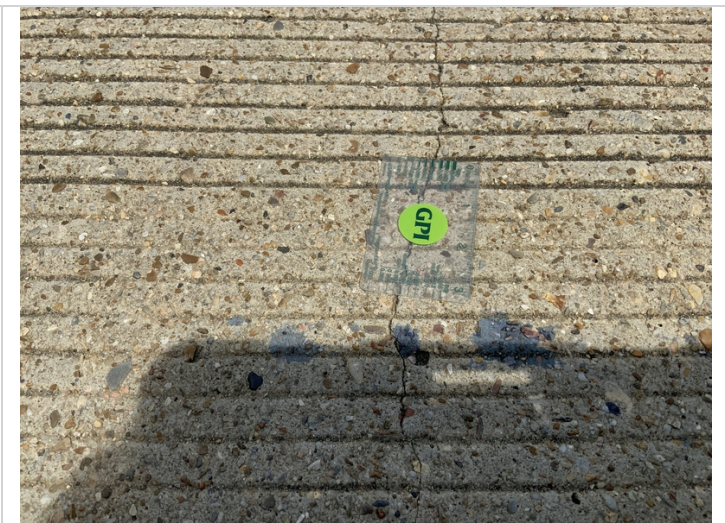
Typical deck crack .040
