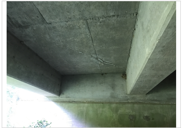
Span 3, diagonal cracks with efflorescence.
