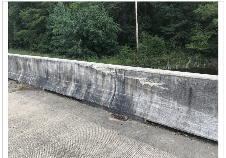
Left side span 6 spall.
