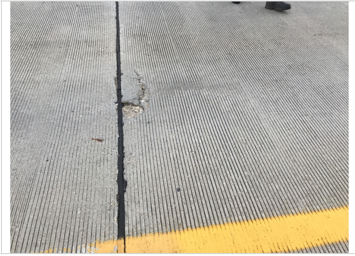
Span 3 bent 4 spall.
