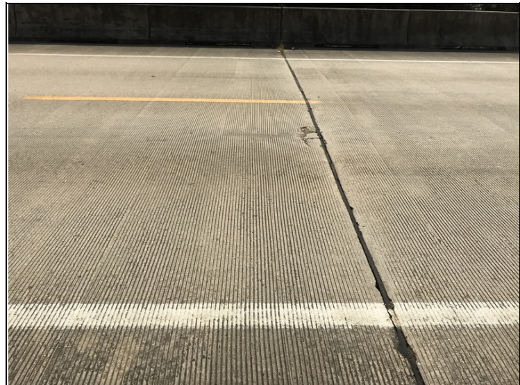
Spall at bent 4
