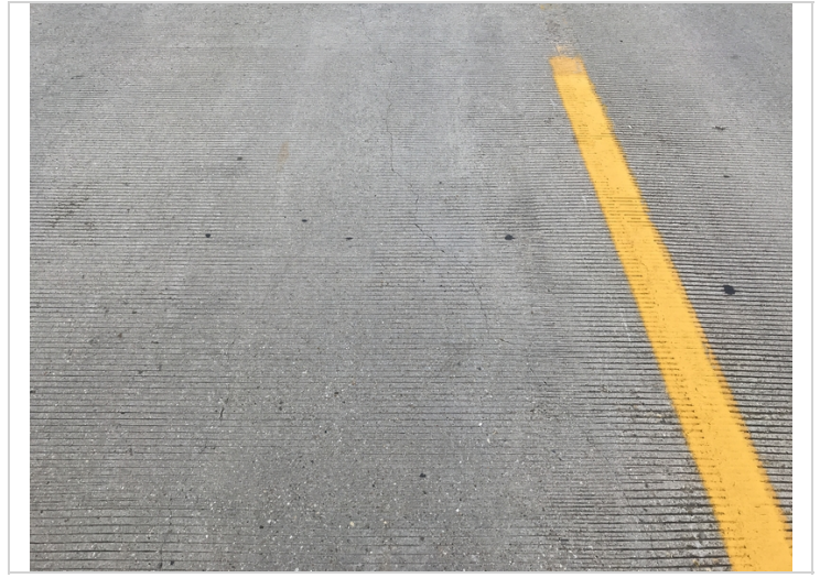
Span 1 longitudinal crack, max 0.030.
