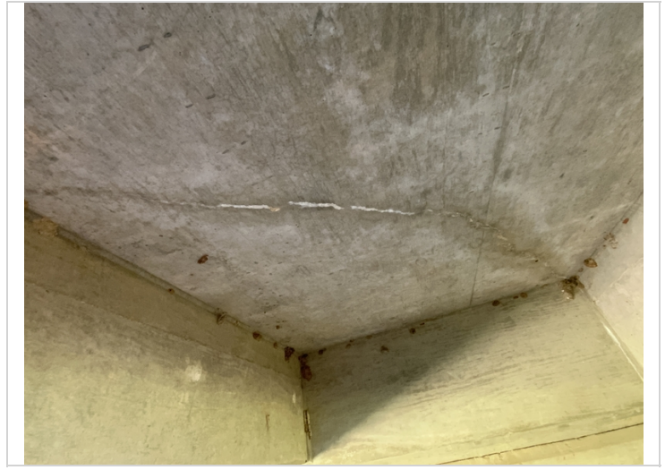
Span 1 soffit cracks with efflorescence.
