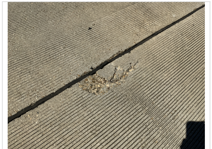
Span 3 at bent 4 spall in deck.
