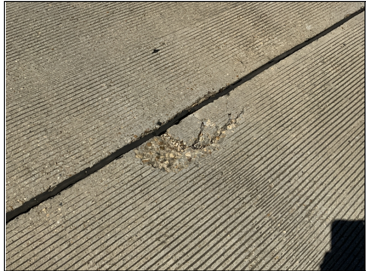
Span 3 at bent 4 spall in deck.
