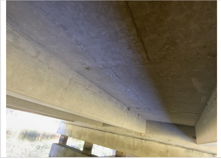
Span 3 soffit has cracks with efflorescence.
