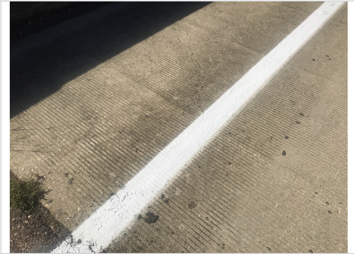
Span 1, diagonal crack.
