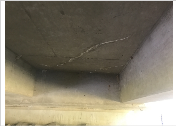
Span 3, cracks with efflorescence.
