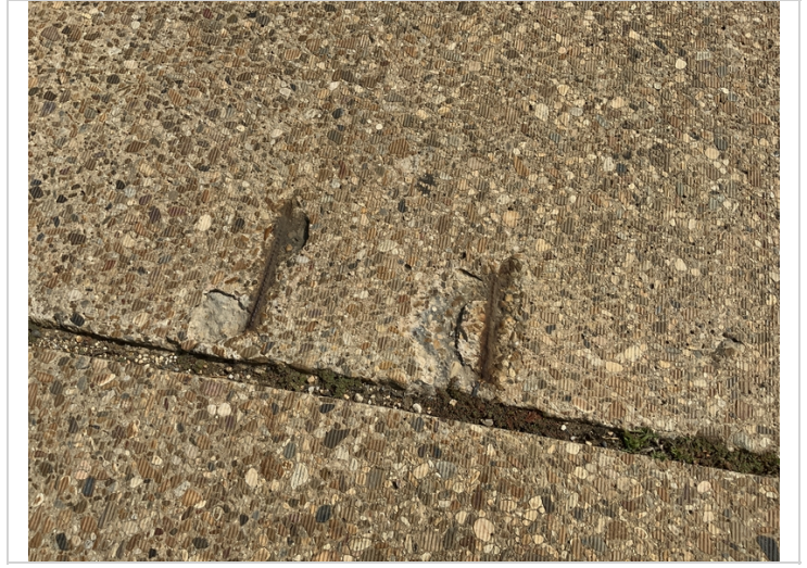
Deck span 7 at bent 8 exposed rebar in the deck.
