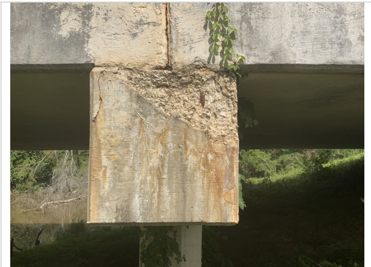
Bent 2 cap left side spall with exposed rebar.
