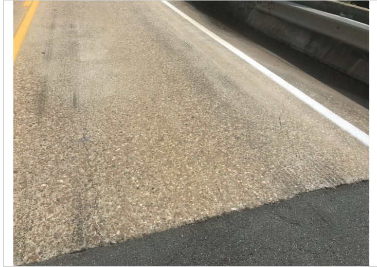
Span 9, longitudinal and diagonal cracks .
