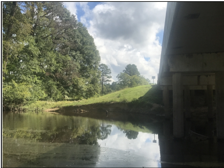
Spans 1 and 2, right of structure, slope erosion.
