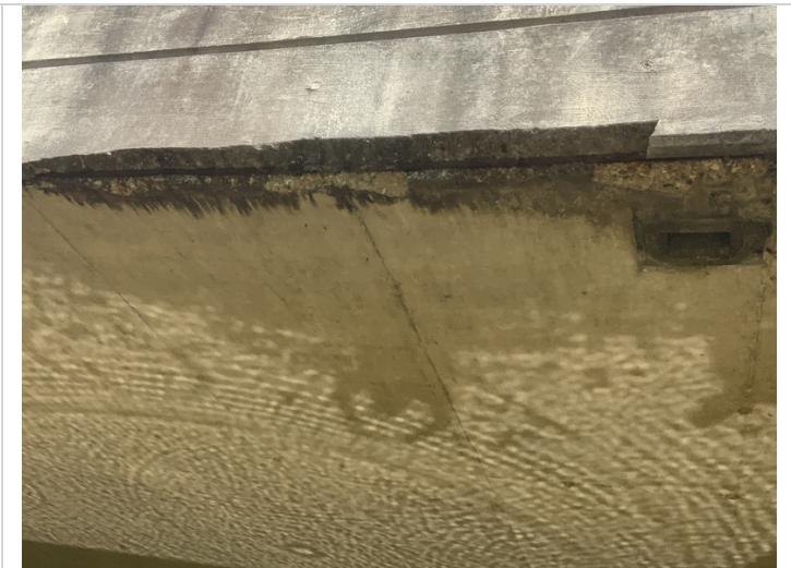
Span 4 soffit left side exposed rebar.
