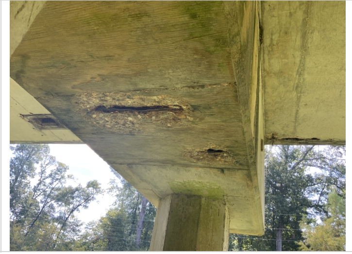
Bent 8 cap bottom has spalls with exposed rebar.
