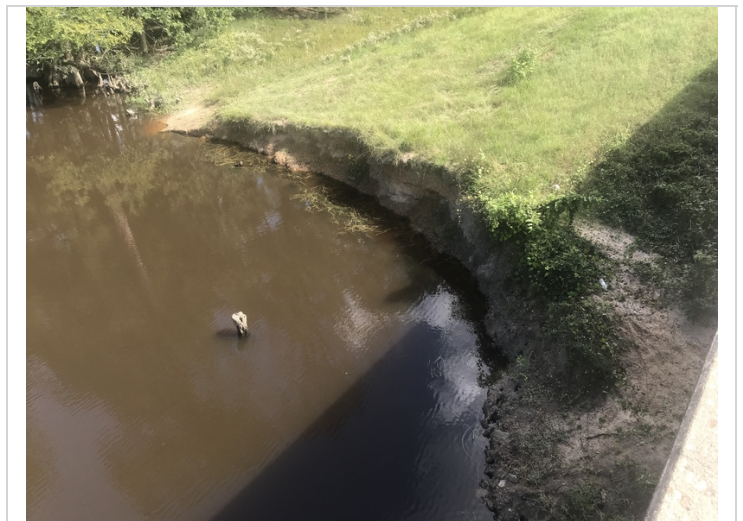
Overview of active slope erosion, 5 foot deep by 50 long.
