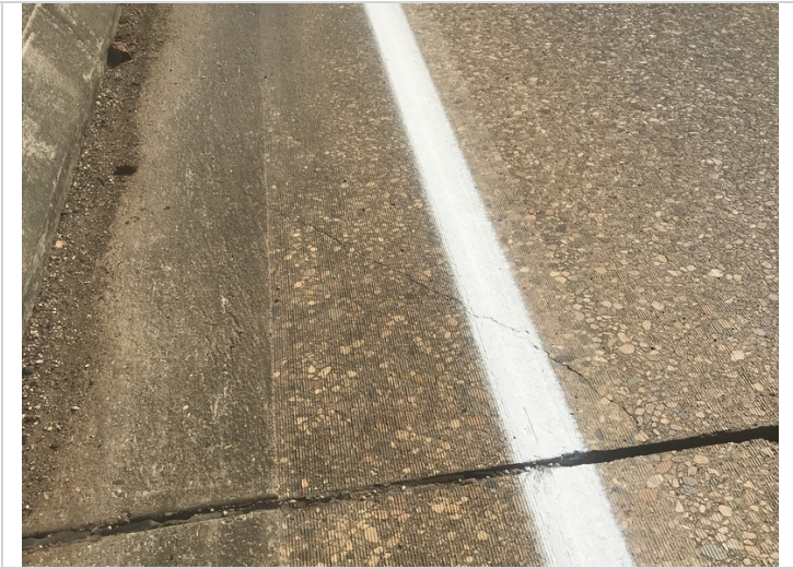
Span 1 diagonal crack
