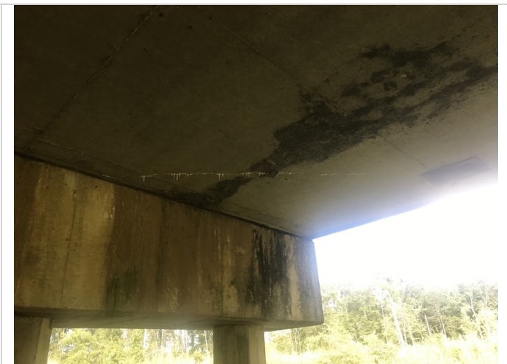
Span 7, crack with efflorescence.
