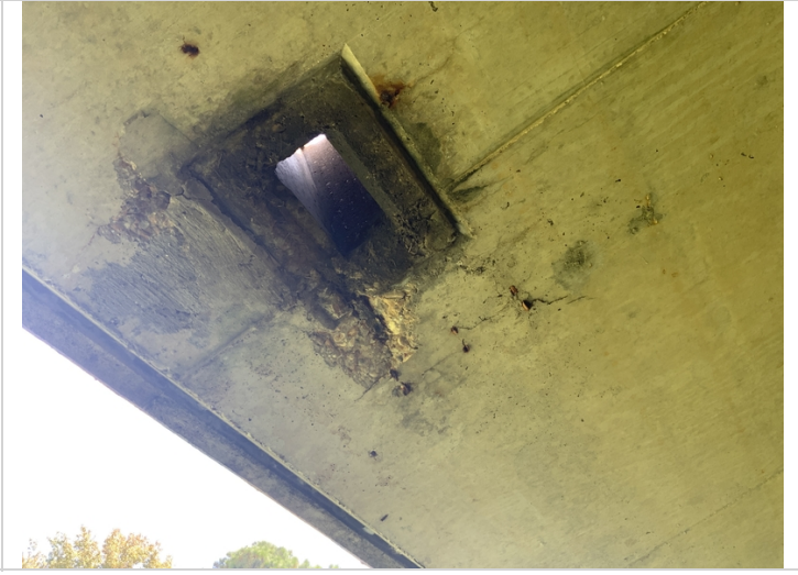
Span 7 soffit has exposed rebar.
