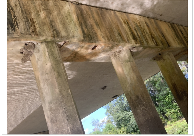
Bent 4 cap bottom has spalls with exposed rebar.
