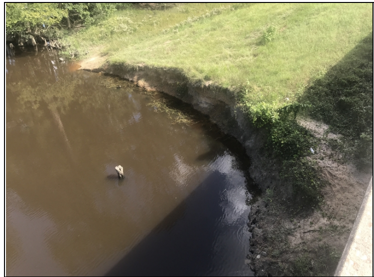
Overview of active slope erosion, 5 foot deep by 50 long.
