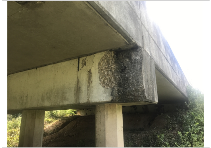
Right side bent 9 cap spall with exposed rebar.
