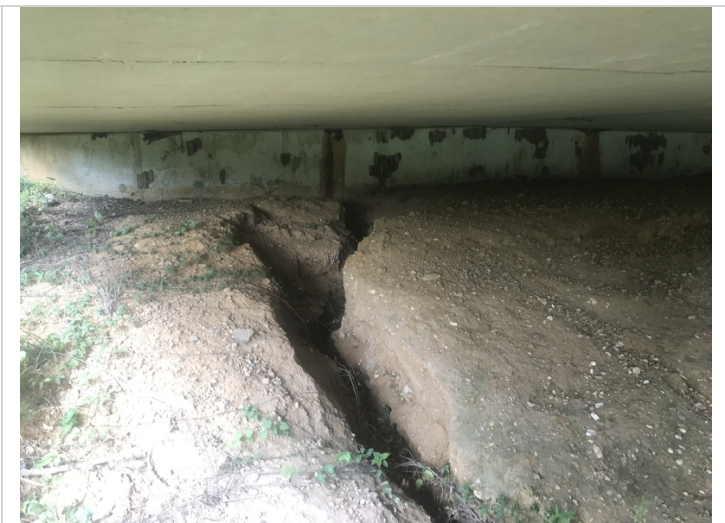
Abutment 10, minor slope erosion.
