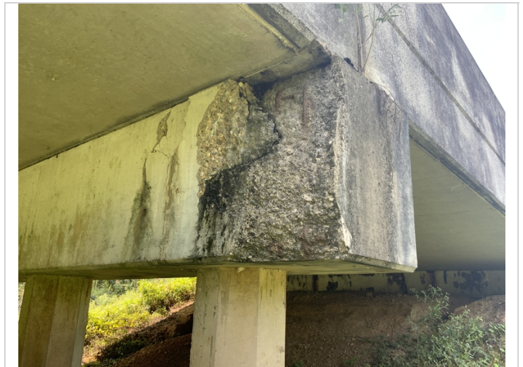
Bent 9 cap right side spall with exposed rebar.
