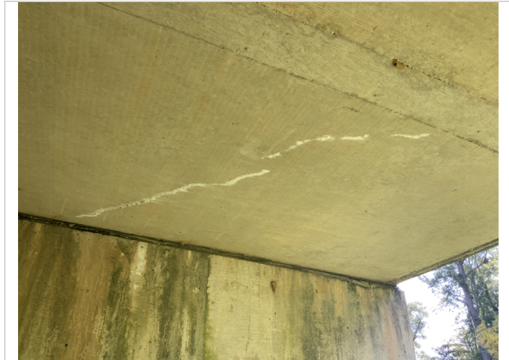
Span 9 soffit has cracks with efflorescence.
