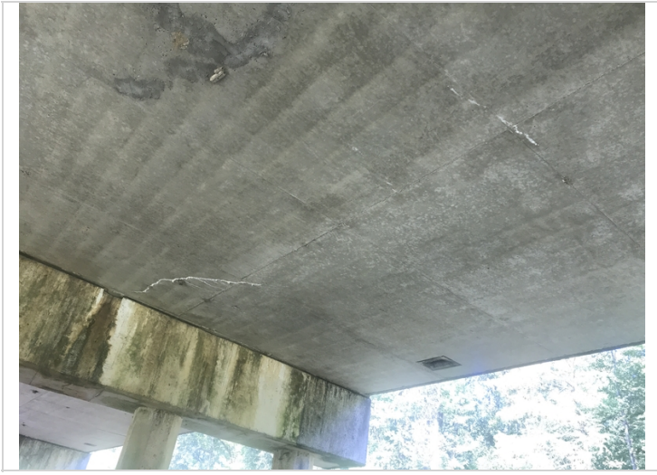
Soffit span 5, crack with efflorescence.
