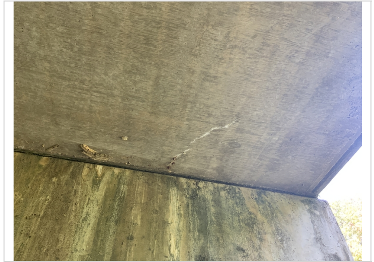
Span 1 cracks with efflorescence.
