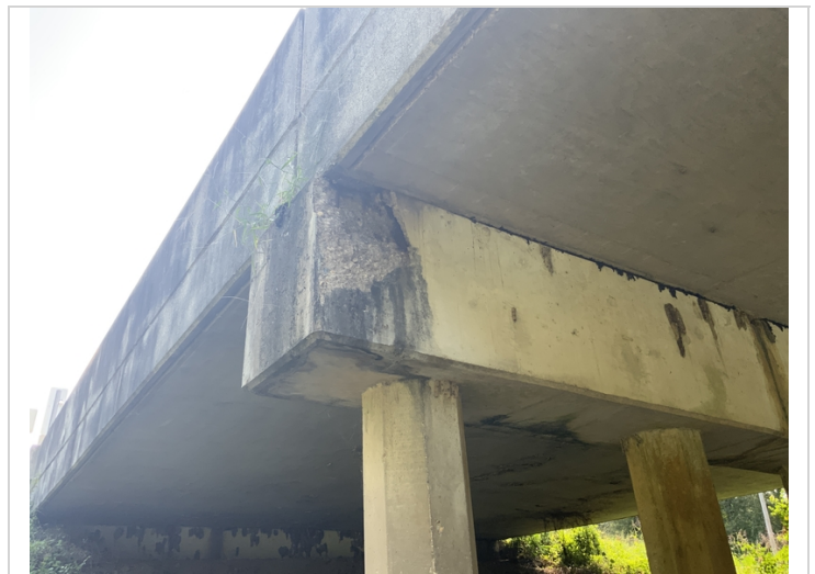
Bent 2 cap ahead spall right side.
