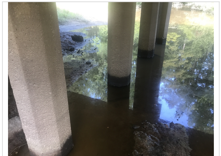
Piles at bent 7, light abrasion.
