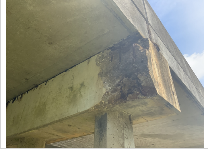
Bent 3 cap ahead left side large spall with exposed rebar.
