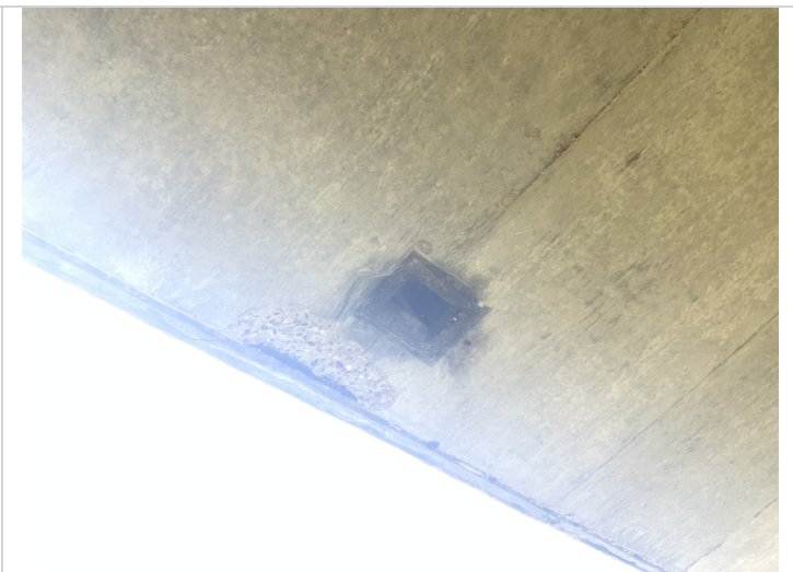
Span 1 soffit has exposed rebar.
