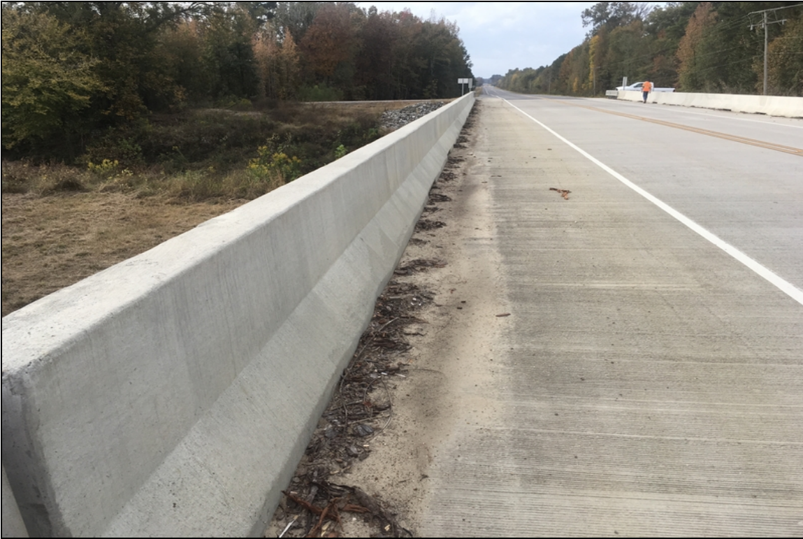
Dirt and debris in gutter.
