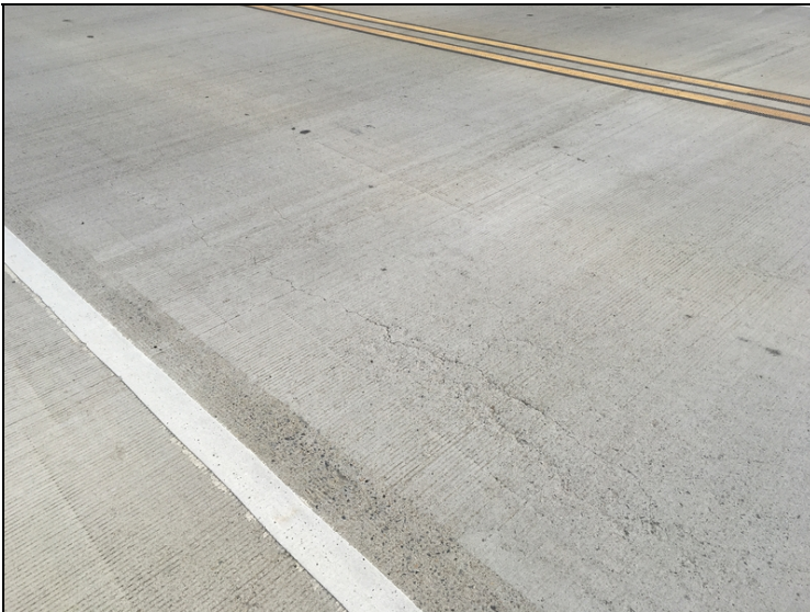
Span #1 sealable deck cracks
