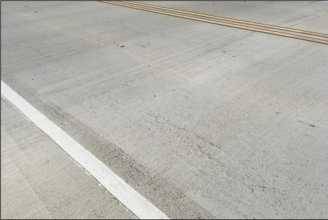
Span #1 sealable deck cracks
