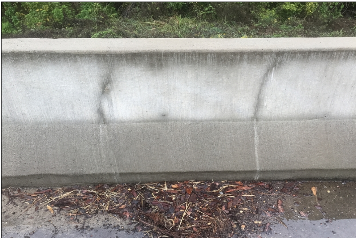
Parapet wall Vertical cracks
