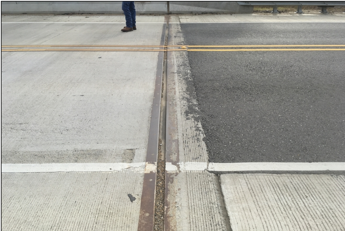
Bent #1 Joint good condition.
