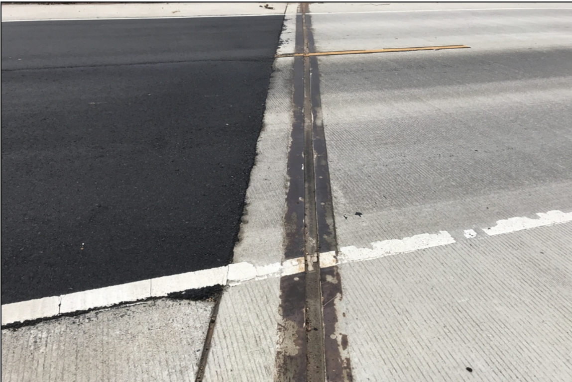
Joint material at abutment 1
