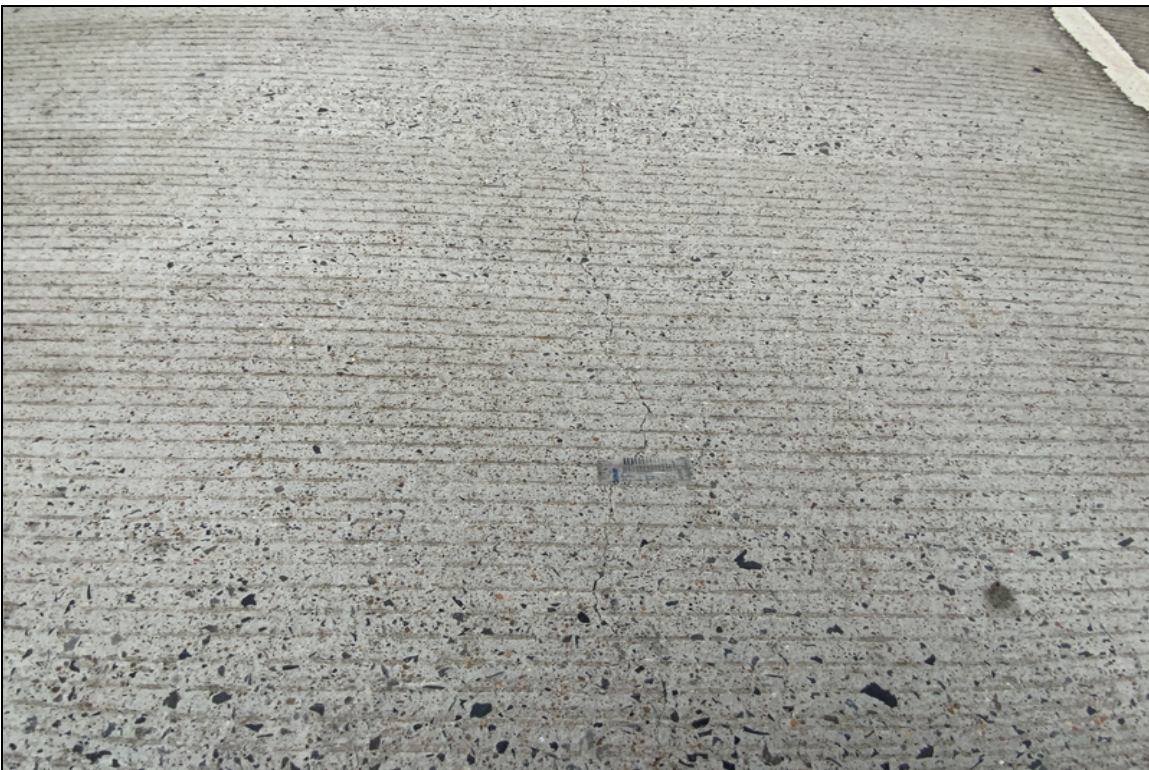
Longitudinal deck cracks 0.025
