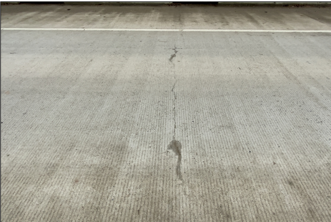
Transverse deck cracks 0.030
