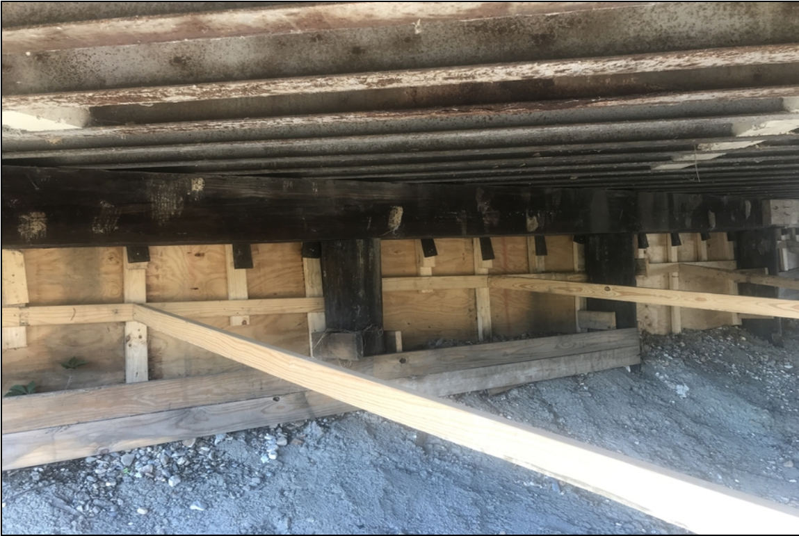
Abutment 1 back-wall repaired.
