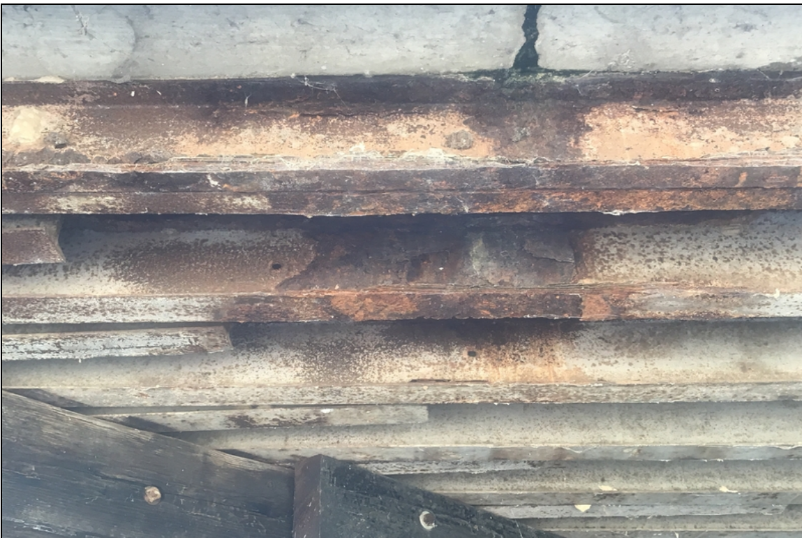
Girders with corrosion, span 2, girders 2-4.
