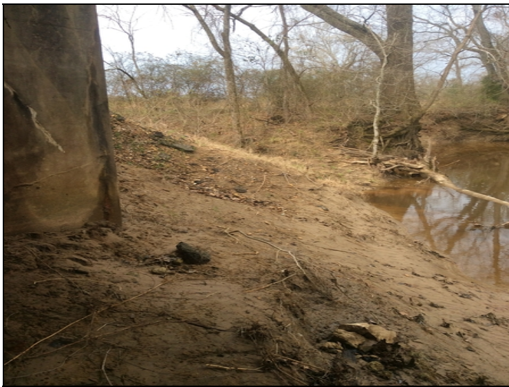
Erosion abutment 1 left side.
