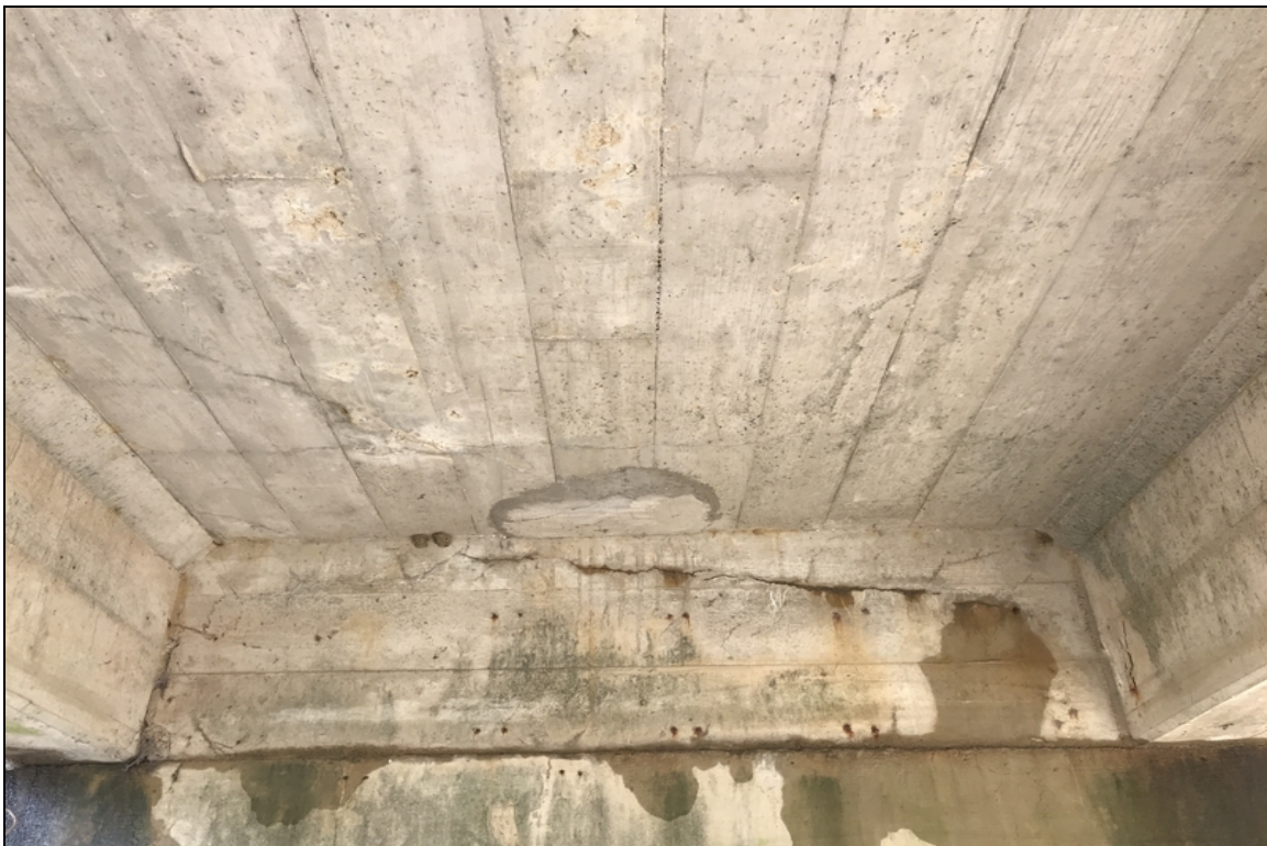
Span 3, bay 1, small cracks.
