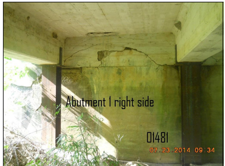
Abutment 1 Rt., cracks in diaphragm between girders 2 & 3.
