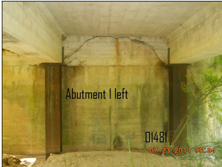
Abutment 1 Lt. cracks in diaphragm between girders 1 & 2.
