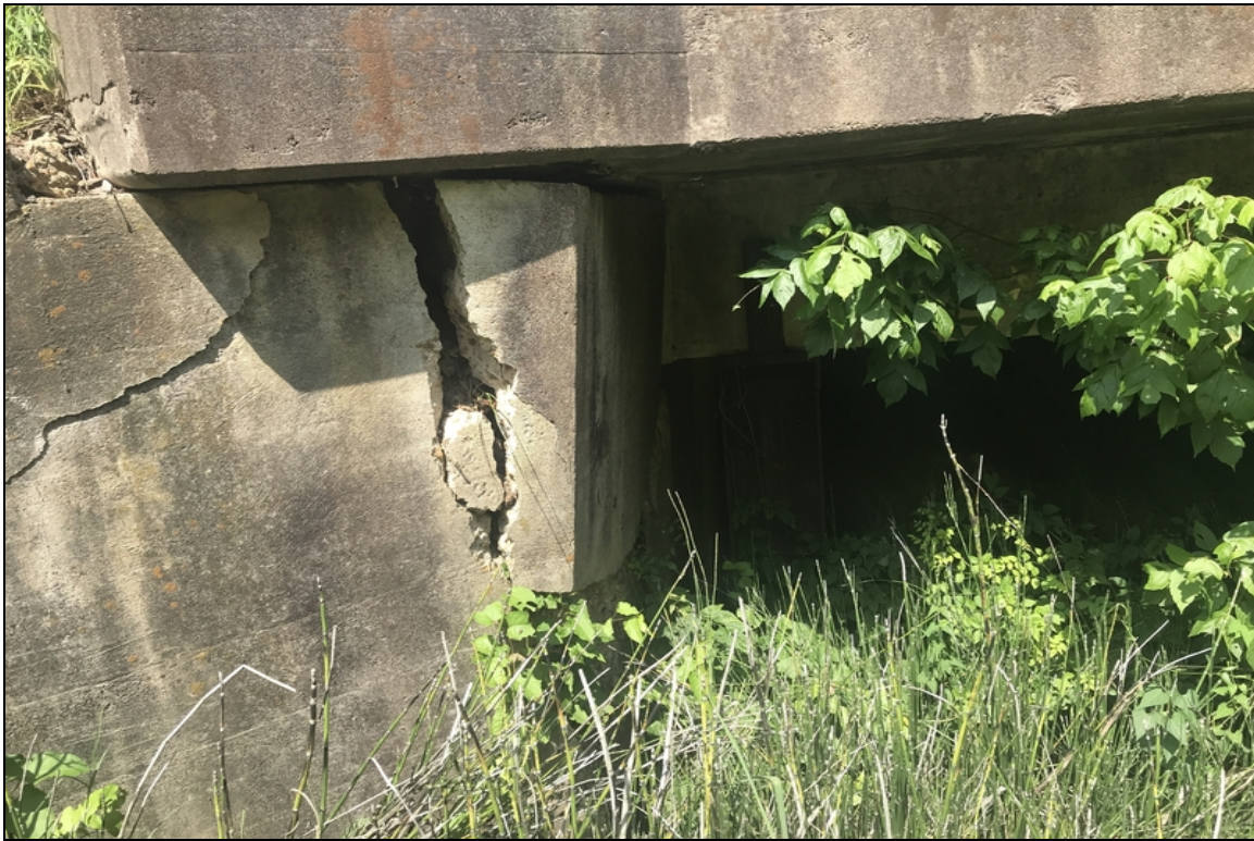
Abutment 1 right side, back wall has large delam
