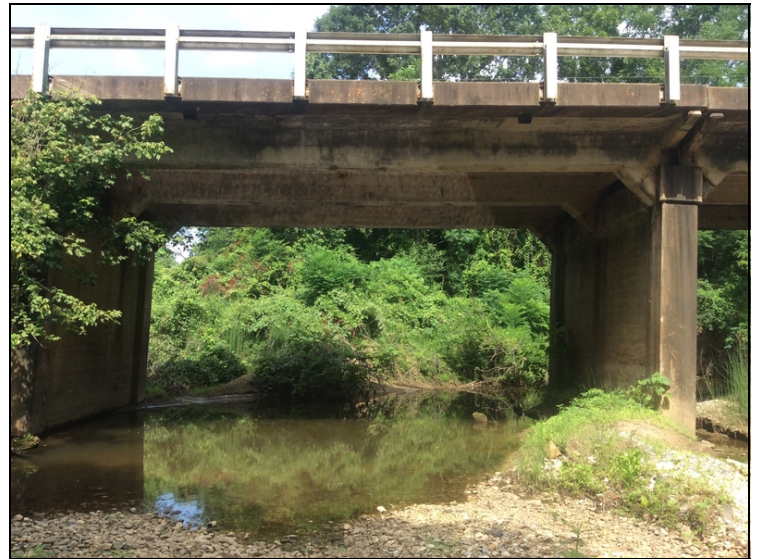
01481 main span, both bents 2 & 3 have rotated ahead.
