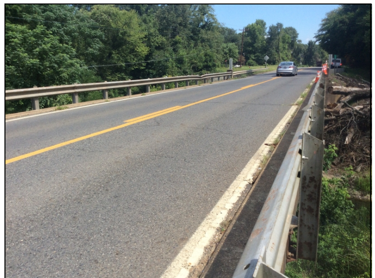
Span 3, minor damage to guardrail on the Rt. side
