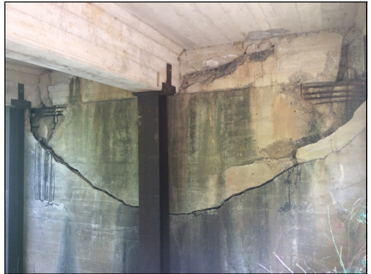
Abutment 2 pier wall has a large crack & spalls & the middle upper section between girders 1 & 3 have shifted ahead thus exposing some of the reinforcing steel.
