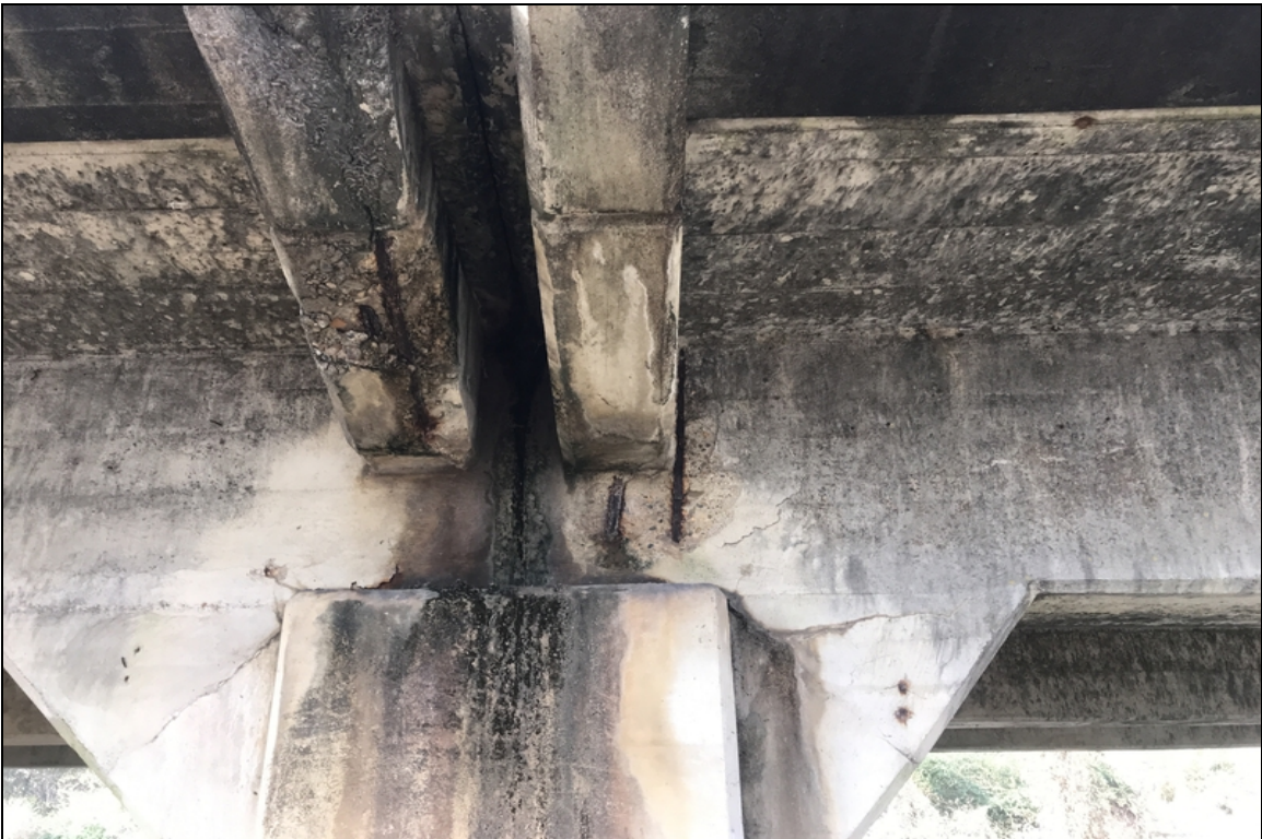
Span 3 girder 3, exposed rebar at bent 3.
