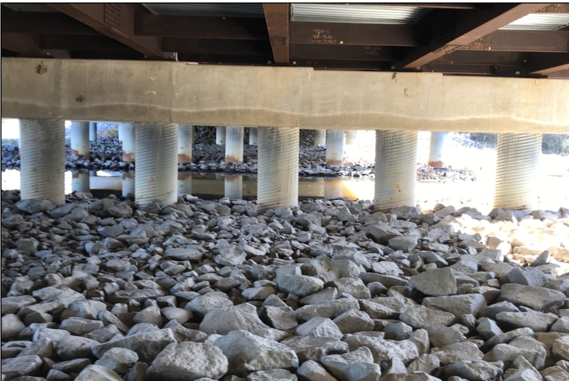
Bent 4 in casement beginning to rust
