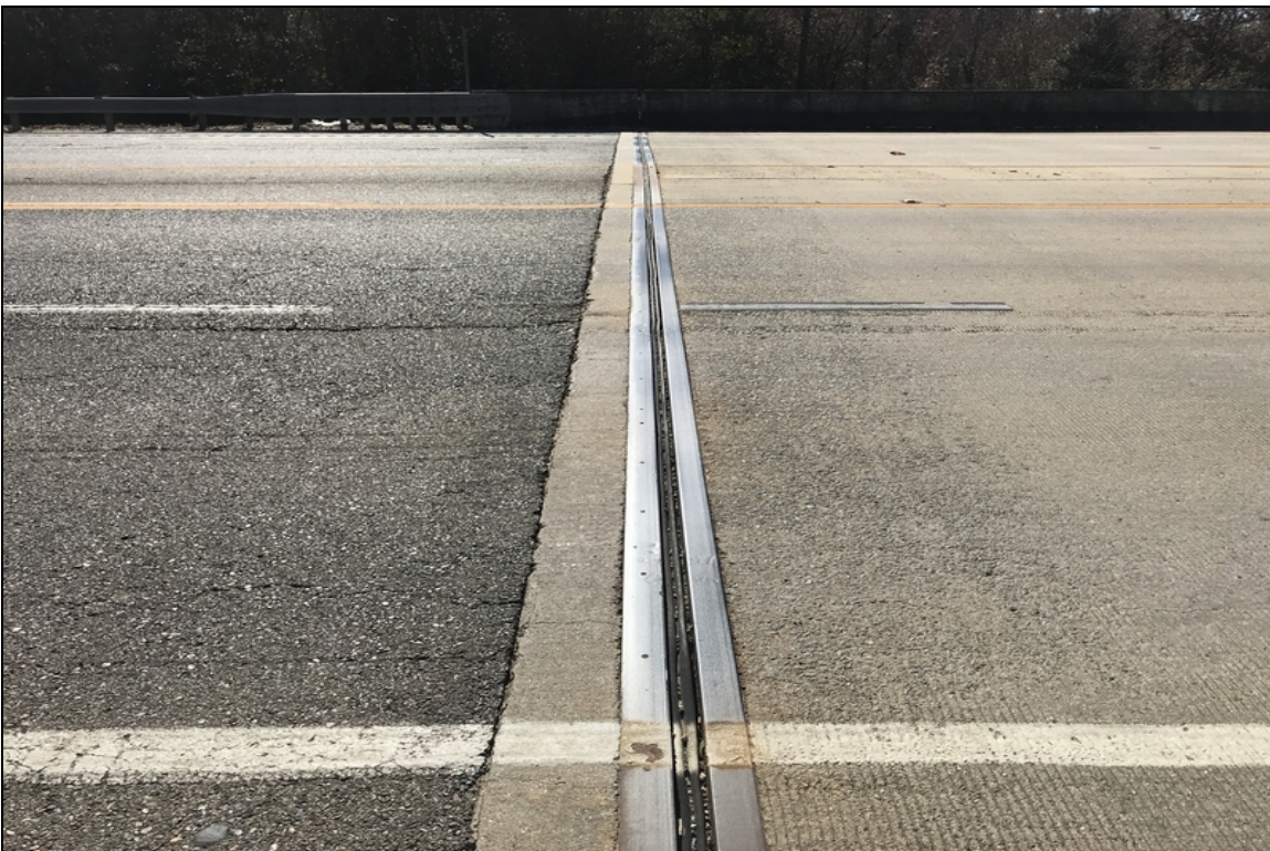
Abutment 2 joint material.
