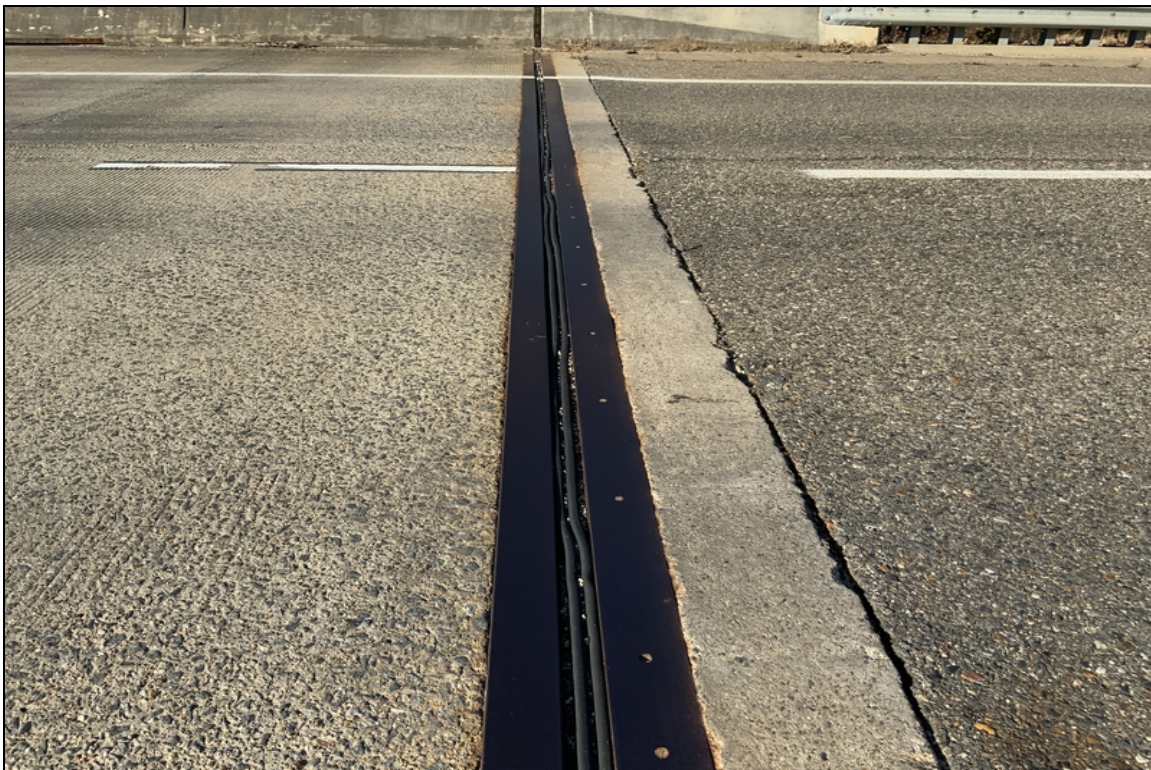
Bent 6 joint seal has lost adhesion and is leaking.
