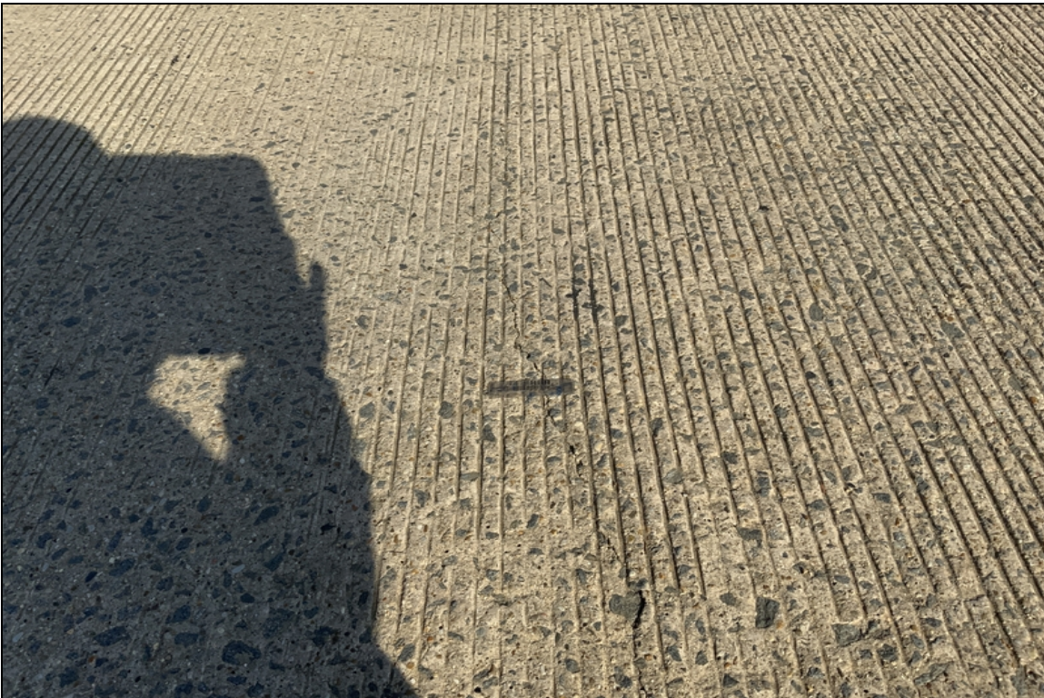
Span 7, transverse deck cracks 0.040
