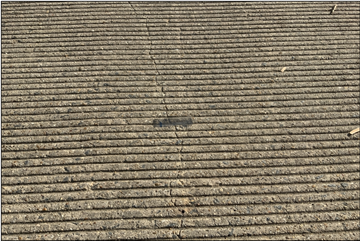
Span 6 deck crack, max 0.040
