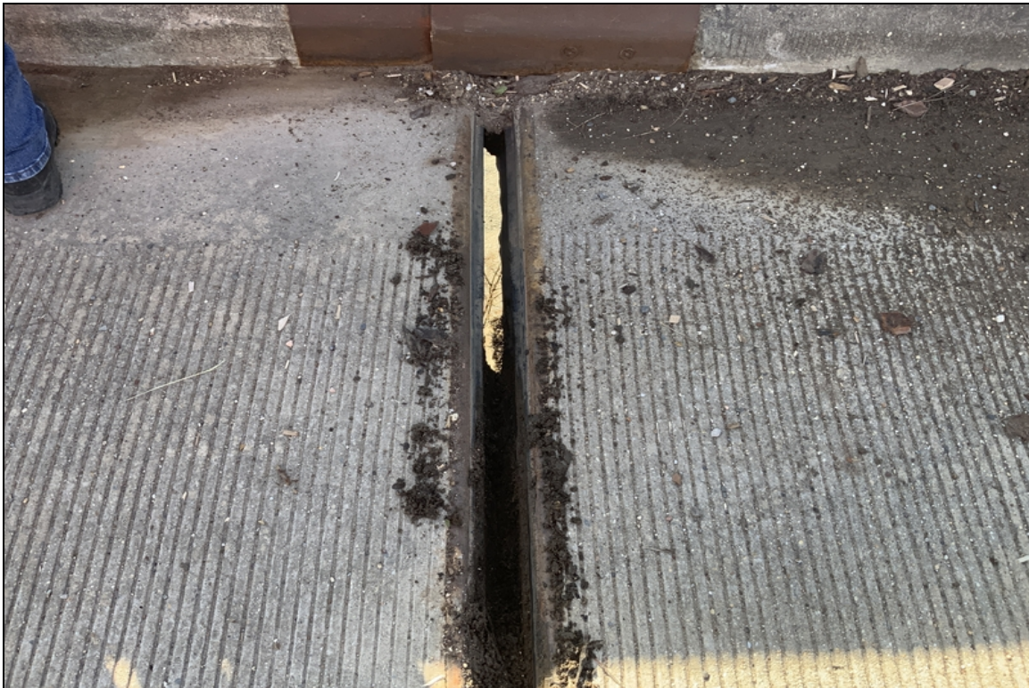
Bent 5 joint missing end, approx 2 feet
