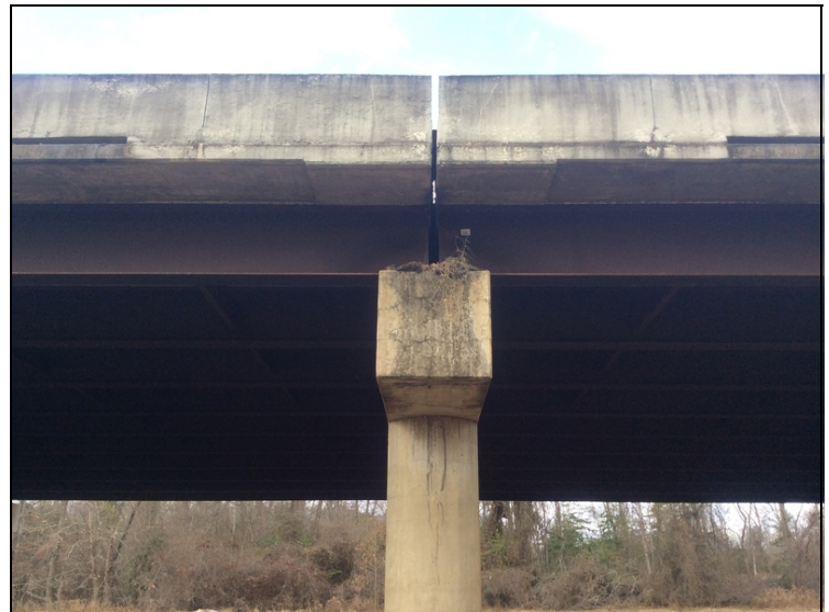
Bent 12 Rt. side, large hole in joint material approx. 1 1/2' long & 3/4" - 1" wide, allowing dirt, debris, & road salts to get through to girder ends & top of caps.
