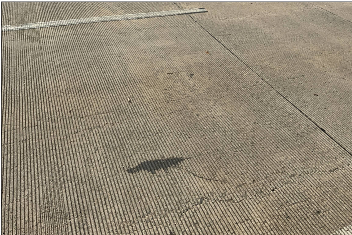
Span 6 map cracks
