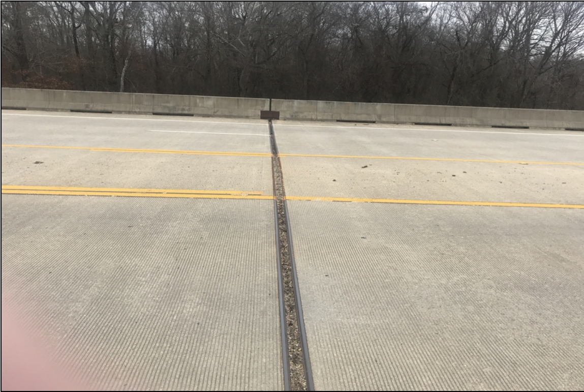
Joint between span 1 and 2. Dirt and debris.
