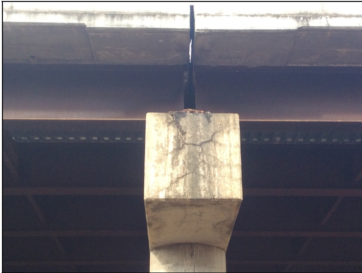
Bent 24 pier cap on Rt. end has several cracks from leaks in joint material above the cracks.
