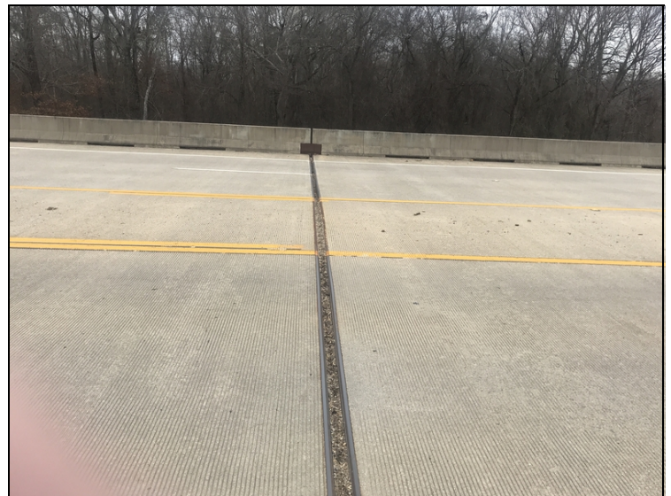
Joint between span 1 and 2. Dirt and debris.
