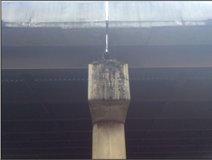
Bent 24 Lt. side large crack in joint material approx. 2 1/2' long & 1" wide, allowing dirt, debris, & road salts to get through to girder ends & top of cap.
