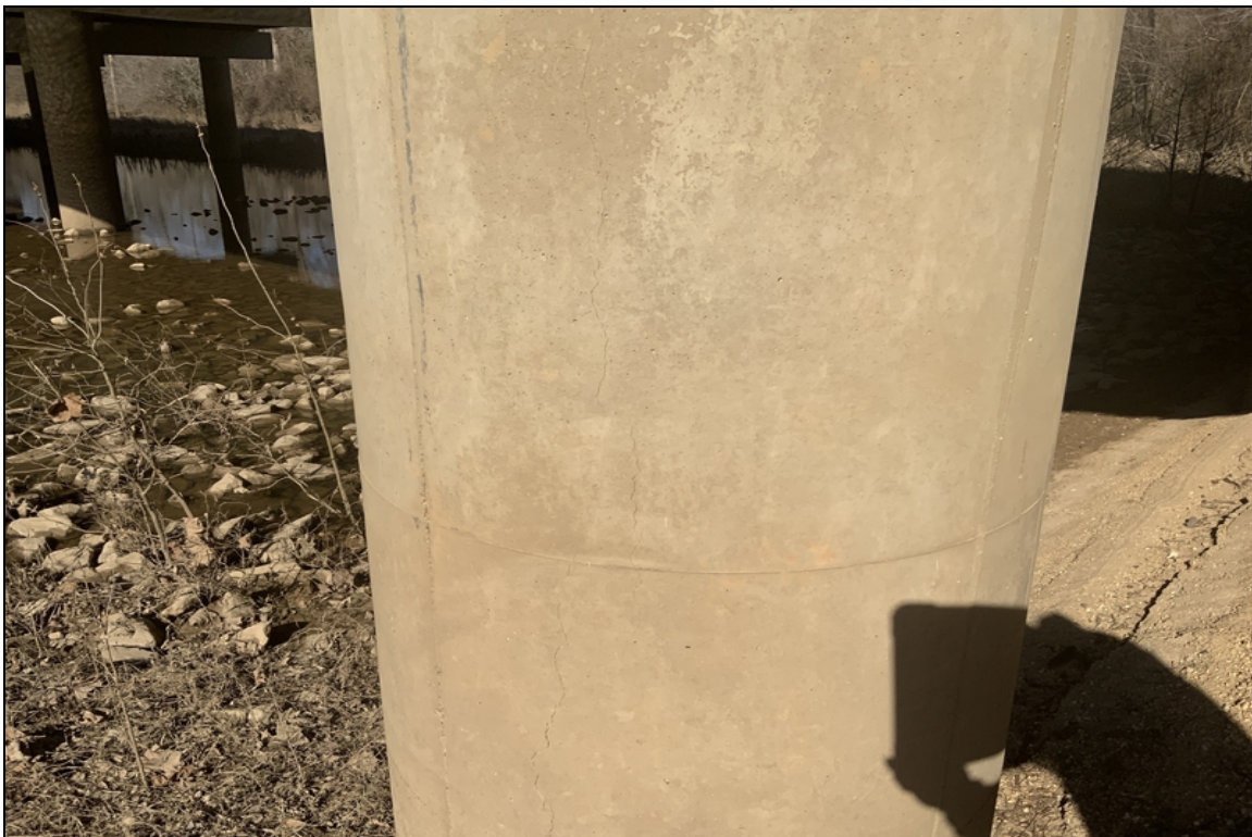
Bent 27 column 4, vertical cracks, 0.030
