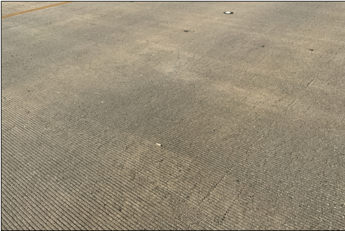
Span 5 map cracks
