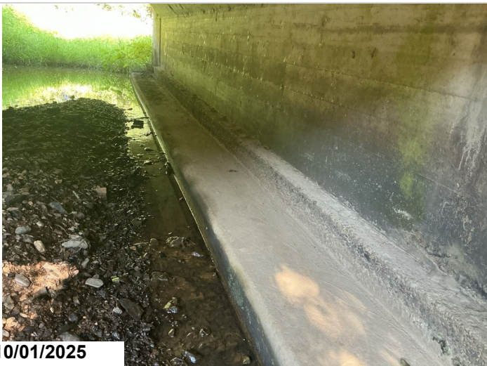
Bent 2: footing is exposed and the countermeasure is working as intended.
