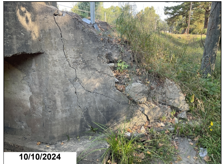
Right wing wall at bent 2 is damaged from traffic impact. 2024
