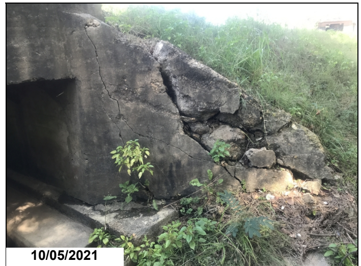
Right side at bent 2, damage to wing wall.
