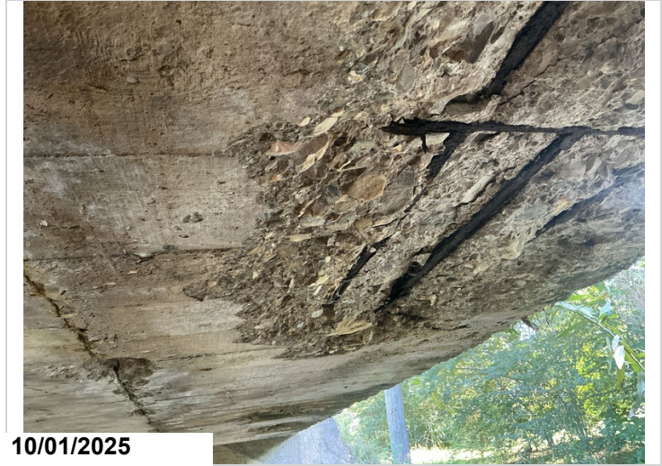
The undersurface has multiple large spalls with exposed rebar that has measurable section loss. CS3- 18sf of spalling, CS3-16' delam
