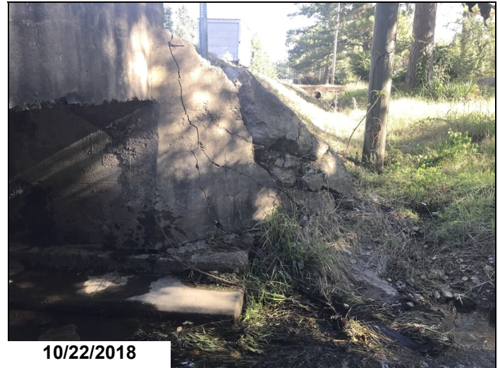
Right wing wall at bent 2 damaged from traffic impact
