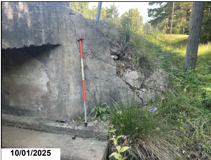
Right wing wall at bent 2 is damaged from traffic impact. 2025
