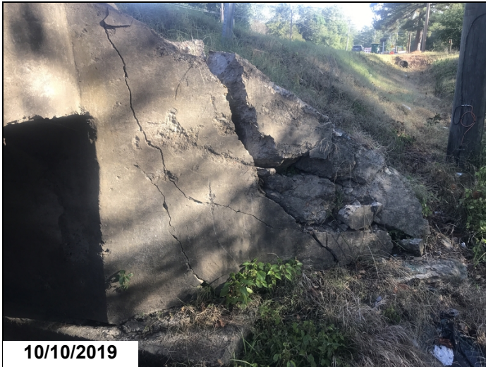
Right wing wall at bent 2 is damaged from traffic impact
