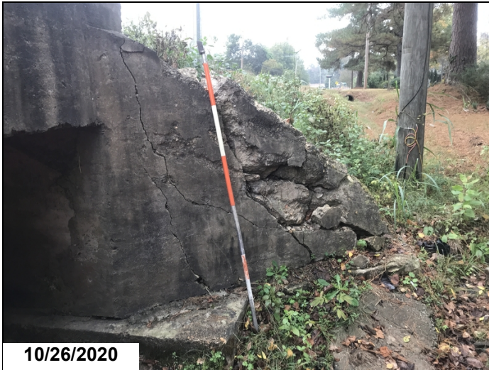
Southeast wing wall impact damage
