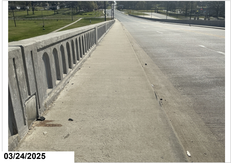
The sidewalk has numerous unsealed transverse cracks at an average of 4 foot spacing. This is common to the opposite sidewalk.
