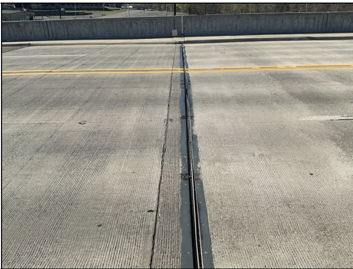
Bent 6: joint seal full of debris.
