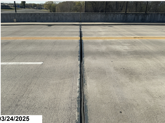
Bent 4: joint seal has fallen at the middle 2 lanes. CS4-20'
