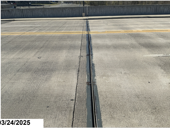
Bent 6: joint seal full of debris.
