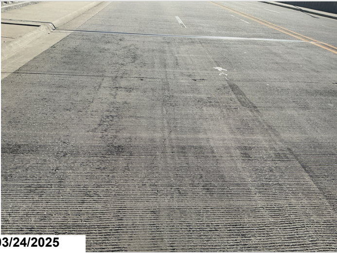
West approach slab with large longitudinal cracking.
