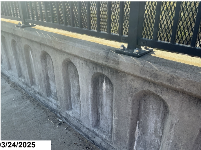
Right rail with numerous vertical cracks with efflorescence staining.
