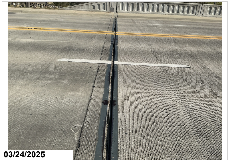
Bent 1: joint seal is full of debris.
