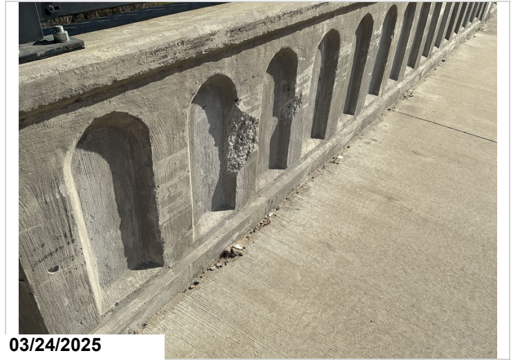
Span 2, left rail: spall due to vehicle impact. CS3-2'
