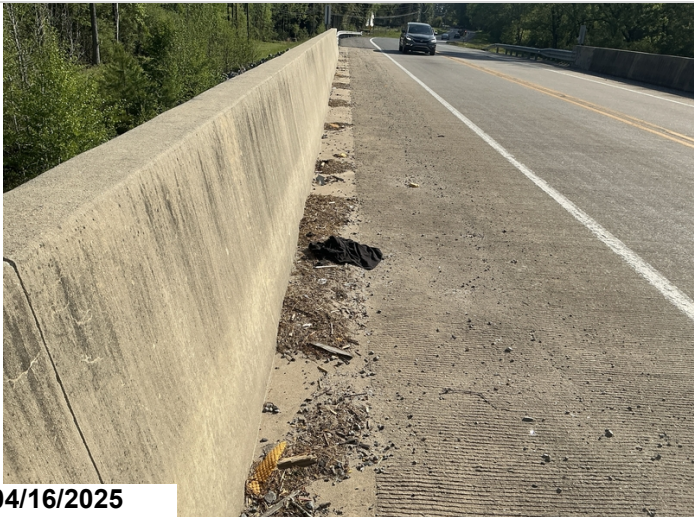
Gutterline full of debris
