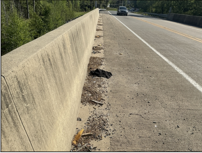
Gutterline full of debris
