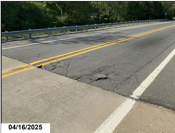
The south approaching pavement with a couple of pot holes.
