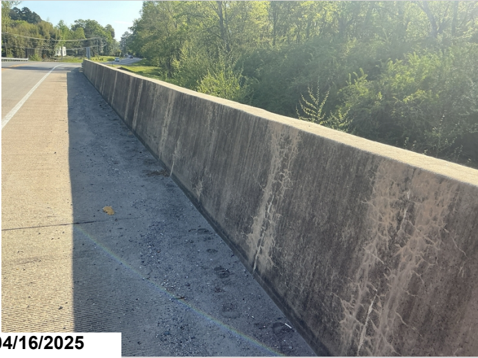
Right concrete railing with numerous vertical cracks at a 4' spacing.
