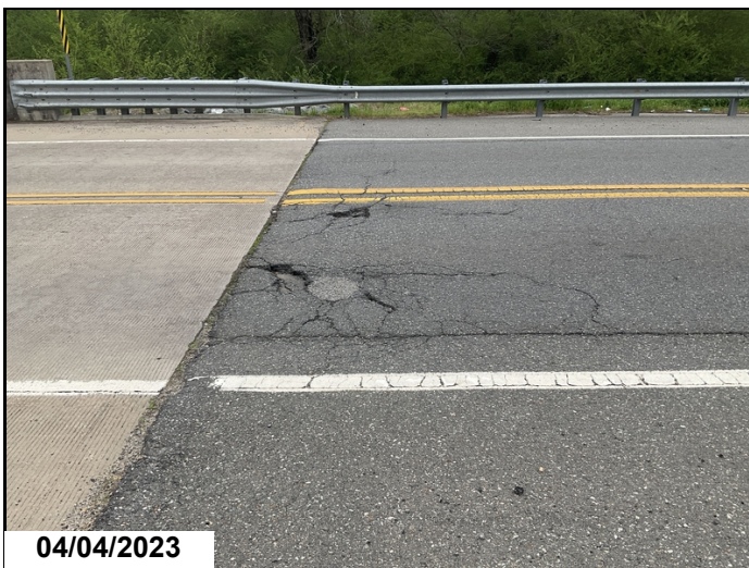
South asphalt roadway pot holes in the approach roadway
