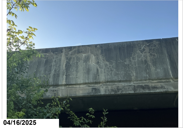
Span 1: left rail with large section of map cracking and efflorescence staining.
