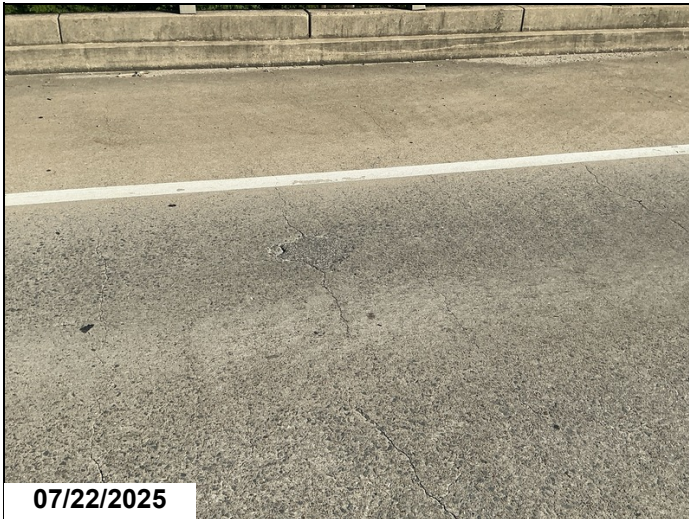
Span 2: spall that has been patched with asphalt.
