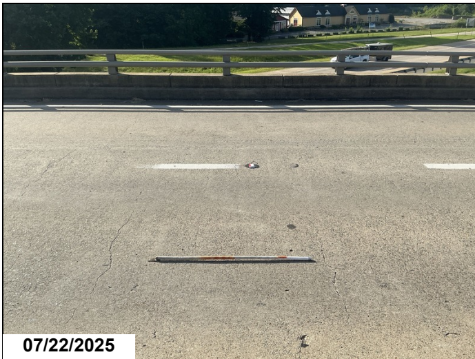
Span 2: the deck with numerous unsealed transverse cracks at a 2' spacing and up to 0.060" in width.
