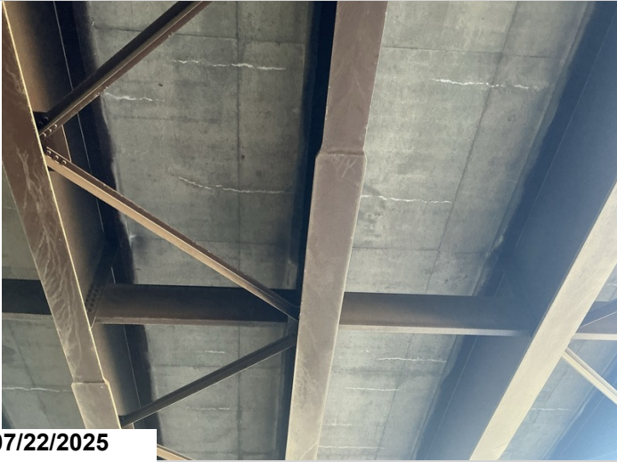
Span 3: deck cracking reflecting through to the undersurface with efflorescence staining.
