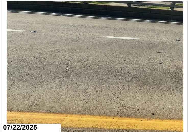
Span 1, northbound side: large unsealed transverse cracks up to 0.060" in width.
