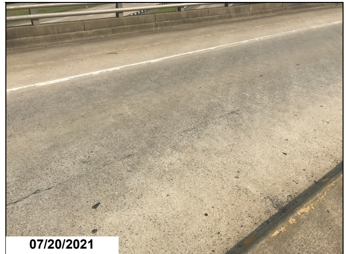
Deck cracks
