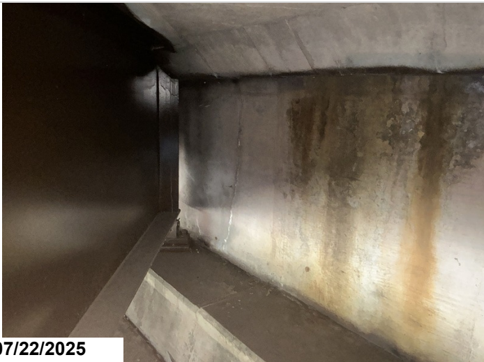
Bent 1: vertical crack with efflorescence staining common to both backwalls.
