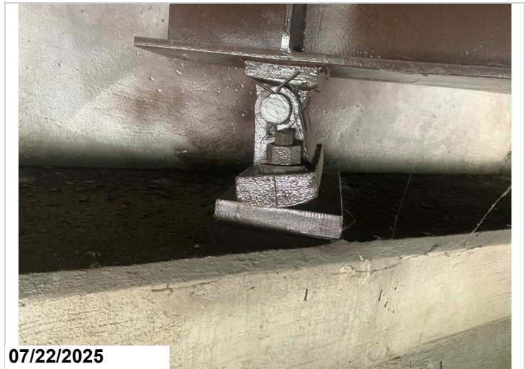
Bent 5: general condition of the bearings are good. All bearings at this bent are rotated back.
