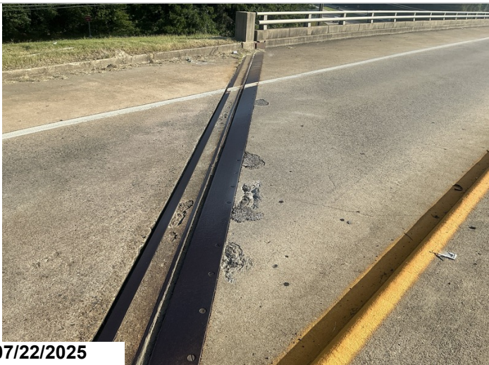
Span 1: multiple spalls filled with asphalt adjacent to the joint. CS3-4
