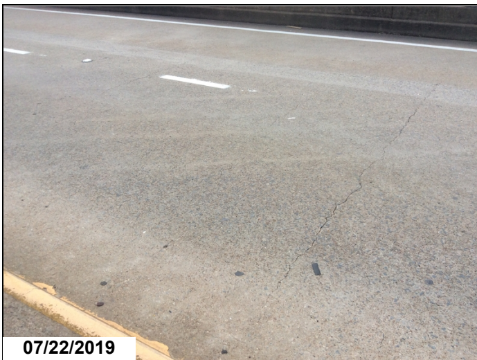
Span 1 large unsealed cracks up to 0.060"
