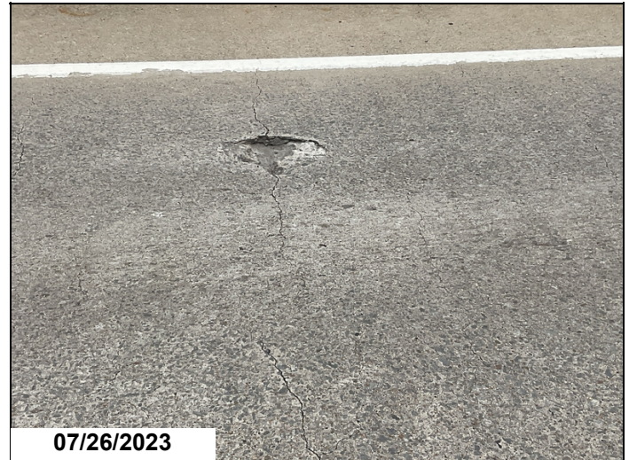
Span 2 deck south bound lane spall with exposed rebar.
