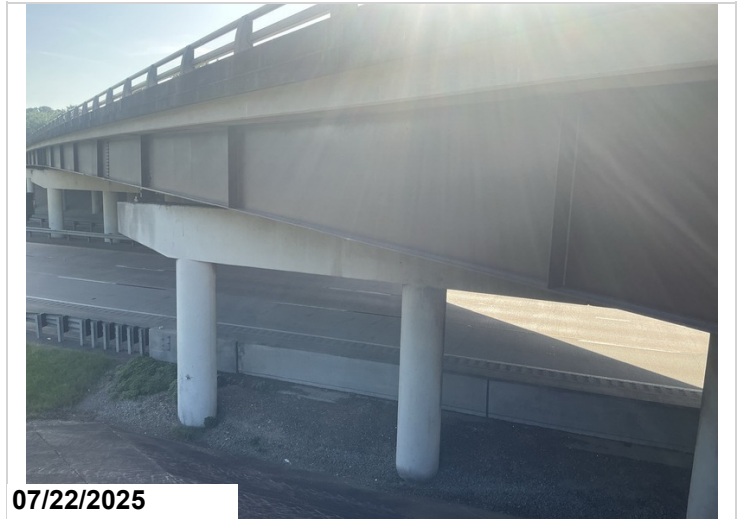
The steel protective coating is in good condition.
