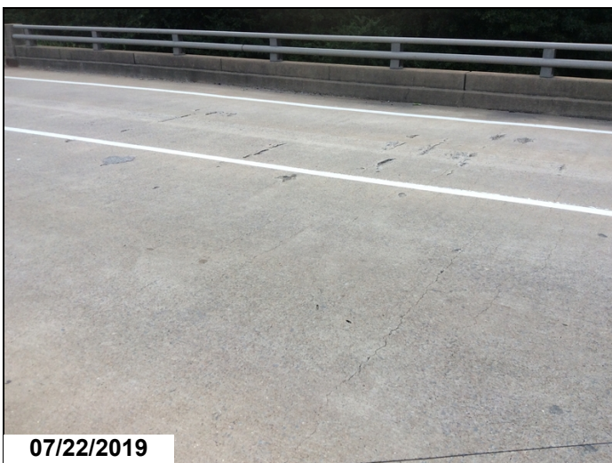
Span 4 northbound lanes spalls with exposed rebar
