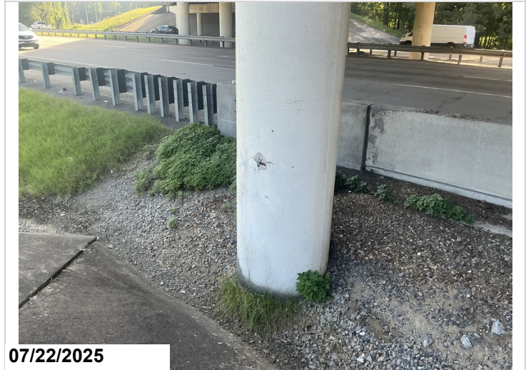
Bent 2, column 1: small spall with exposed rebar. CS3-1
