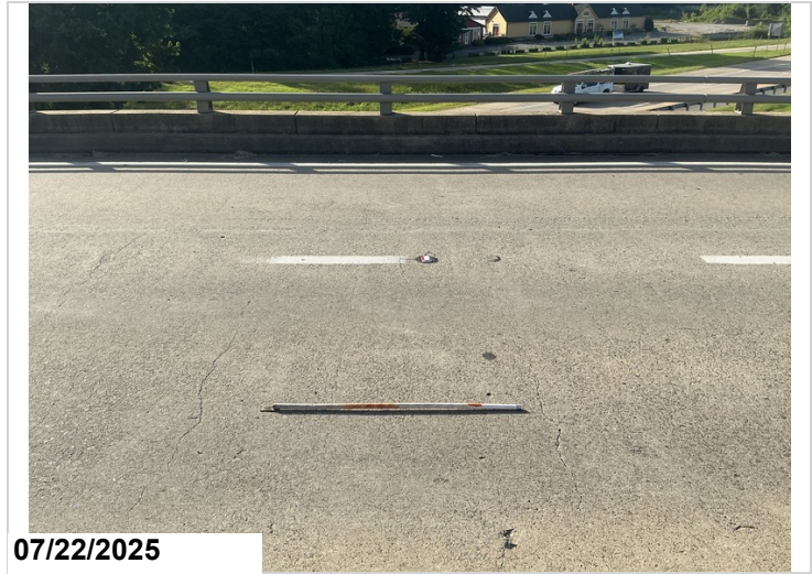
Span 2: the deck with numerous unsealed transverse cracks at a 2' spacing and up to 0.060" in width.
