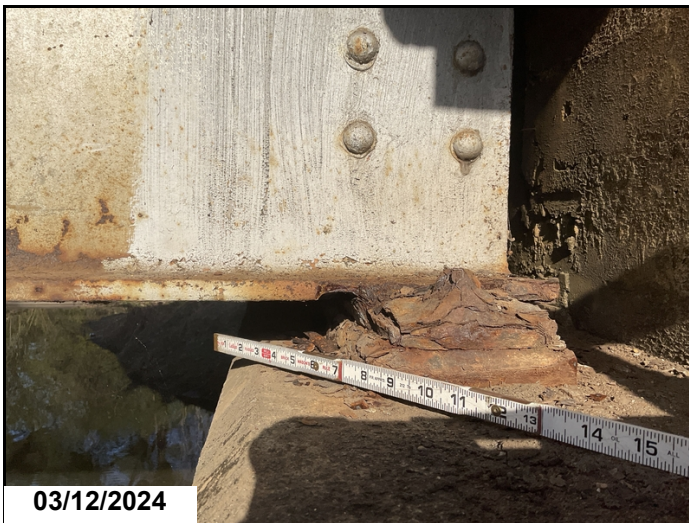
Span 3 Bent 4 girder 5 has 3/8" pitting to lower flange at bearing area.
