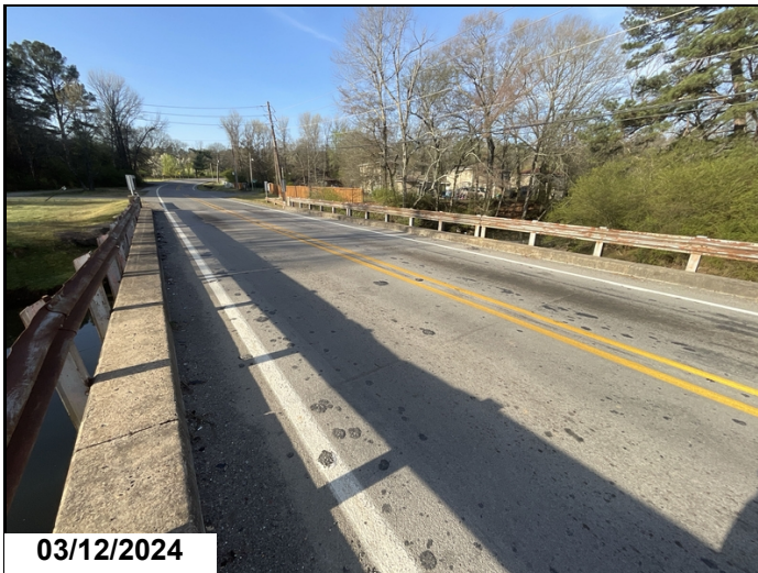
Cracks have been sealed with polymer overlay.
