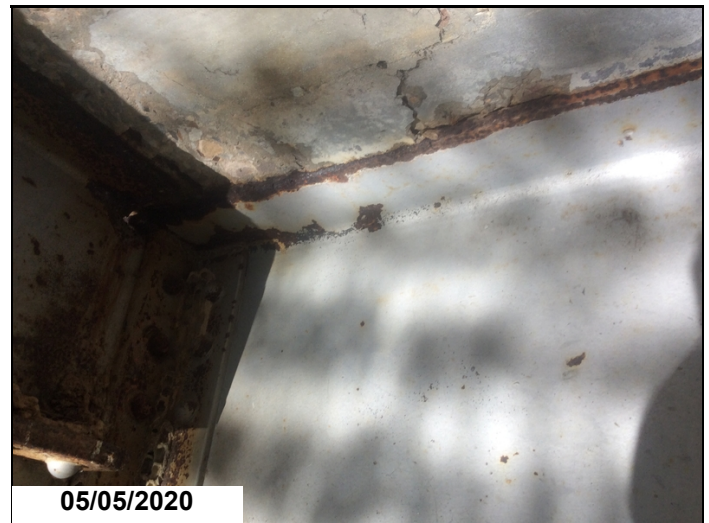
Span 3 beam 3 active rust to top flange at diaphragm mid span. Common all spans.
