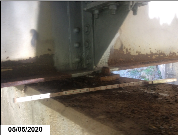
Bent 3 spans 2 and 3 active rust with pitting up to 1/8" deep to bottom flange and lower web. Common beams 1 thru 4.
