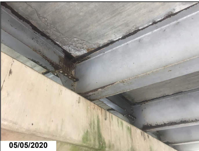
Bt. 3, corrosion on top & bottom flange.
