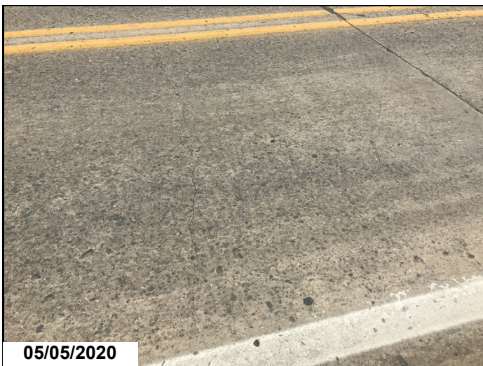
Span 3 large unsealed cracks and abrasion. Up to 0.040".
