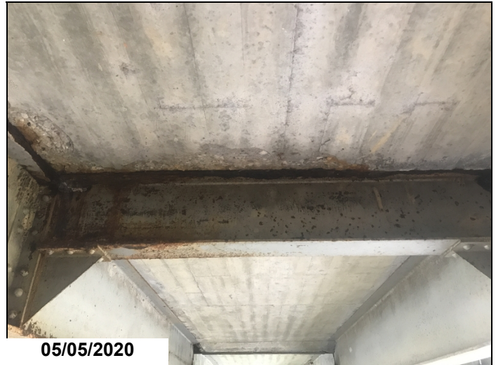
Span 1, diaphragm between Bm 3 & 4, top flange has corrosion.
