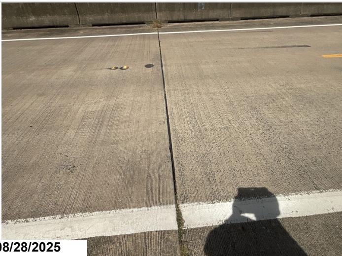
Bent 3, pourable joint seal: has lost adhesion. CS2-34'
