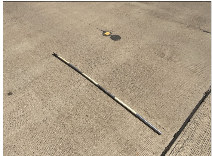
Bent 4, span 4: cracking. CS2- 7'
