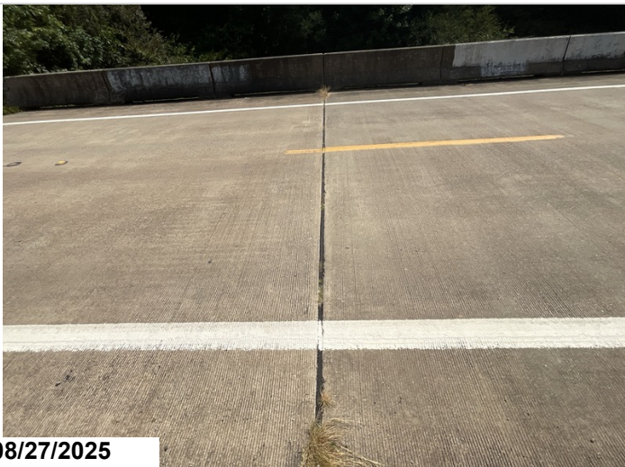
Bent 5, pourable joint seal: has lost adhesion. CS2-34'
