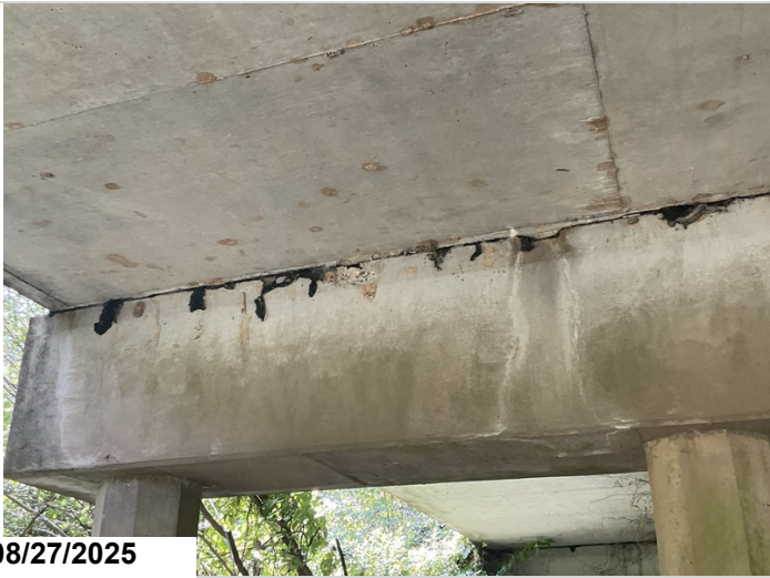
Bent 2, ahead side, between piles 1 & 2: small spall. CS2-1'
