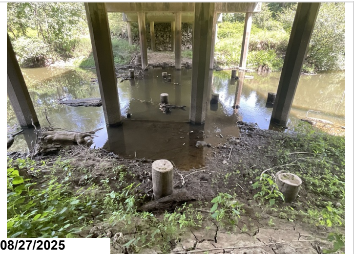
Bent 3: all pile have abrasion. CS2- 4 ea
