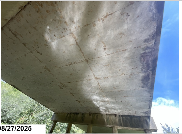
Span 3: insignificant hairline map cracking throughout the entire span.
