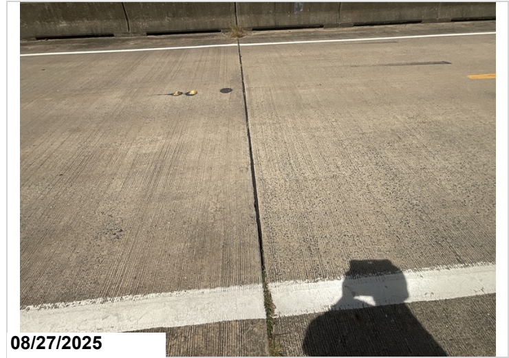
Bent 3, pourable joint seal: has lost adhesion. CS2-34'
