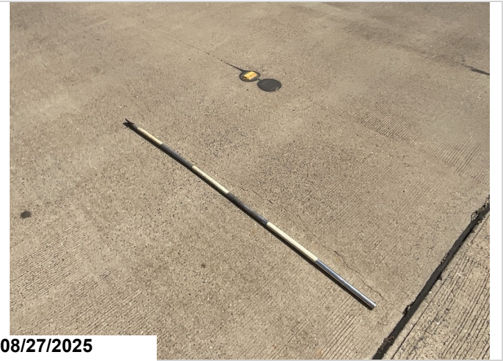
Bent 4, span 4: longitudinal cracking. CS2- 7'
