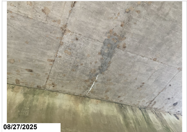
Span 4, at bent 4: cracking with efflorescence staining. CS2-2'
