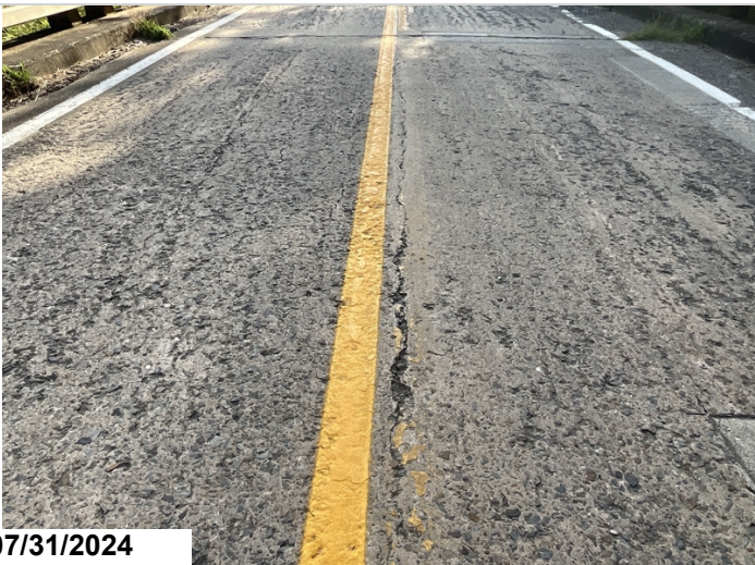
Span 2 longitudinal crack at centerline.
