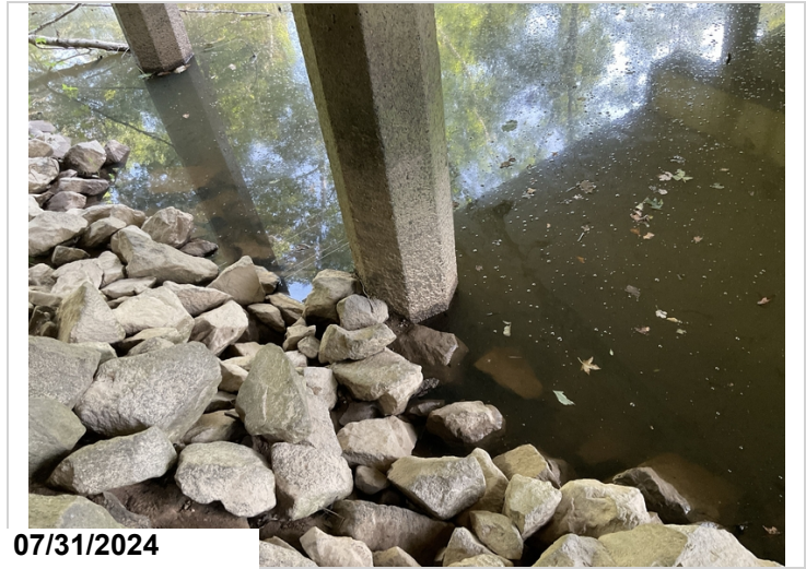
Bent 2 pile 2 minor abrasion at waterline. Common all piles this bent.
