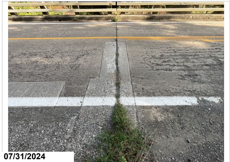
Bent 3 joint seal full of debris.
