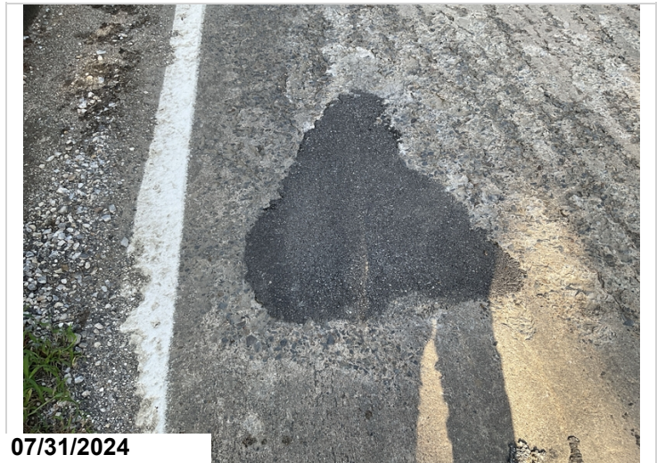
Span 3 spall filled with asphalt. 15'CS3
