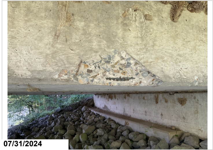
Span 1 left side spall with exposed rebar in side of deck. CS3 1'.
