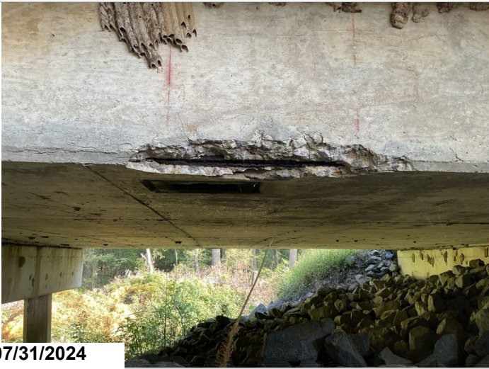
Span 3 right side spall with exposed rebar in side of deck. CS3 2'.
