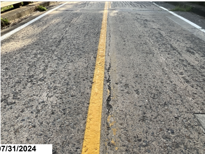
Span 2 longitudinal crack at centerline.
