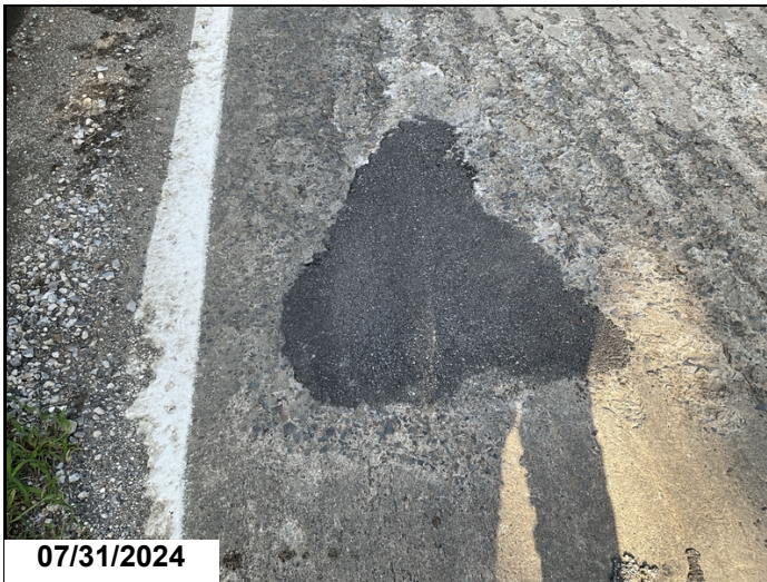
Span 3 spall filled with asphalt. 15'CS3
