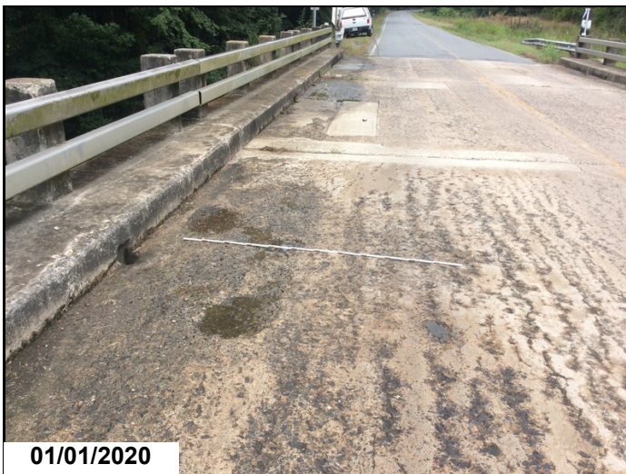
Span 3 spall filled with asphalt. 15'CS3
