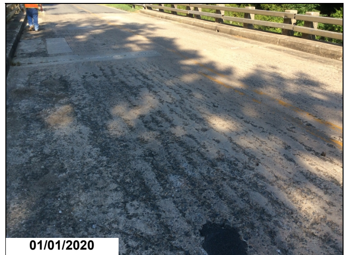
Overview of deck with heavy abrasion, cracks and patches.
