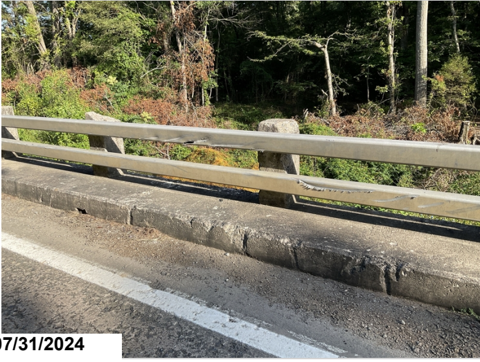
Span 3 left bridge rail damaged due to traffic impact.
