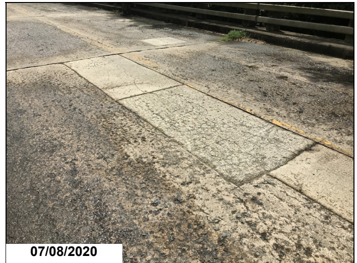
Deck has small spalls and heavy scaling.
