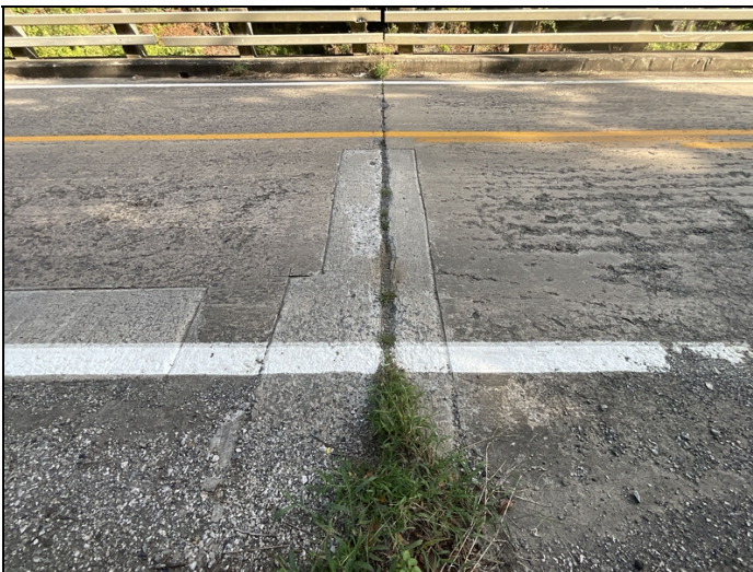
Bent 3 joint seal full of debris.
