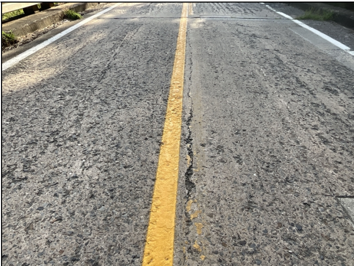
Span 2 longitudinal crack at centerline.
