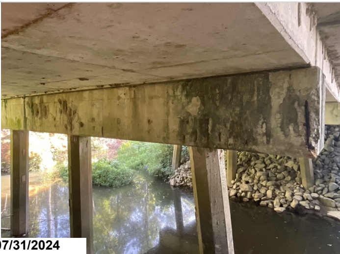
Bent 2 cap back spalls with exposed rebar. CS3 7'.
