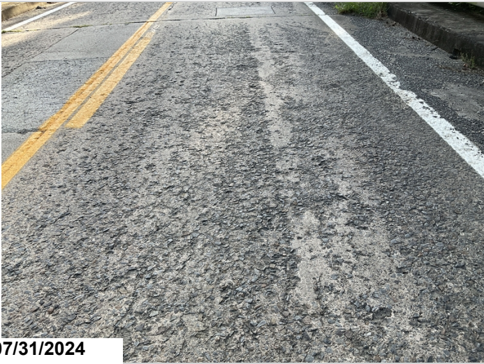
Span 1 abrasion in concrete deck.
