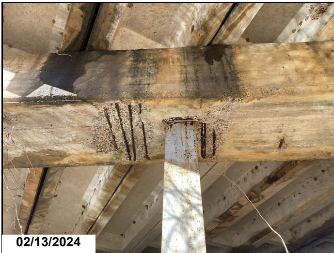
Bent 5 cap at pile 2 spall with exposed rebar at pile 2. 50% section loss to hoop bars.
