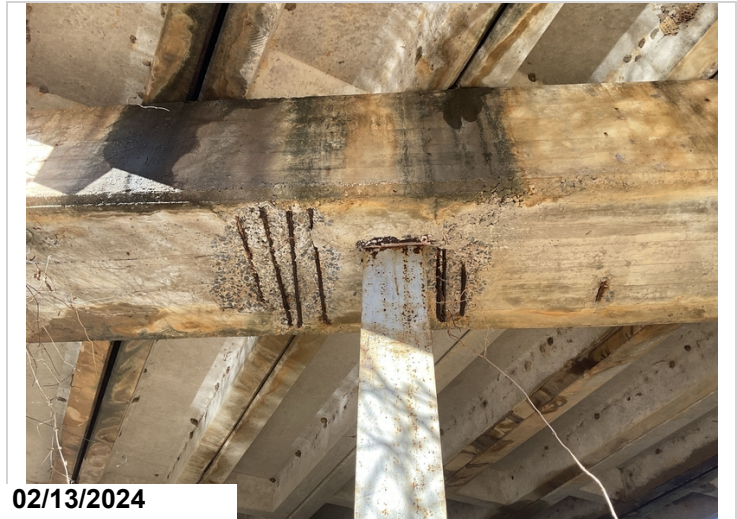
Bent 5 cap at pile 2 spall with exposed rebar at pile 2. 50% section loss to hoop bars.
