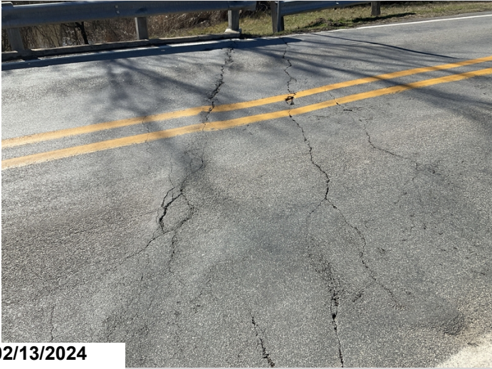
Bent 6 cracks in the asphalt wearing surface.
