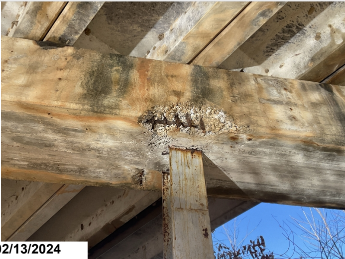
Bent 5 cap back above pile 4 spall with exposed rebar. 50% section loss on rebar.
