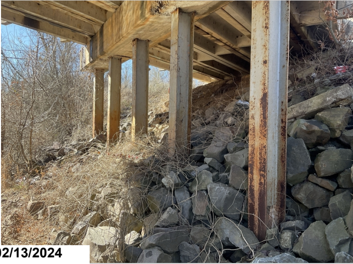
Bent 5 steel piles have active corrosion with minor pitting.
