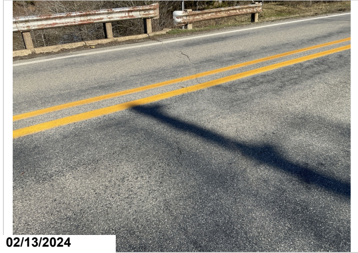
Bent 1 cracks in asphalt wearing surface.
