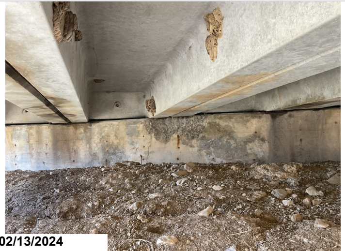
Bent 6 large spall under units 3 & 4.
