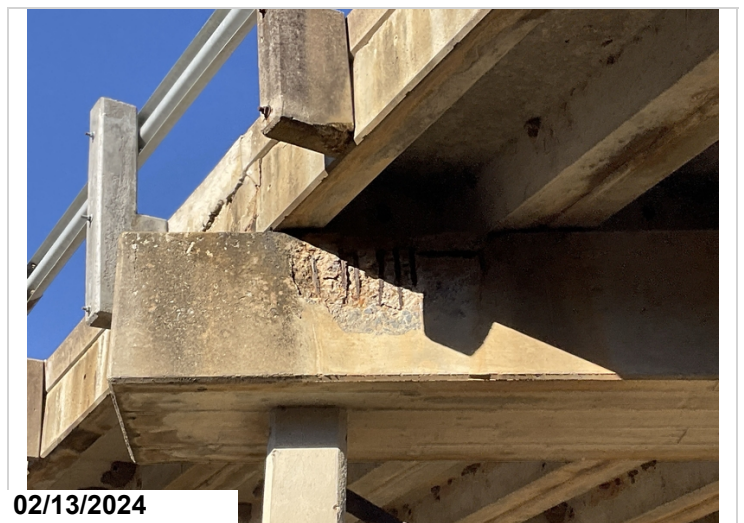
Bent 2 cap back right side spall with exposed rebar.
