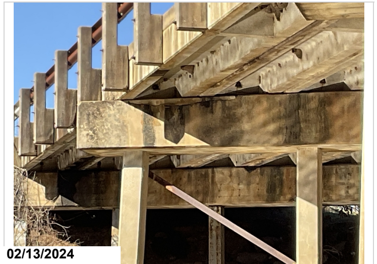
Bent 4 cap back above piles 1 & 2 large delam.
