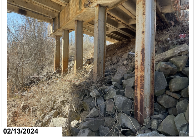
Bent 5 steel piles have active corrosion with minor pitting.
