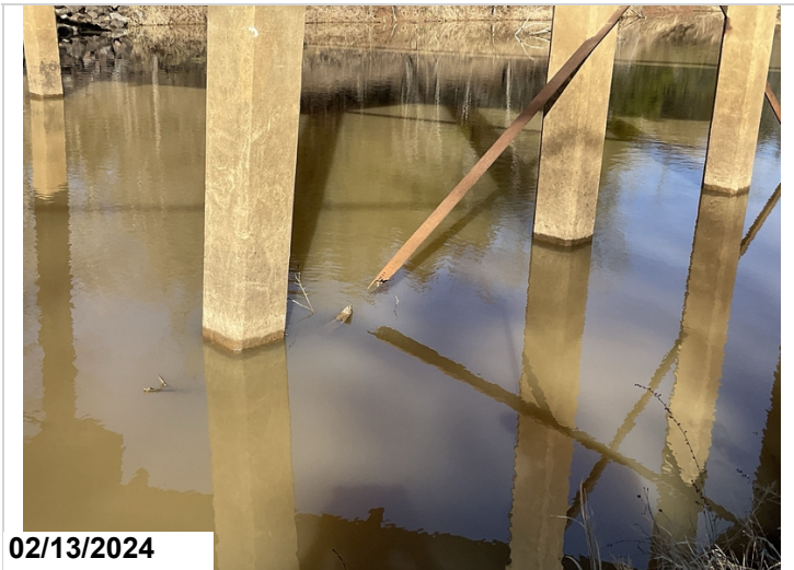
Bent 2 cross bracing section loss.
