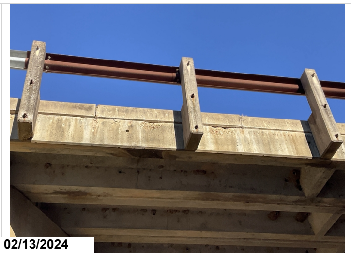
Span 1 girder 1 left side spalls.
