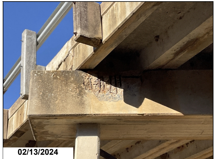
Bent 2 cap back right side spall with exposed rebar.
